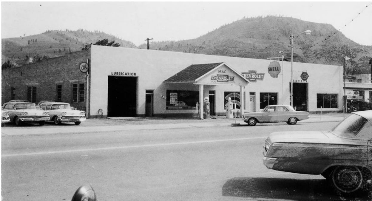
221 E. Woodin Avenue: View looking northeast on Woodin Avenue, showing the Shell Oil service station at the Mac Chevrolet dealership. Richfield service station is on far right. Photo date is 1962 or 1963. Source: Chelan Museum collection.
