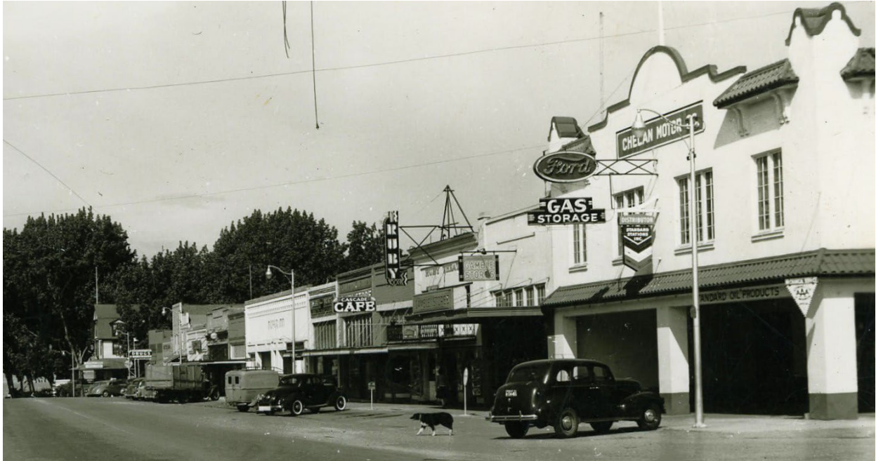
141 E. Woodin Avenue: View looking west on Woodin Avenue. On the right is the Chelan Motor Company's garage and Ford dealership, after removal of the gasoline pump from the street margin. The hanging sign reads "Distributor, Standard Stations Inc." Photo date is late 1940s. Source: online photo (John Boyd Ellis photo).
