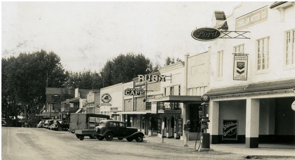
141 & 125 E. Woodin Avenue: View looking west on Woodin Avenue. On the right is the Chelan Motor Company's garage (141 E. Woodin), with a Standard Oil gasoline pump next to the sidewalk. The Motor Inn garage (125 E. Woodin) is the white building left of the Cafe sign, with a Gilmore Red Lion gasoline sign. Photo date is circa 1939. Source: Chelan Museum collection (John Boyd Ellis photo).
