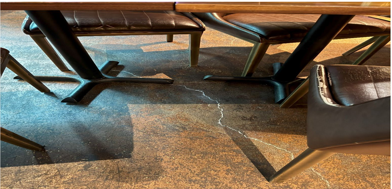
Photograph 2. The previously identified crack sealed with compatible epoxy/caulking in good shape at the 13 Coins Restaurant on the King Street property.
