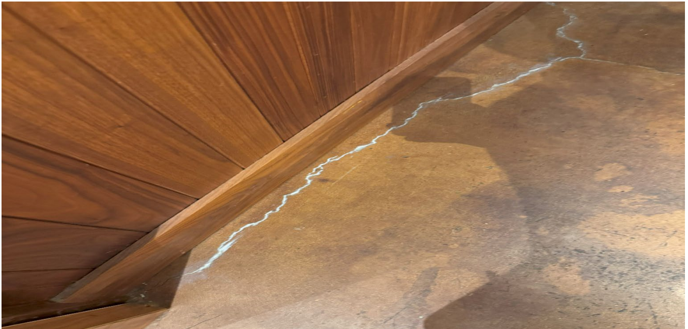
Photograph 1. The previously identified crack sealed with compatible epoxy/caulking in good shape at the 13 Coins Restaurant on the King Street property.
