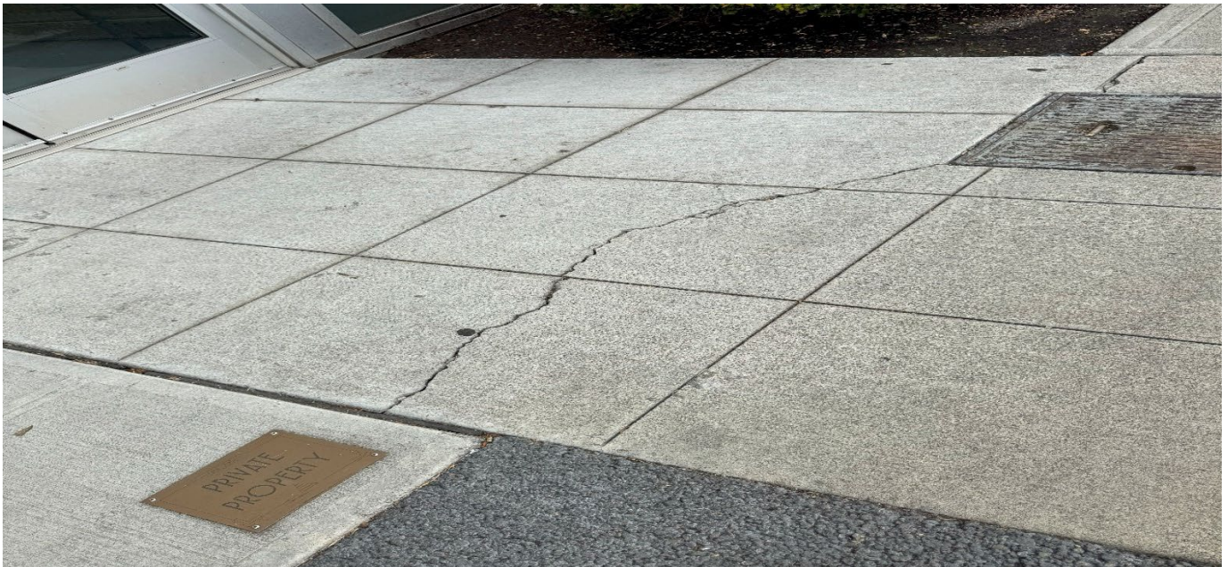
Photograph 4. Previously identified cracking on the southern exterior walkway of the building, immediately adjacent to the southeast corner of the building and at the edge of the property. Repairs are recommended at this time.
