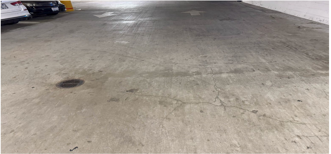
Photograph 3. Non-structural hairline cracking in the underground parking garage. The amount of cracking does not appear to have increased since the 2024 inspection. Repairs are not needed at this time.
