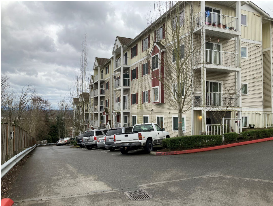
Photo 2: Driveway along north end of Property from north entrance
