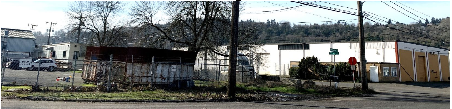
South Park Landfill Cleanup Site from S. Kenyon Street
