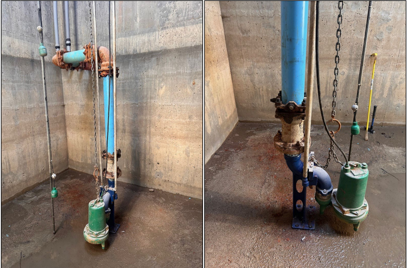
New West Vault Sump Pump Installation
