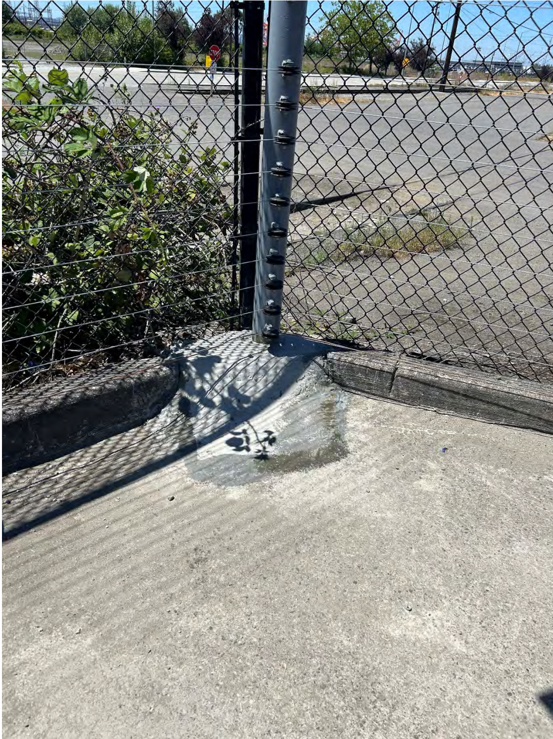
Typical corner post foundation raised to divert water away from post. Post to foundation and foundation to surrounding pavement have been sealed with epoxy to prevent water intrusion at the joint, typical.
