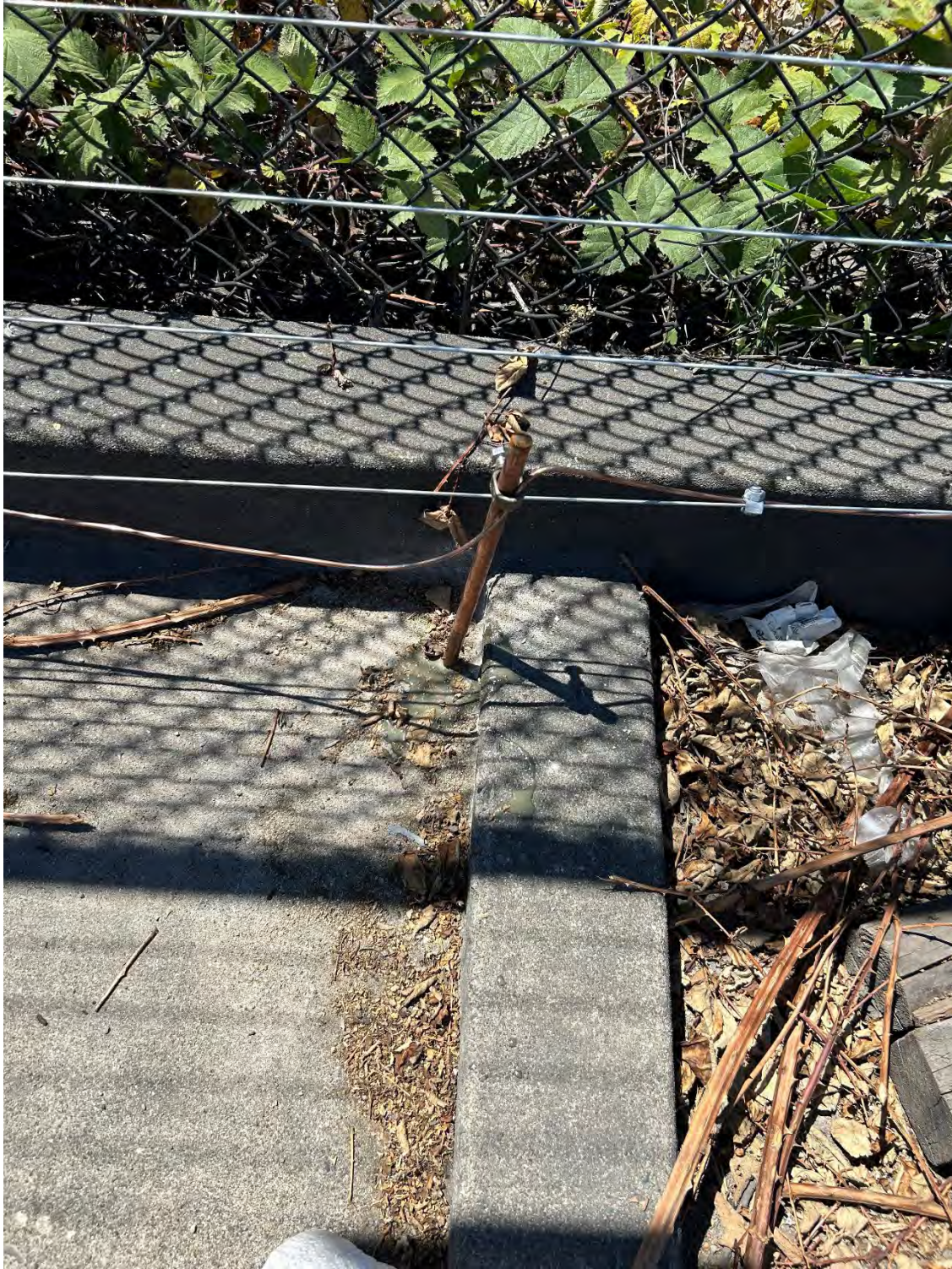
Ground rod installation is similar to intermediate posts shown on previous picture.
