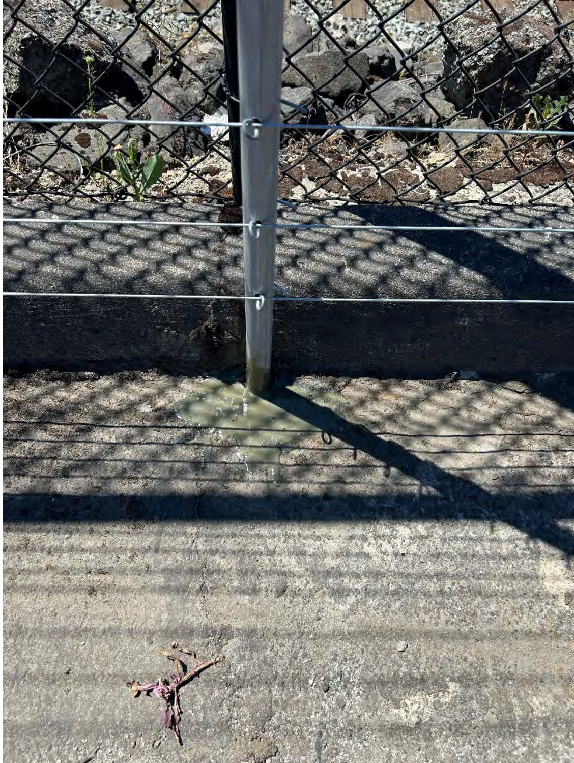
Intermediate posts were core drilled into the concrete cap. Following grouting in place the entire area was flooded with epoxy to prevent water intrusion.
