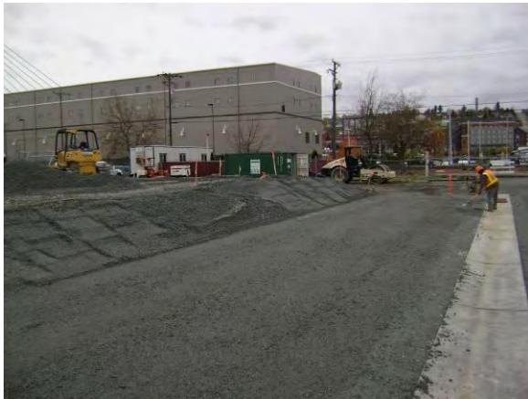
Photo 74B: Site grading– Phoenix lay down yard reconstruction looking southwest.
