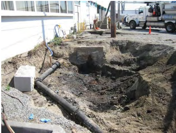
Photo 7B: Safe Dig Area excavation – west side looking east.
