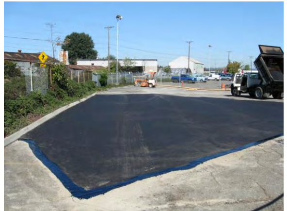
Photo 10D: Asphalt pavement complete, south end of excavation area looking north.
