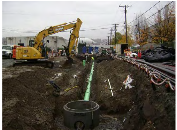
Photo 30C: Utility reconstruction – sanitary sewer alignment looking south.
