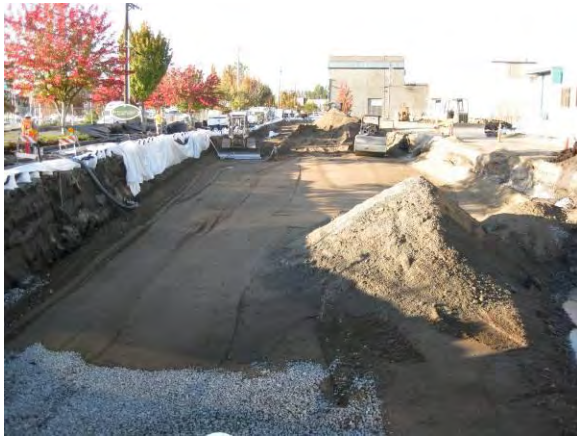
Photo 44C: Excavation backfilling – southwest quarter of excavation area looking north.
