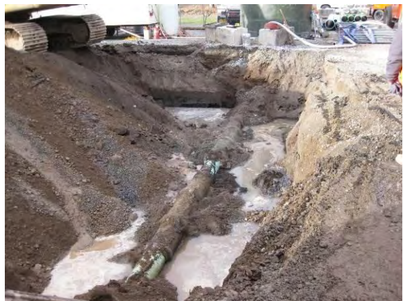
Photo 43B: Excavation area southwest of Area B along sanitary sewer alignment.
