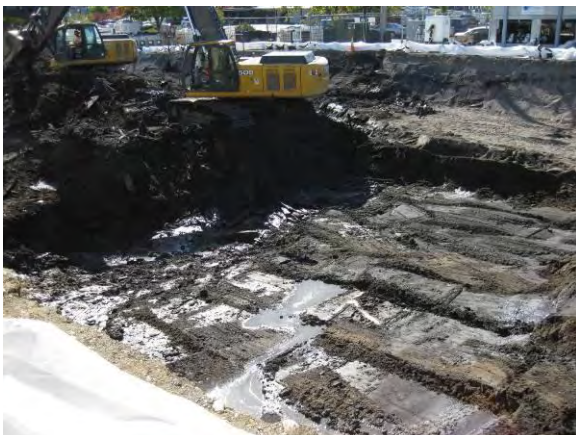
Photo 21C: Excavation – north half of excavation area looking southwest.
