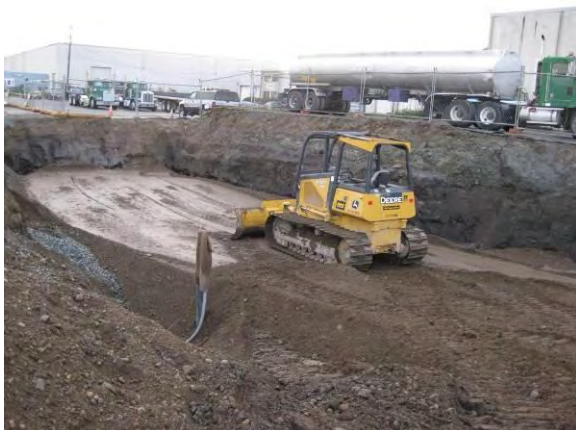
Photo 64B: Excavation backfilling – northwest corner of Phoenix excavation looking southeast.
