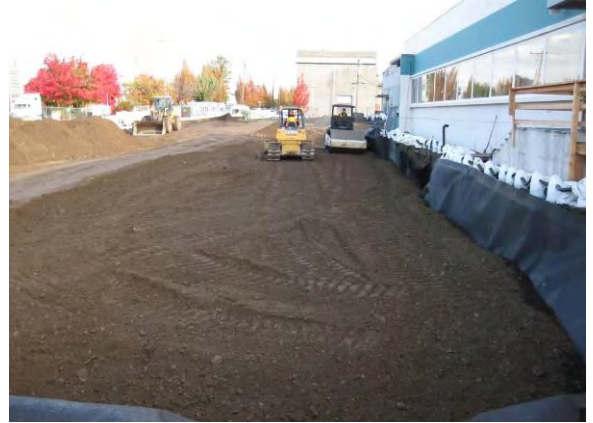
Photo 51C: Excavation backfilling – southeast quarter of excavation area looking north.
