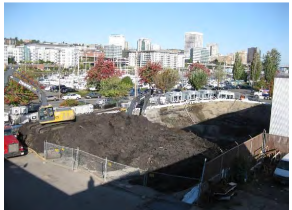
Photo 22C: Excavation – north half of excavation area looking northwest.
