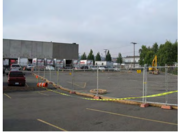
Photo 2D: Pre remediation – north end of excavation area looking southwest.
