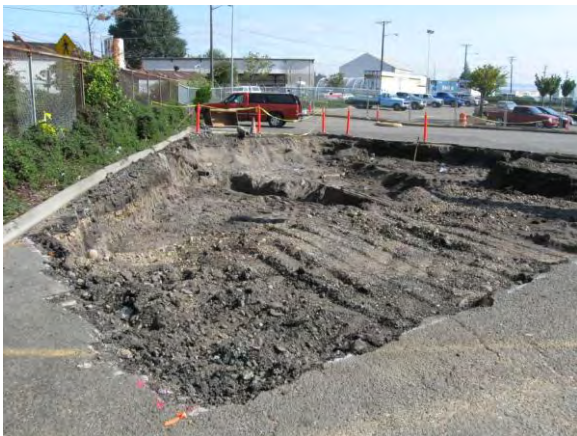
Photo 3D: Excavation – south end of excavation area looking north.
