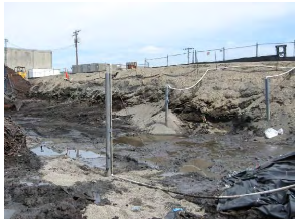
Photo 12A: Excavation dewatering – south end of excavation area looking northeast.
