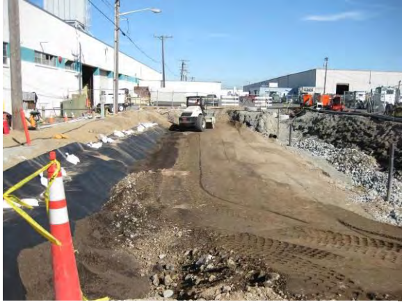
Photo 60B: HDPE liner – darker high TOC material placed against liner looking east.
