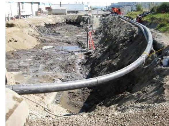
Photo 20B: Excavation area southwest corner looking east along sewer bypass lines.
