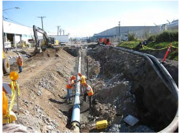
Photo 47B: Utility reconstruction – East 19th Street storm sewer alignment.
