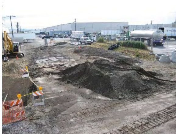
Photo 14B: Excavation area – northwest corner looking southeast.
