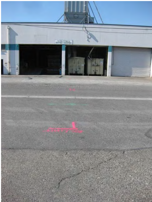
Photo 3B: Pre remediation – southeast corner looking north.
