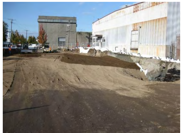
Photo 43C: Excavation backfilling – north half of excavation area looking north.
