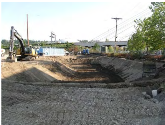
Photo 19A: Pond rebuilding – looking south over north pond.
