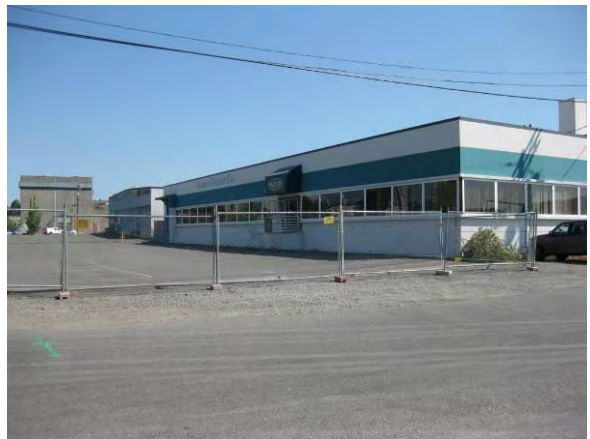
Photo 5C: Pre remediation – Tacoma Fixtures building southwest corner of excavation area looking northeast.
