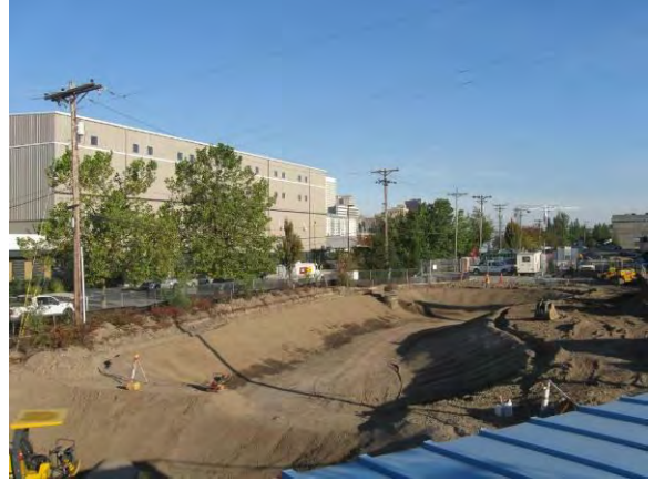
Photo 26A: Pond rebuilding – southeast corner of excavation area looking northwest.
