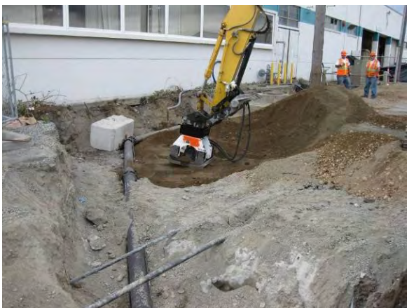
Photo 57B: Excavation backfilling – west end of Safe Dig Area looking northeast.
