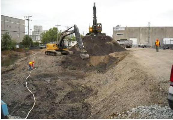
Photo 7A: Excavation – overburden removal, south end of excavation area looking north.
