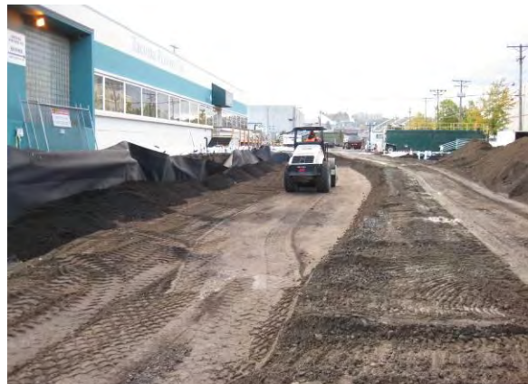
Photo 47C: Excavation backfill – high TOC fill next to HDPE liner looking south.
