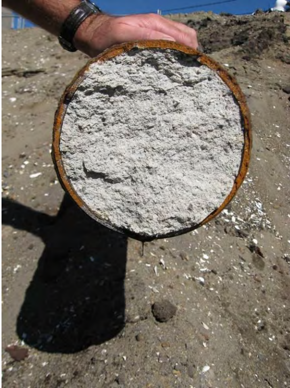
Photo 39C: BNSF Oil Pipeline – grouted at north end of excavation area.
