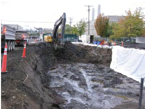
Photo 25C: Excavation – southwest quarter of excavation area looking south.
