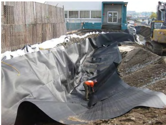
Photo 46C: HDPE liner – north end of liner looking south.
