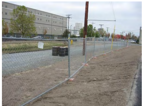
Photo 30A: Post remediation – east side of excavation area looking northwest.
