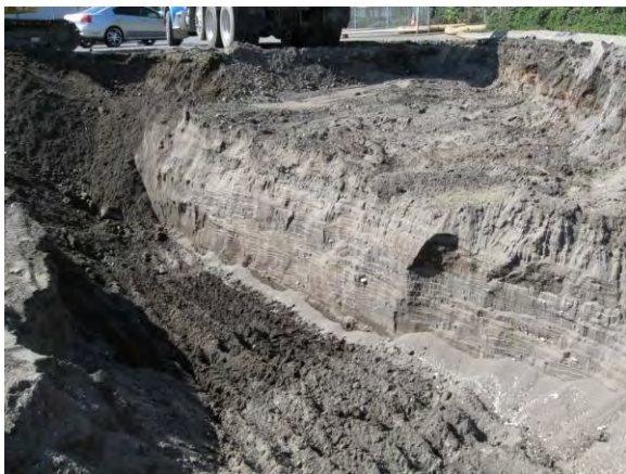
Photo 5D: Excavation – trench along oil pipeline alignment looking southwest.
