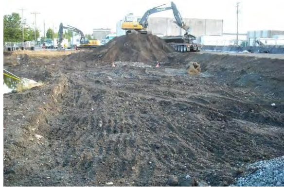
Photo 8A: Excavation – overburden removal, southwest corner of excavation area looking northeast.
