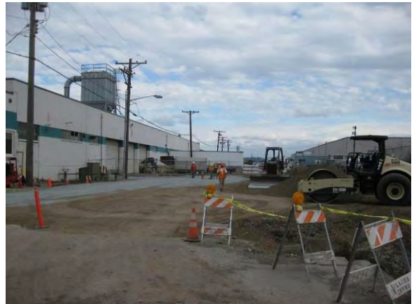
Photo 69B: Site grading – west end of excavation looking east.
