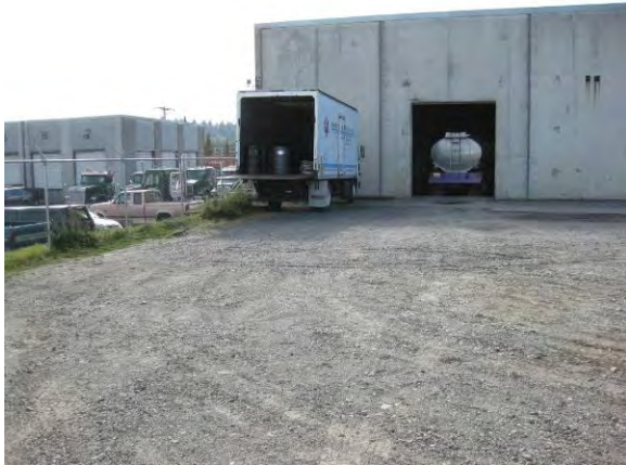
Photo 5B: Pre remediation – north side of Phoenix lay down yard looking southeast.
