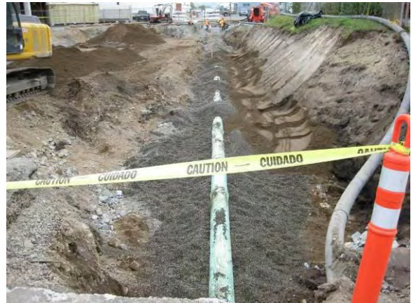
Photo 49B: Utility reconstruction – sanitary sewer main alignment looking east.
