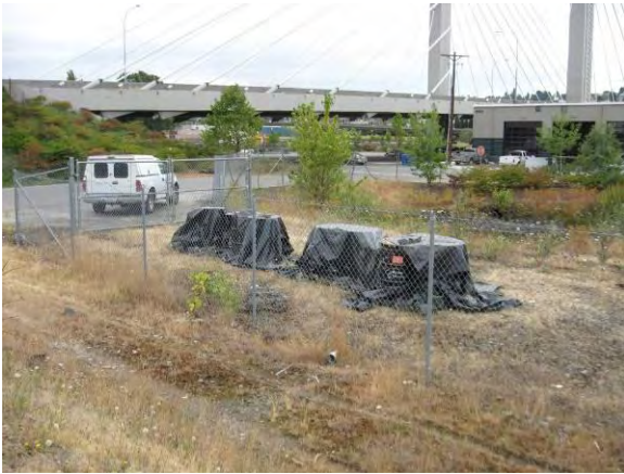
Photo 1A: Pre remediation – east side of excavation area looking southwest.
