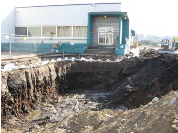
Photo 10C: Soil freeze wall – northwest corner of Tacoma Fixtures looking south.
