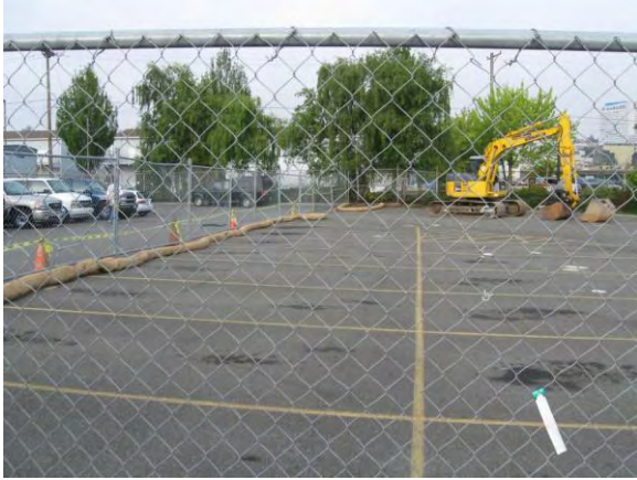
Photo 1D: Pre remediation – southeast corner of excavation area looking northwest.
