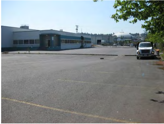
Photo 1C: Pre remediation – northwest corner of excavation area looking southeast.
