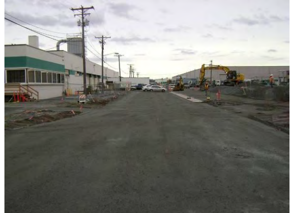
Photo 73B: Site grading – gravel subgrade for East 19 th Street looking east.
