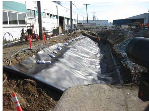
Photo 59B: HDPE liner – north sidewall looking east.
