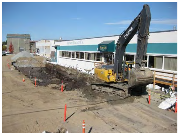
Photo 28C: Excavation – southeast quarter in front of Tacoma Fixtures building looking northeast.
