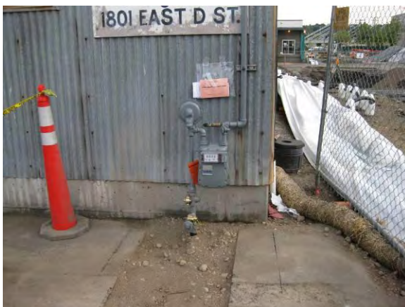
Photo 33C: Utility reconstruction – new natural gas meter for SuperValu building.
