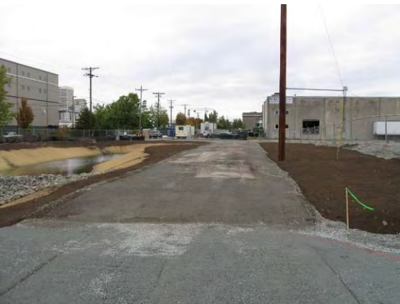
Photo 29A: Post remediation – WSDOT pond maintenance road looking north.
