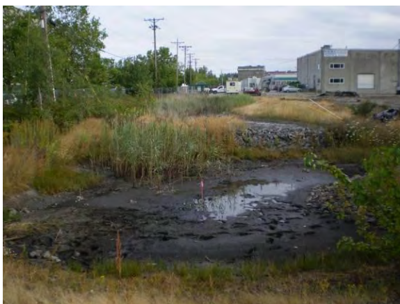
Photo 5A: Pre remediation – south side of WSDOT ponds looking north.
