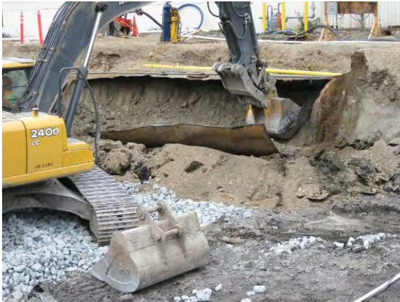
Photo 29B: East 19 th Street UST - removing CDF from UST.
