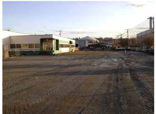
Photo 53C: Site grading – south half of excavation area looking south.
