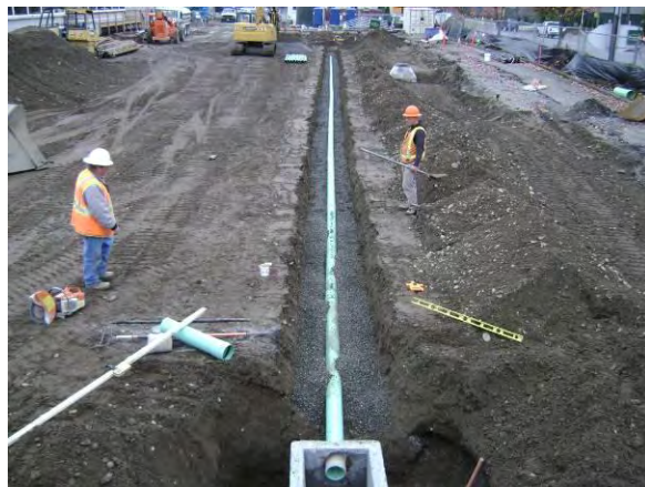
Photo 37C: Utility reconstruction – storm sewer lateral alignment looking south.
