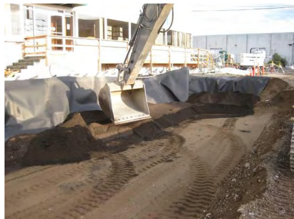
Photo 49C: High TOC fill – southeast quarter of excavation area looking southeast.
