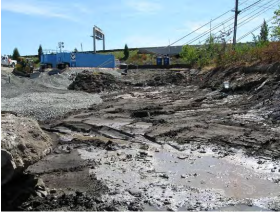
Photo 13A: Excavation – base under WSDOT ponds, looking south.
