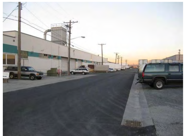
Photo 77B: Post remediation – East 19 th Street new asphalt pavement looking northeast.
