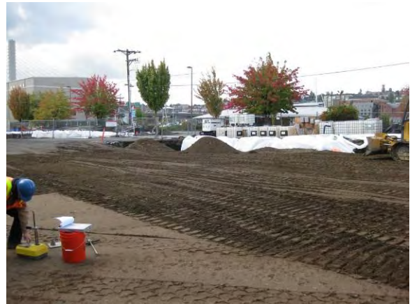
Photo 45C: Excavation backfilling – compaction testing within of excavation area.
