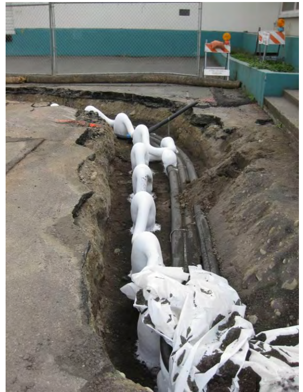
Photo 9C: Soil freeze wall – freeze pipe manifolding with ice buildup.
