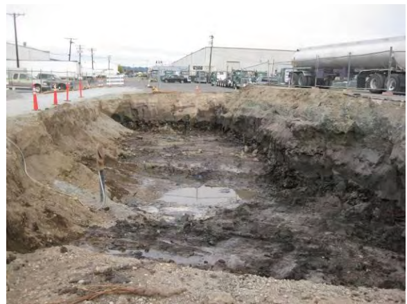
Photo 37B: Phoenix area excavation – west end of excavation looking east.
