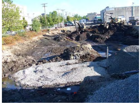
Photo 14A: Excavation – south end of excavation area looking north.
