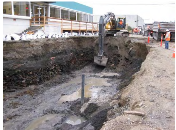
Photo 26C: Excavation – southeast quarter of excavation area looking southeast.
