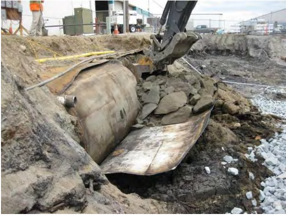
Photo 27B: East 19 th Street UST - removing CDF from UST.
