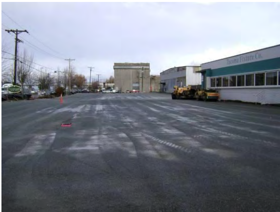
Photo 52C: Site grading – south end of excavation area looking north.
