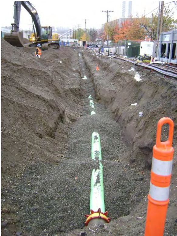
Photo 35C: Utility reconstruction – north end of the sanitary sewer alignment looking south.
