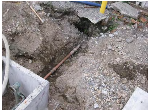
Photo 53B: Utility reconstruction – water service for Tacoma Fixtures.
