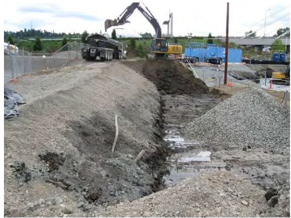
Photo 18A: Excavation – removing material to eastern limit looking south.
