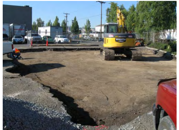
Photo 8D: Backfilling – north end of excavation area looking southwest.
