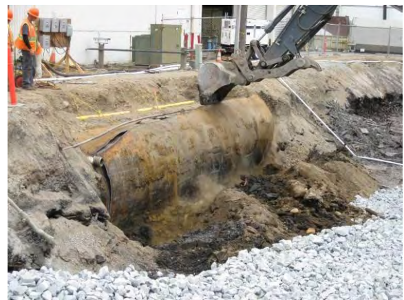
Photo 26B: East 19 th Street UST - cutting of UST has been completed, opening UST to access CDF.
