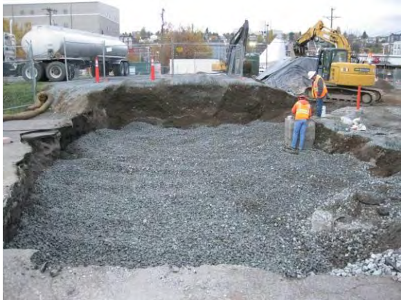
Photo 66B: Excavation backfilling – east end of Nichols excavation looking west.
