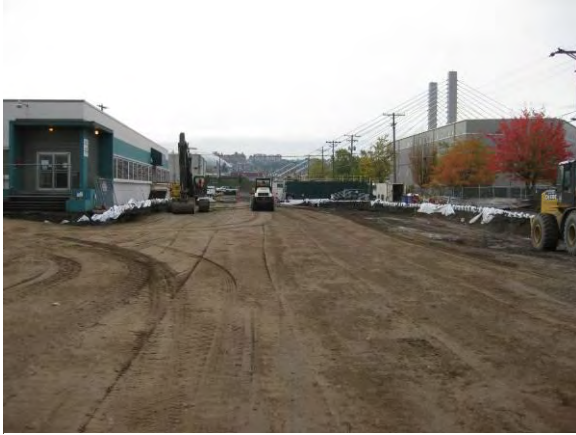
Photo 50C: Excavation backfilling – south half of excavation area looking south.
