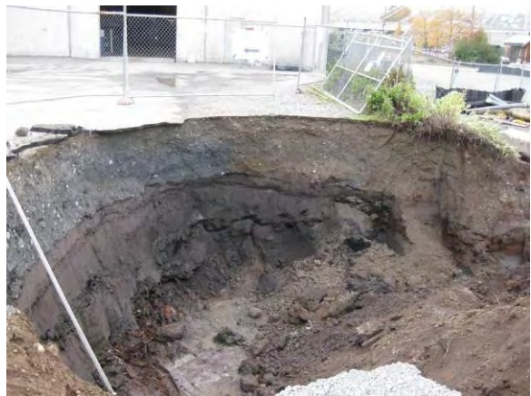
Photo 41B: Phoenix/Nichols area excavation – looking south along west side of Phoenix lay down yard.
