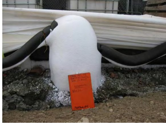
Photo 12C: Soil freeze wall – ice buildup on freeze pipe head.
