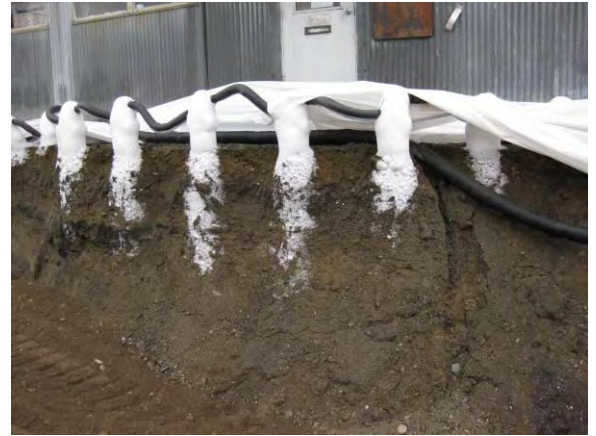
Photo 7C: Soil freeze wall – east sidewall adjacent to the SuperValu west entrance.
