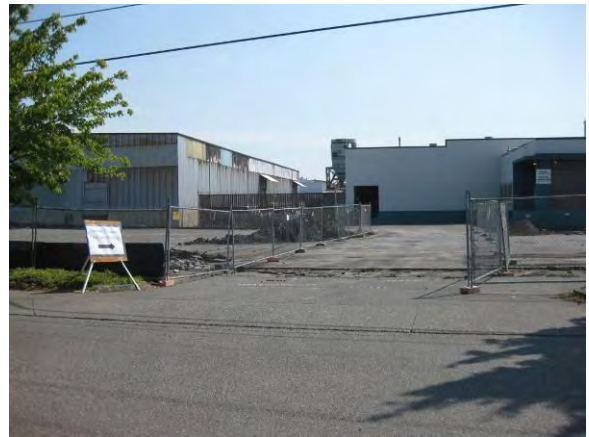
Photo 4C: Pre remediation – D Street entrance of excavation area looking east.
