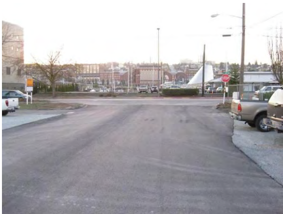
Photo 76B: Post remediation – East 19 th Street new asphalt pavement looking west.
