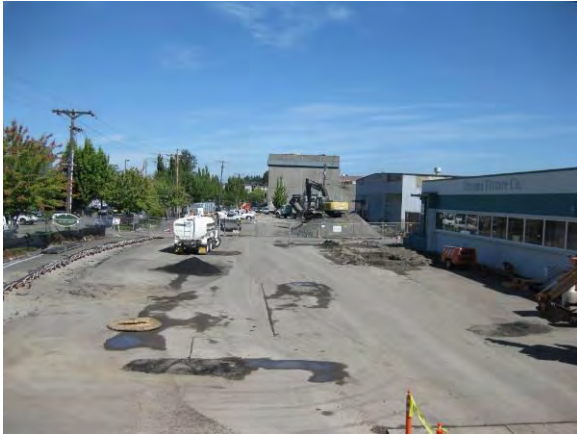
Photo 13C: Excavation area south end looking north.
