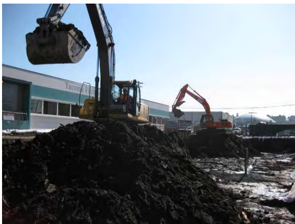
Photo 27C: Excavation – northwest corner of southwest quarter of excavation area looking southeast.
