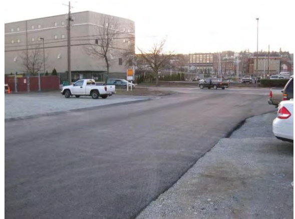
Photo 75B: Post remediation – East 19 th Street new asphalt pavement looking southwest.
