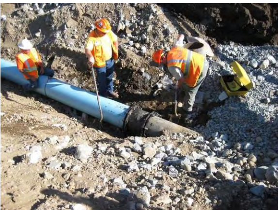
Photo 48B: Utility reconstruction – East 19th Street storm sewer west connection.
