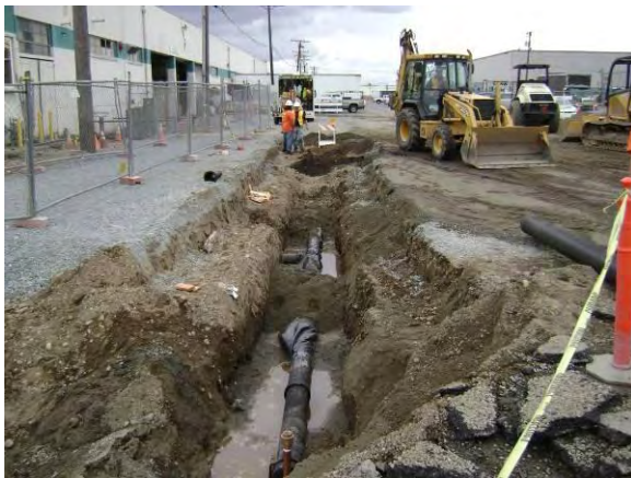
Photo 52B: Utility reconstruction – East 19 th Street water main looking east.
