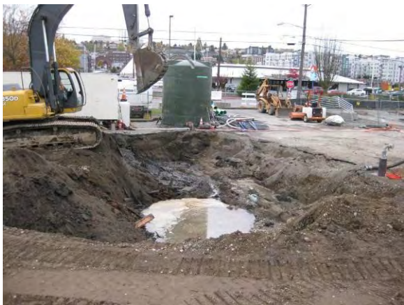
Photo 42B: Excavation area southwest of Area B looking west.
