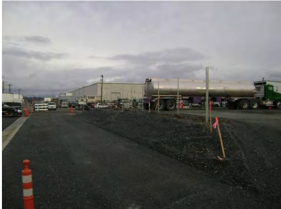
Photo 72B: Site grading – Phoenix lay down yard reconstruction looking southeast.
