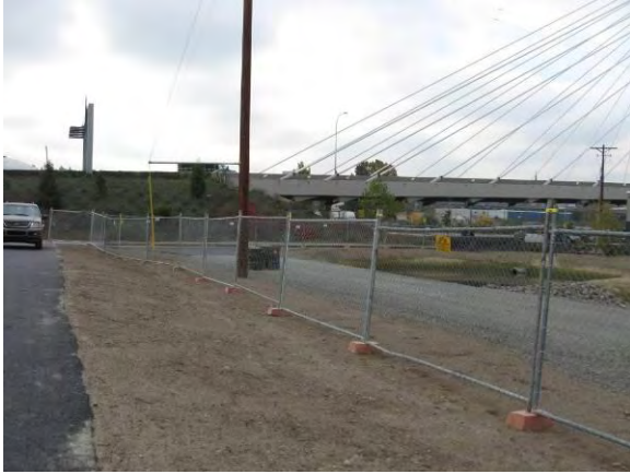
Photo 31A: Post remediation – east side of excavation area looking southwest.
