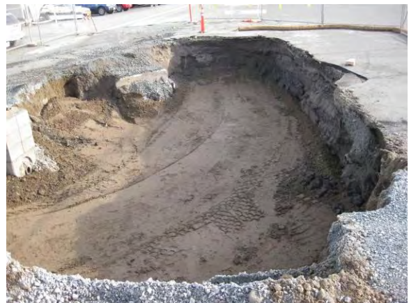
Photo 65B: Excavation backfilling – west end of Nichols excavation looking east.
