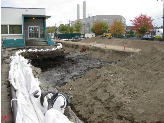
Photo 11C: Soil freeze wall – looking southwest, displaying east sidewall curvature.
