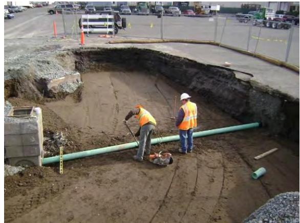
Photo 51B: Utility reconstruction – storm sewer lateral crossing Nichols excavation area.
