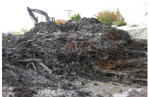
Photo 18C: Excavation – wood waste from north half of excavation area looking southwest.
