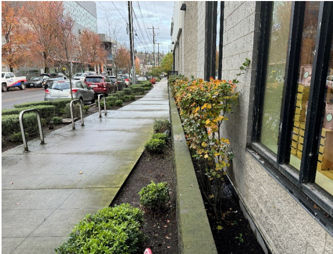
Photograph 3. Easterly-facing view of the Area B cap (right of the sidewalk) along the northern side of the Site.
