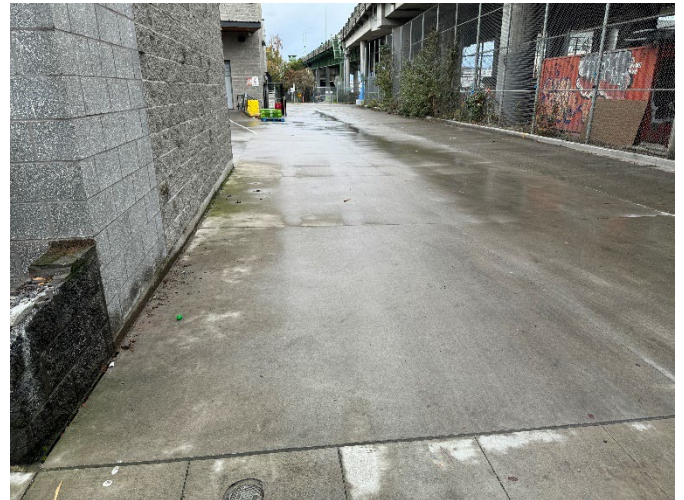
Photograph 2. Southerly-facing view of the Area B cap along the western side of the Site.
