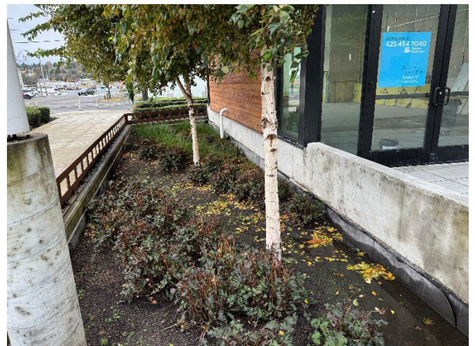
Photograph 6. Southerly-facing view over the Area B Cap along the eastern side of the Site.
