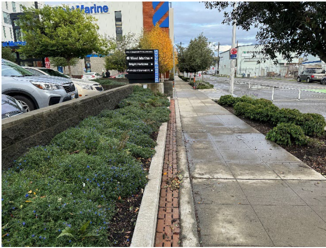
Photograph 1. Easterly-facing view of the Area B cap (left of the sidewalk) along the southern side of the Site.
