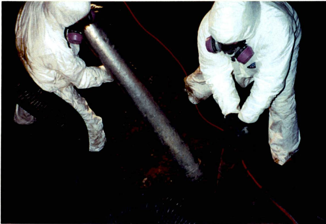
Photograph 3 – Excavation of impacted soil using vector truck.
