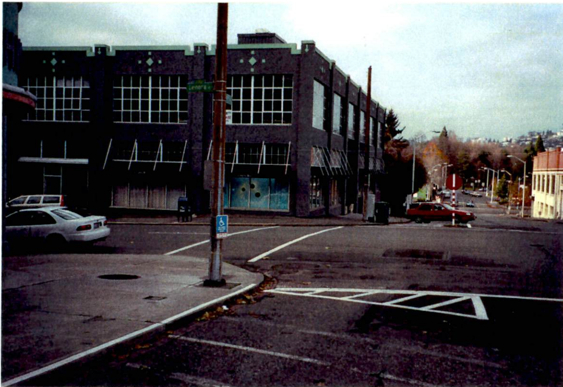
Photograph 2 – The Lenora Building (looking northerly).
