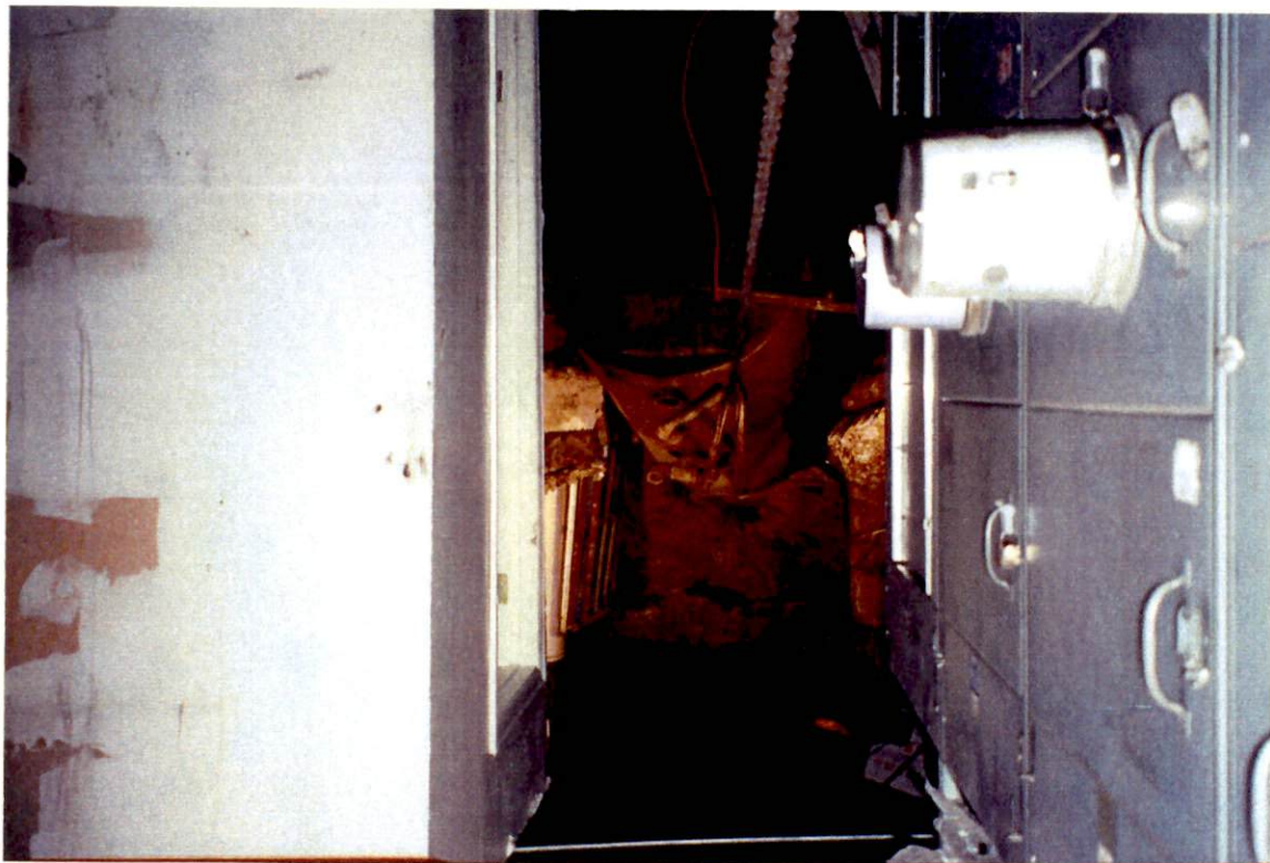
Photograph 8 – Lifting up UST1 (Note the tight clearance).
