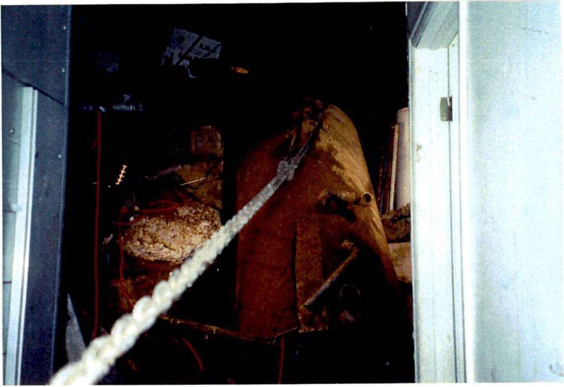
Photograph 9 (above) – Lifting up UST1 (Note the tight clearance).
