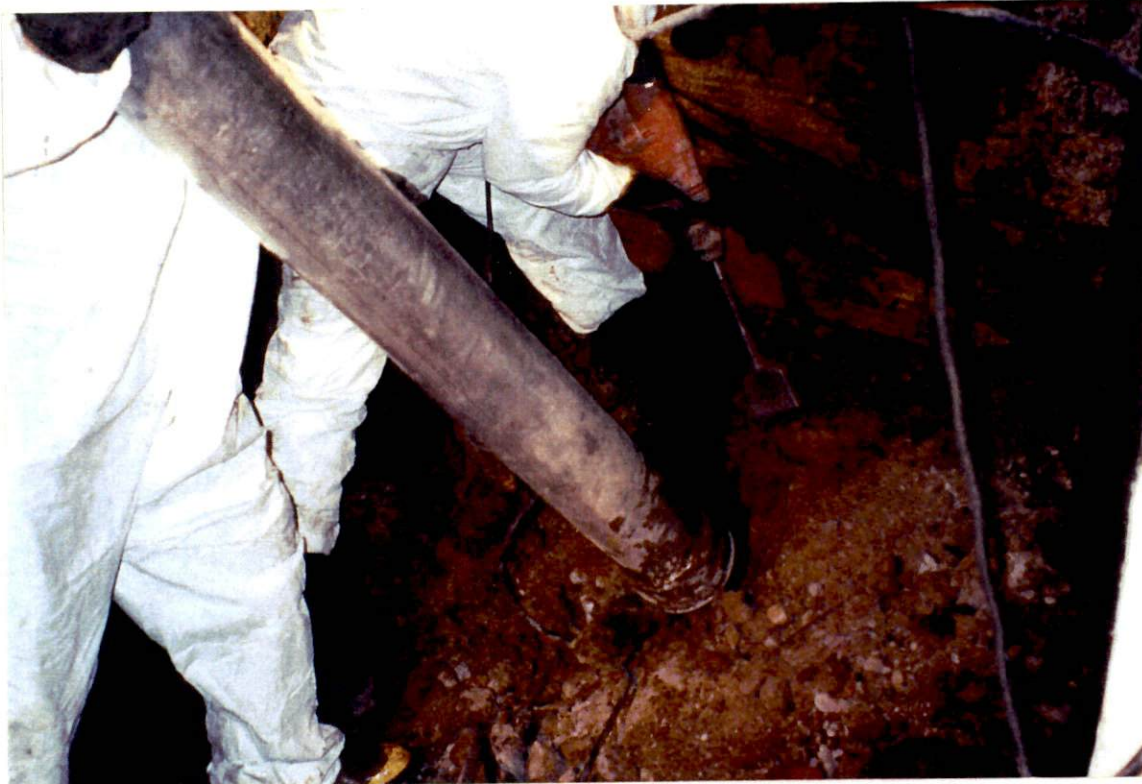
Photograph 5 (Above) – Excavation of impacted soil using vector truck.
