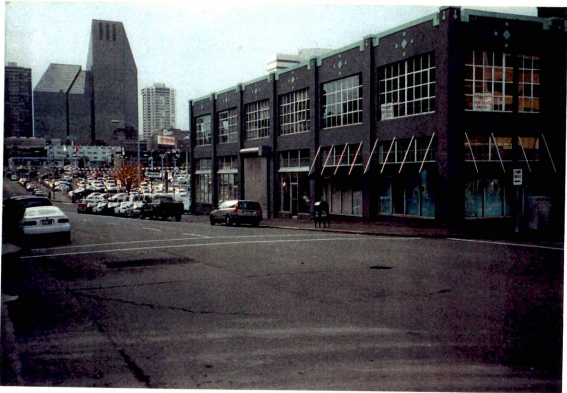
Photograph 1 – The Lenora Building (looking northwesterly).
