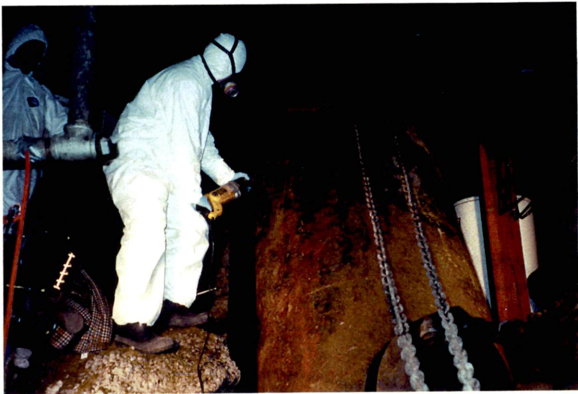
Photograph 12 – Cutting up UST1 into manageable pieces.
