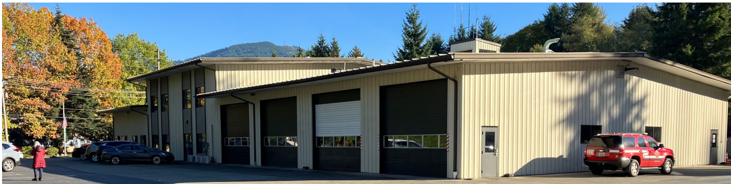
Eastside Fire & Rescue Headquarters 地块，属于 Eastside Fire & Rescue Headquarters and Issaquah Valley Elementary School (EFR HQ IVES) 清理场地
