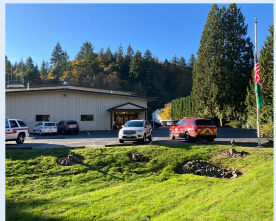
Eastside Fire & Rescue Headquarters 地块，属于 Eastside Fire & Rescue Headquarters and Issaquah Valley Elementary School (EFR HQ IVES) 清理场地
