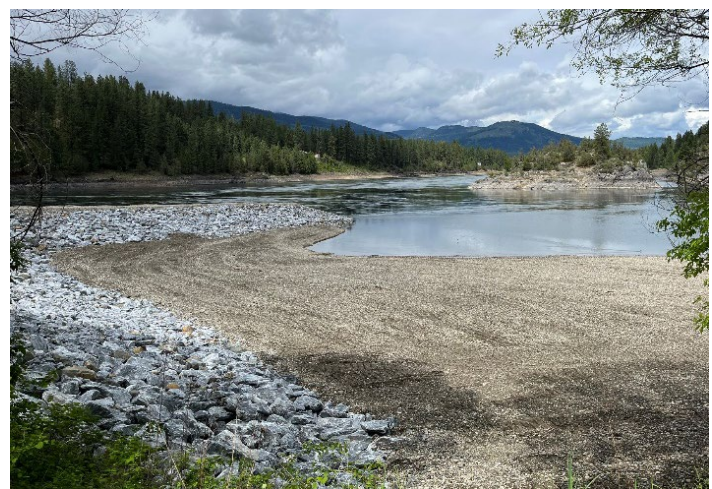
Jetty and bay area with clean caps. Two red maple trees will be planted on the jetty in fall 2025.
