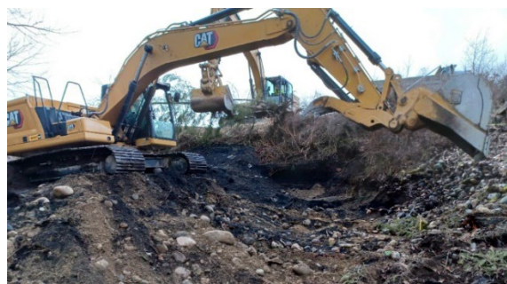
Black slag-contaminated soil being excavated from the hillside in 2024.
