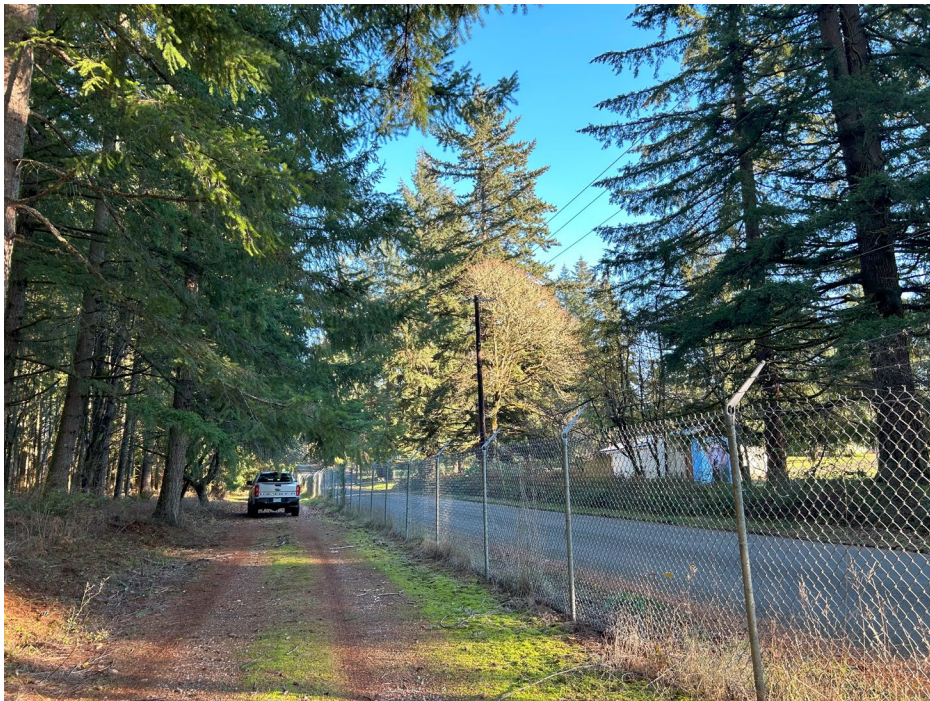
26. Perimeter fence at southern boundary of site. Signage is readily visible and at appropriately spaced intervals.
