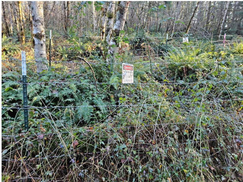
Photo 4. Five strand barbed wire at CITA expansion
