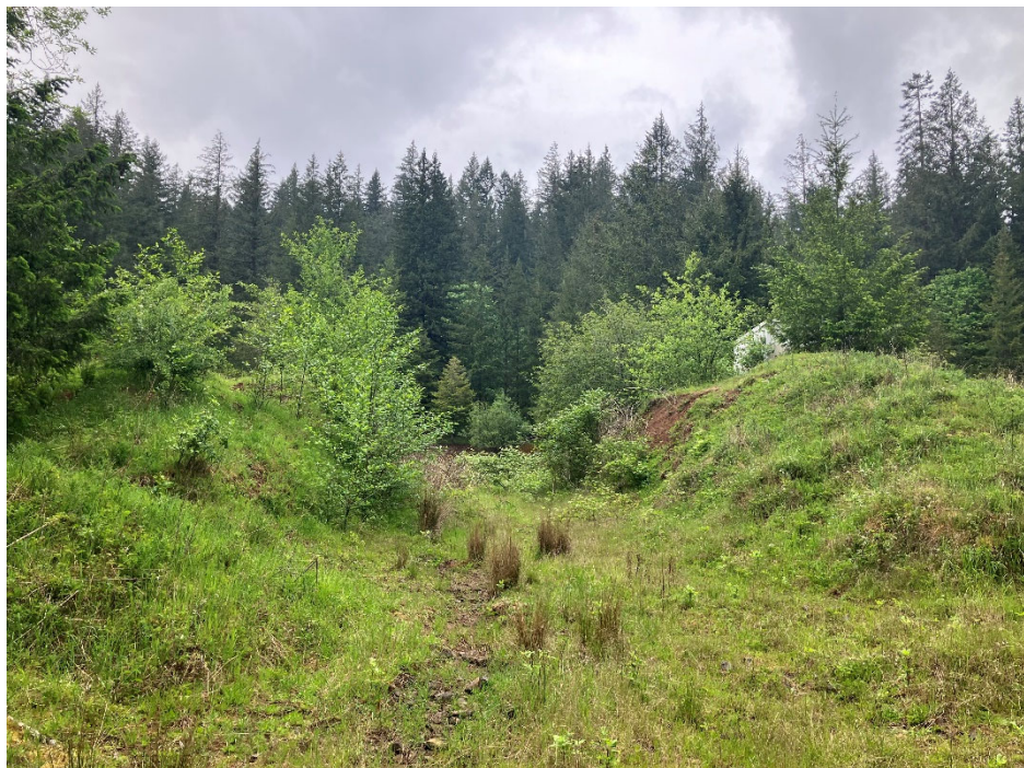
16. Sewage Lagoon – Facing north at entrance to west lagoon. Former operation house present on berm between lagoons.
