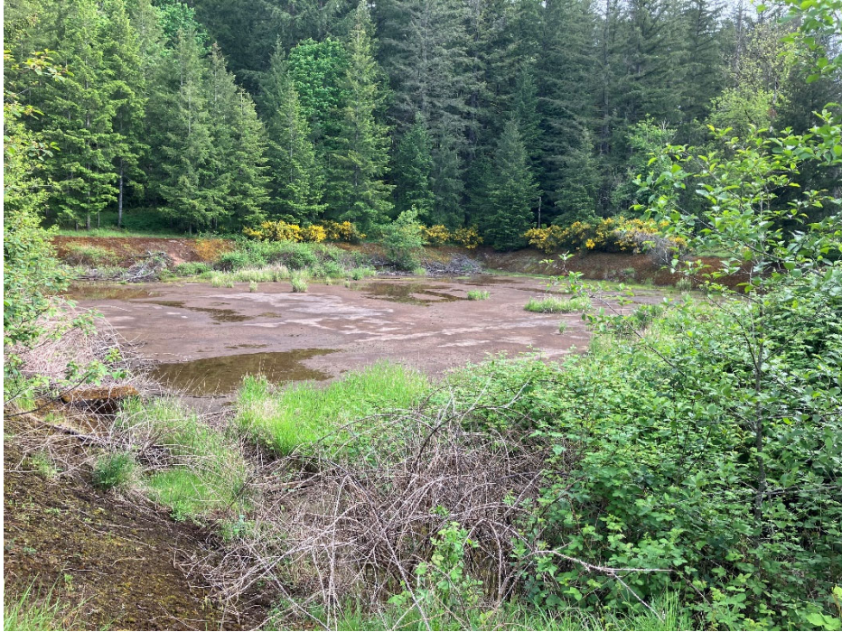
18. Sewage Lagoon (East) – Facing Northeast.
