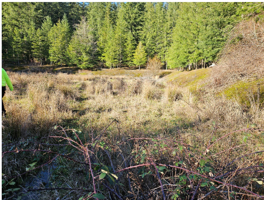
Photo 25. Breach in lagoon
