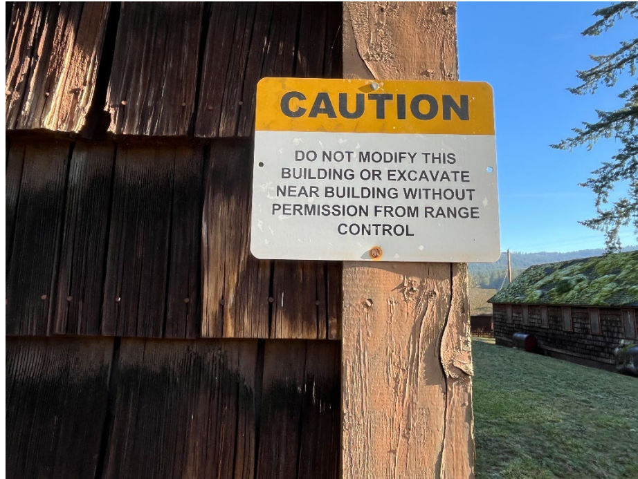
Photo 15. Building T-1932 AST signage
