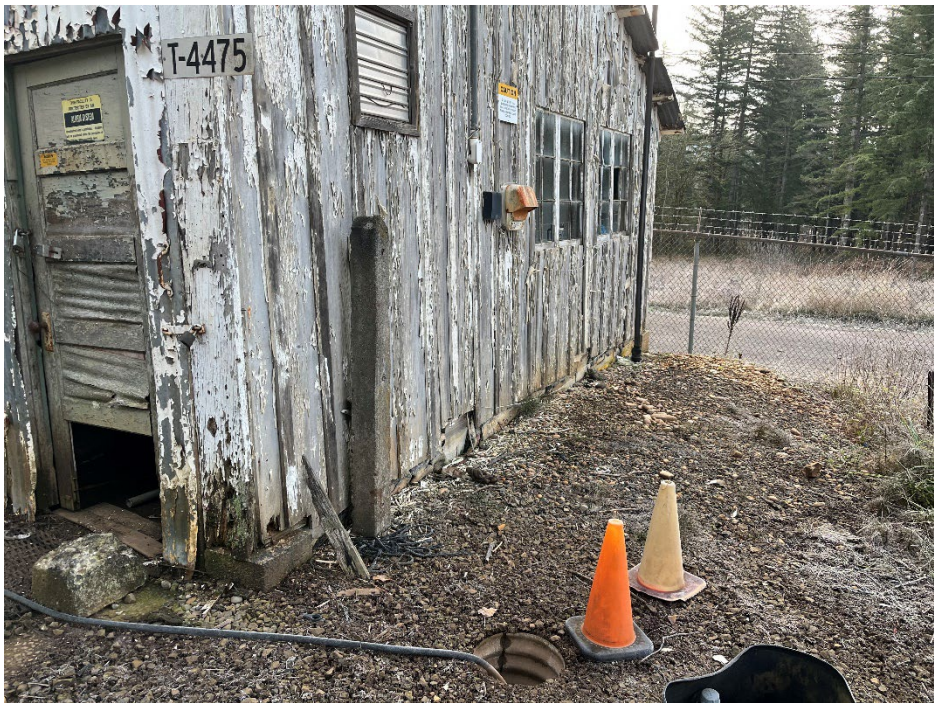
30. Bldg. 4475. Appropriate signage present on 4 sides of the building.
