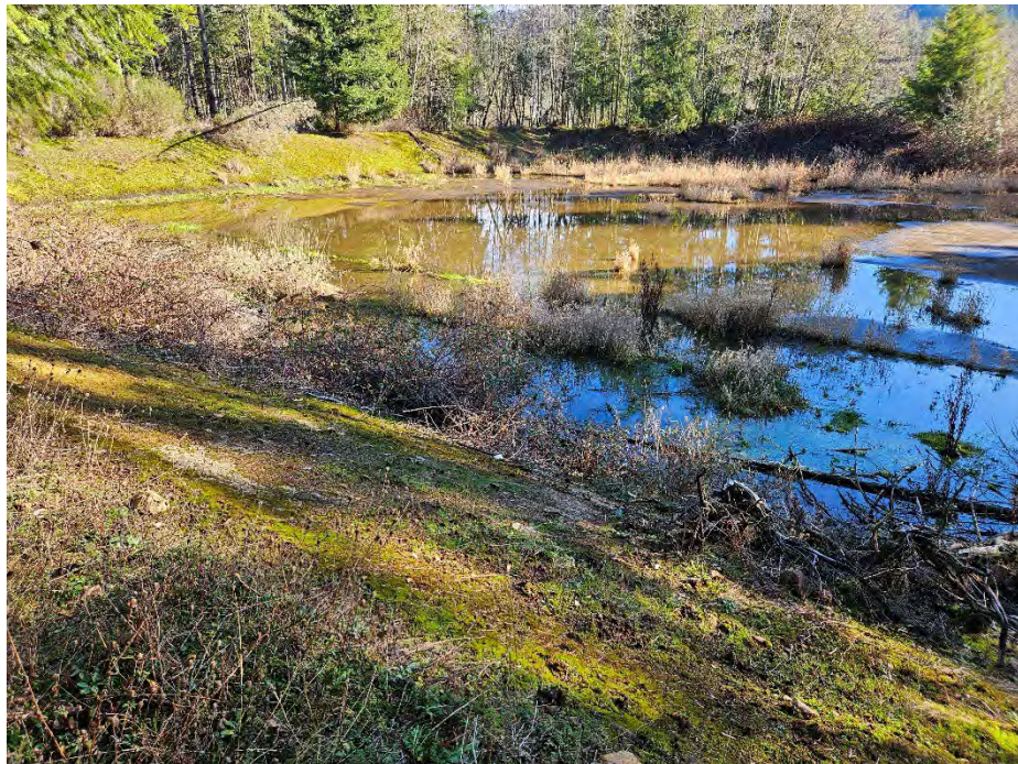
Photo 22. Eastern sewage lagoon view, facing southeast.
