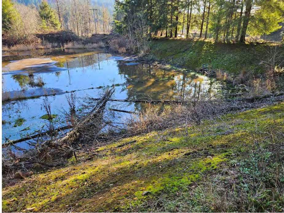
Photo 23. Eastern sewage lagoon view, facing southwest.
