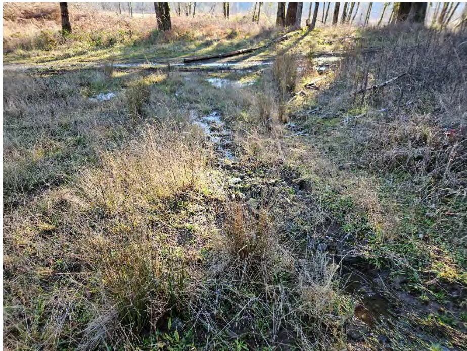
Photo 28. Drainage from the lagoon breach reaches the access road.
