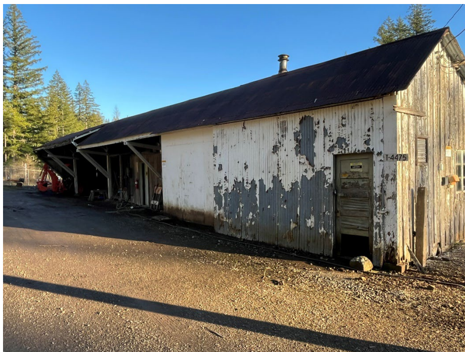
Photo 10. Building 4475 maintenance pit area signage
