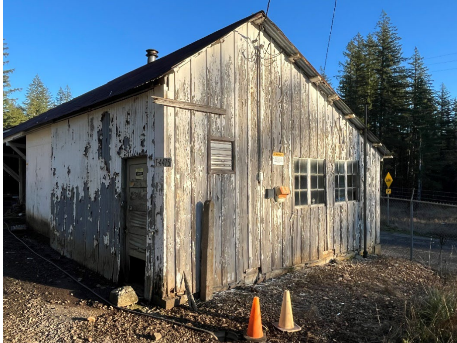
Photo 11. Building 4475 maintenance pit area signage
