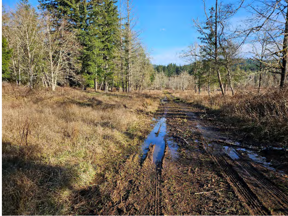
Photo 29. Drainage from the lagoon breach reaches the access road.
