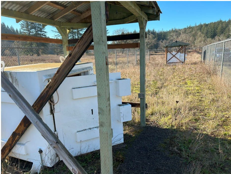
16. Empty Type 2 explosives storage magazines located near 1000-yard range in an unsecured fenced compound.
