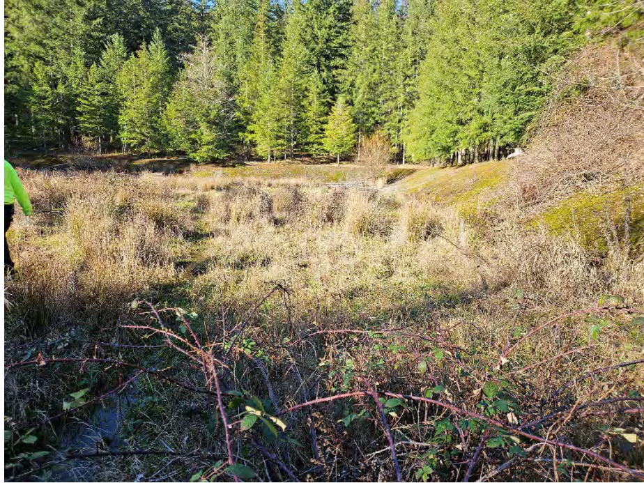
Photo 25. Breach in the western sewage lagoon.
