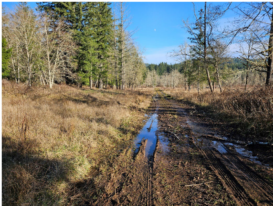
Photo 29. Drainage from lagoon breach reaches access road
