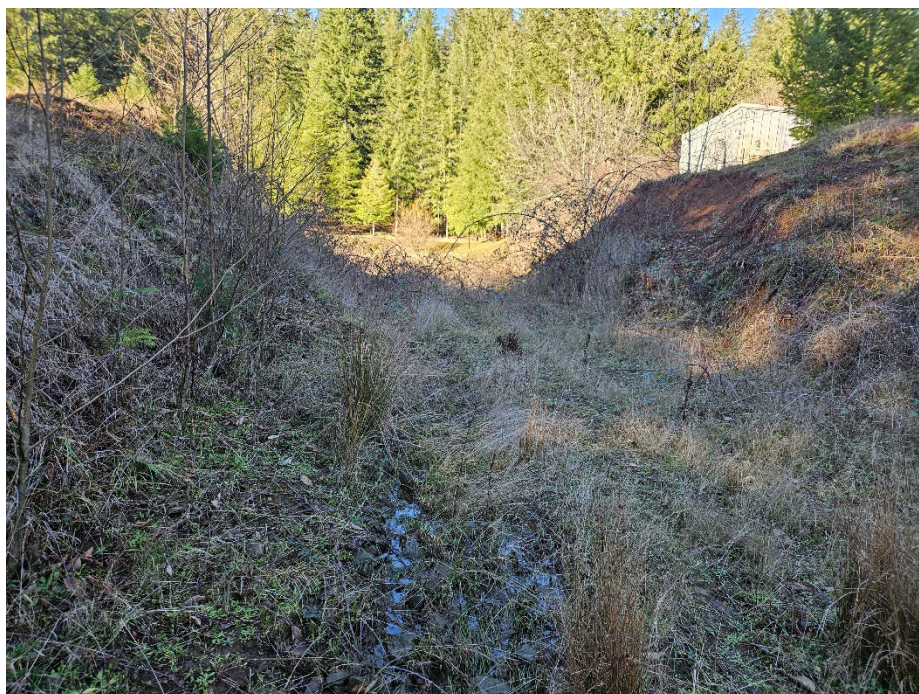
Photo 26. Drainage from lagoon breach
