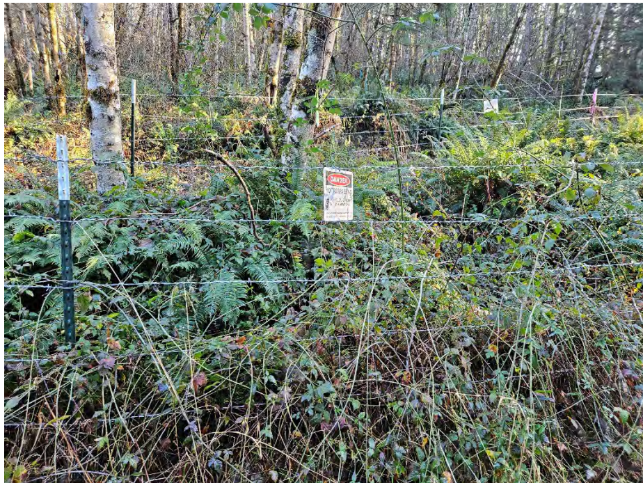
Photo 4. Five-strand barbed wire at CITA expansion.
