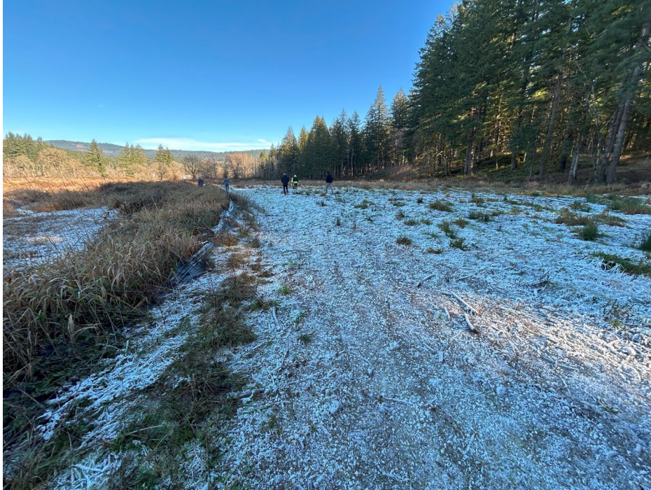
23. RAU-2A-16 soil cap area. Remnants of silt fencing visible in left 1/3 of image.
