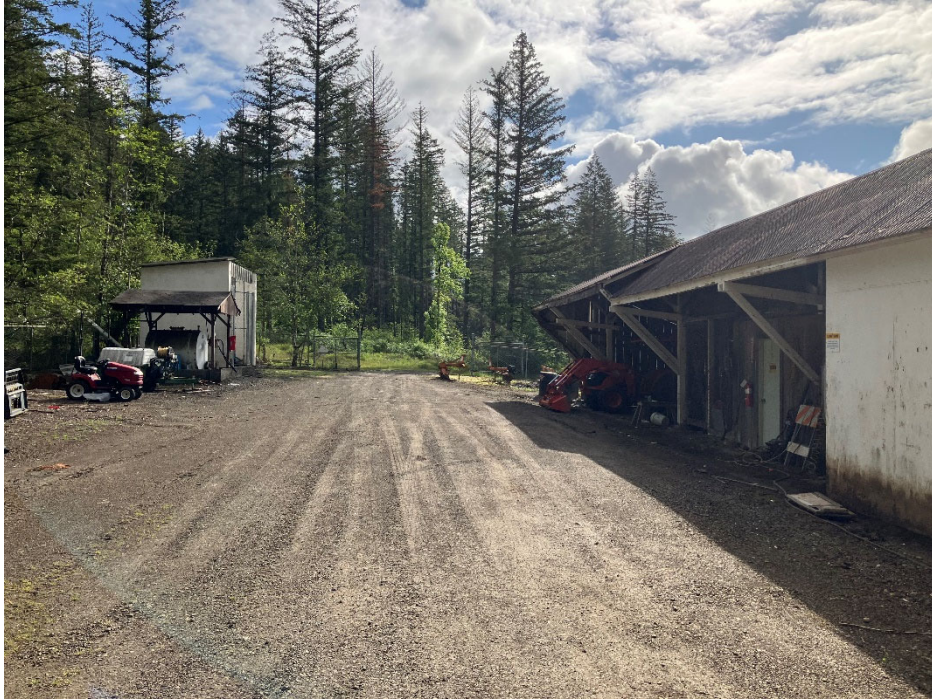
24. Maintenance Yard at Camp Killpack cantonment Facing East.
