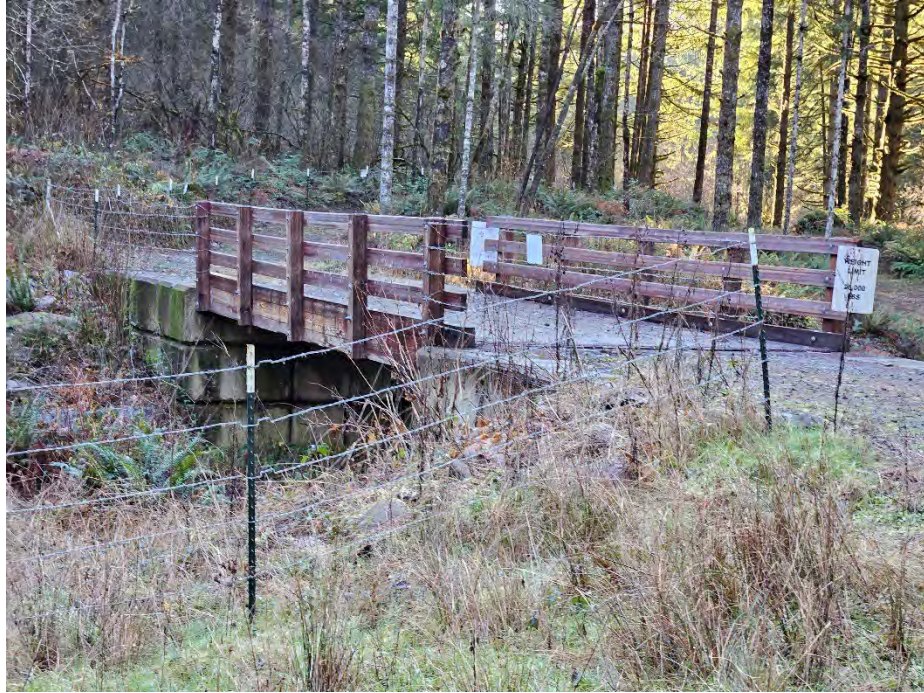
Photo 3. Five-strand barbed wire at Central Impact Target Area (CITA) expansion.
