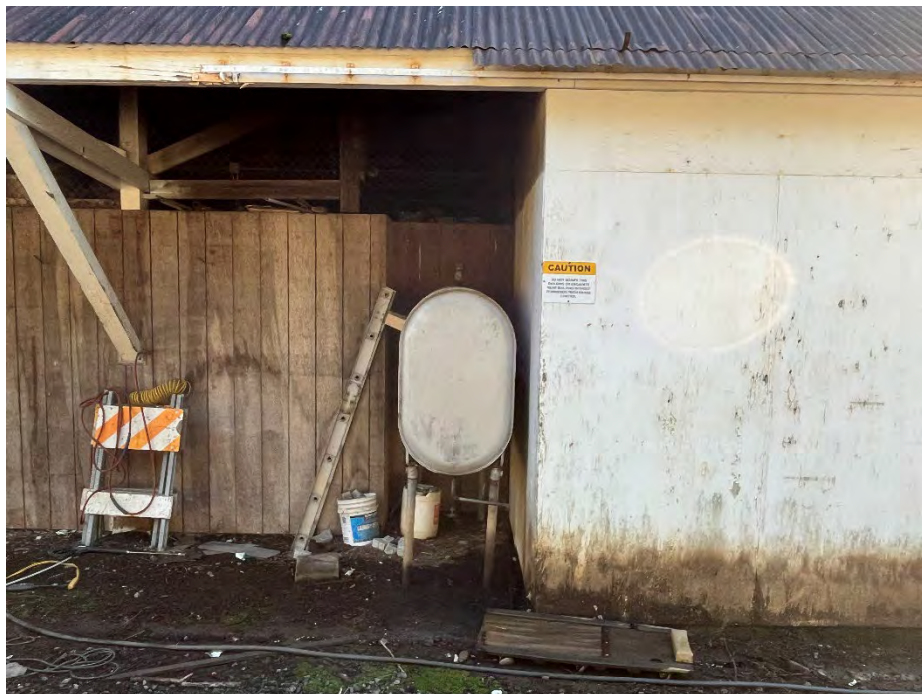
Photo 12. Building 4475 maintenance pit area signage.
