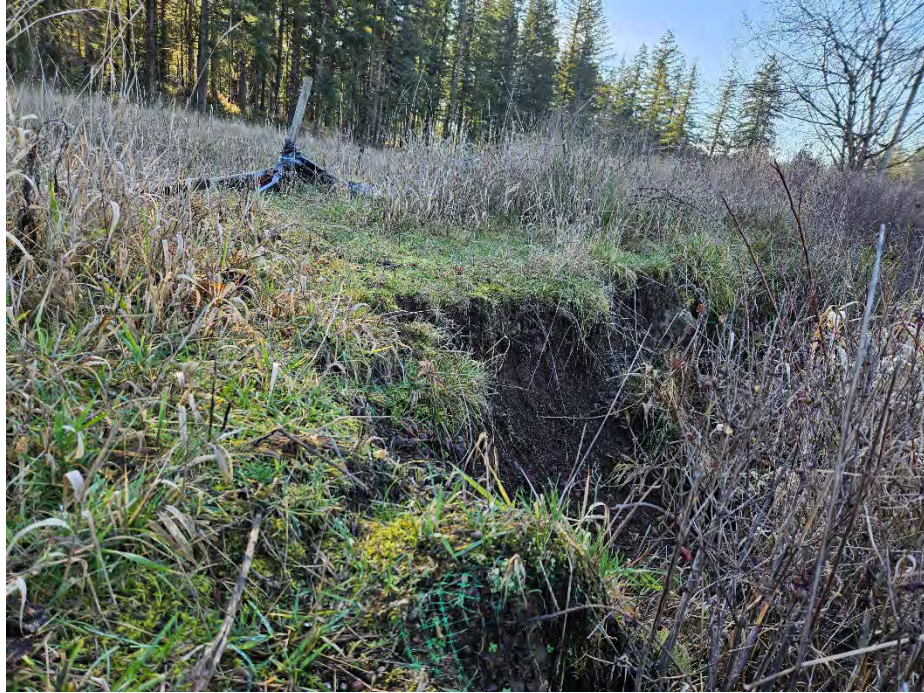
Photo 19. RAU-2A-16 soil cap area: bank erosion 4.5 feet from soil cap.
