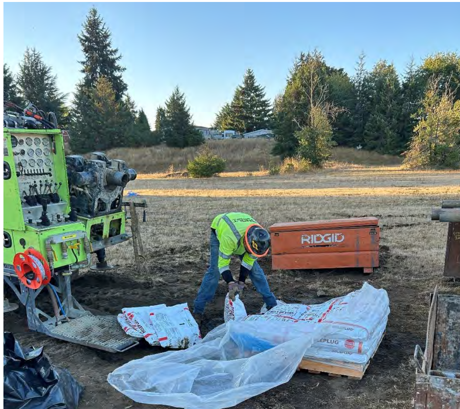
Photo 4: View looking south at Holt drillers backfilling with bentonite chips at LB-5D.
