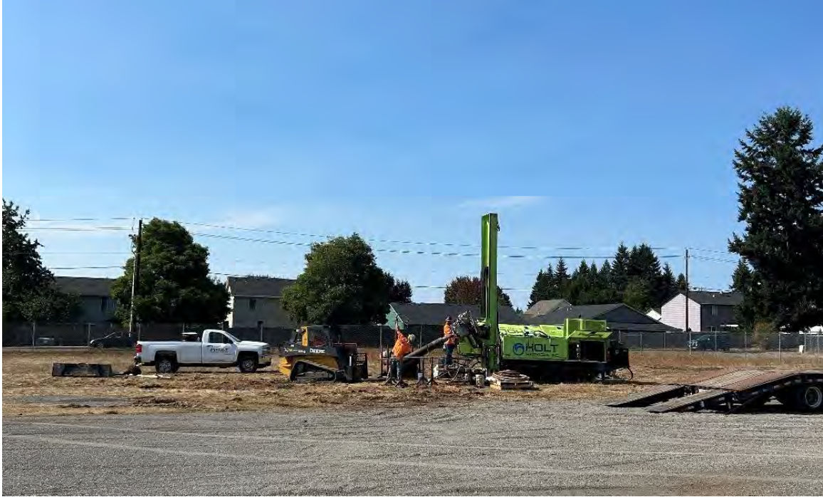
Photo 7: View looking west at the Terra Sonic tracked drill rig stationed at LB-6S.
