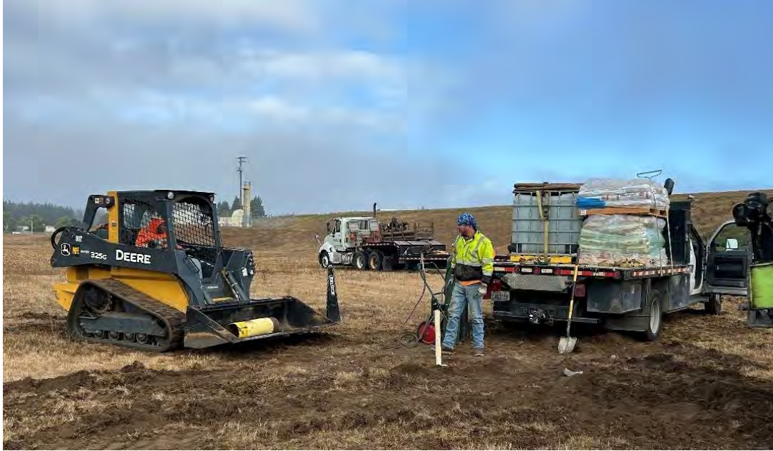
Photo 1: View looking northwest at LB-5D. The image shows the torching equipment used to remove 8-inch above ground metal casing.
