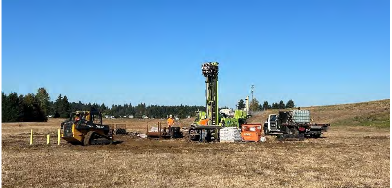
Photo 5: View looking west at the Terra Sonic tracked drill rig stationed at LB-5C.
