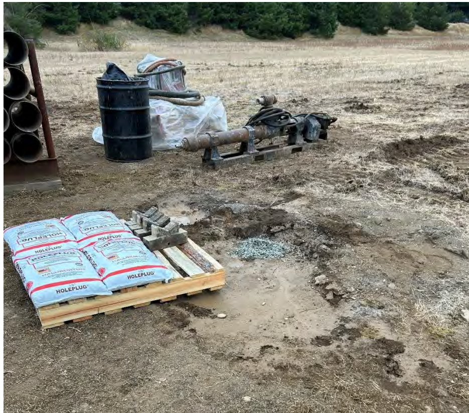
Photo 6: View looking southwest at LB-5S after it was grouted and chipped.
