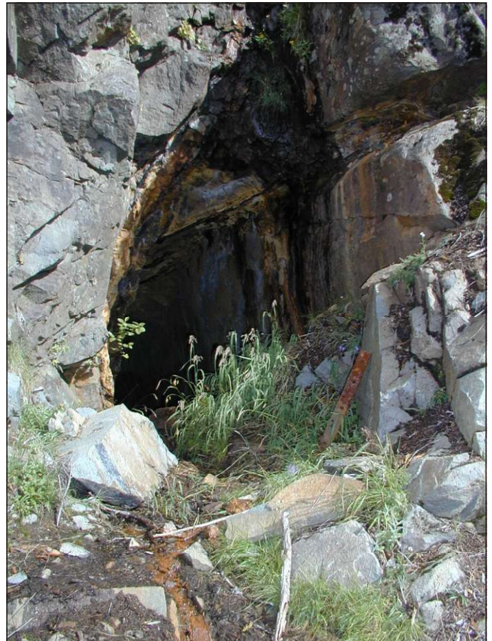
Figure 6. New Discovery adit 2. Note water discharge in lower lefthand corner of photo.
