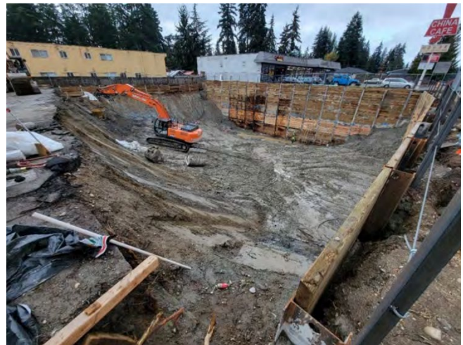
Figure 1 shows the excavation that happened during the Interim Action in 2022. Over 15,000 tons of soil was removed during this cleanup.
