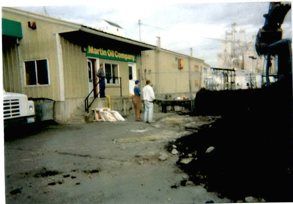
TANK REMOVAL AT S.W. CORNER
