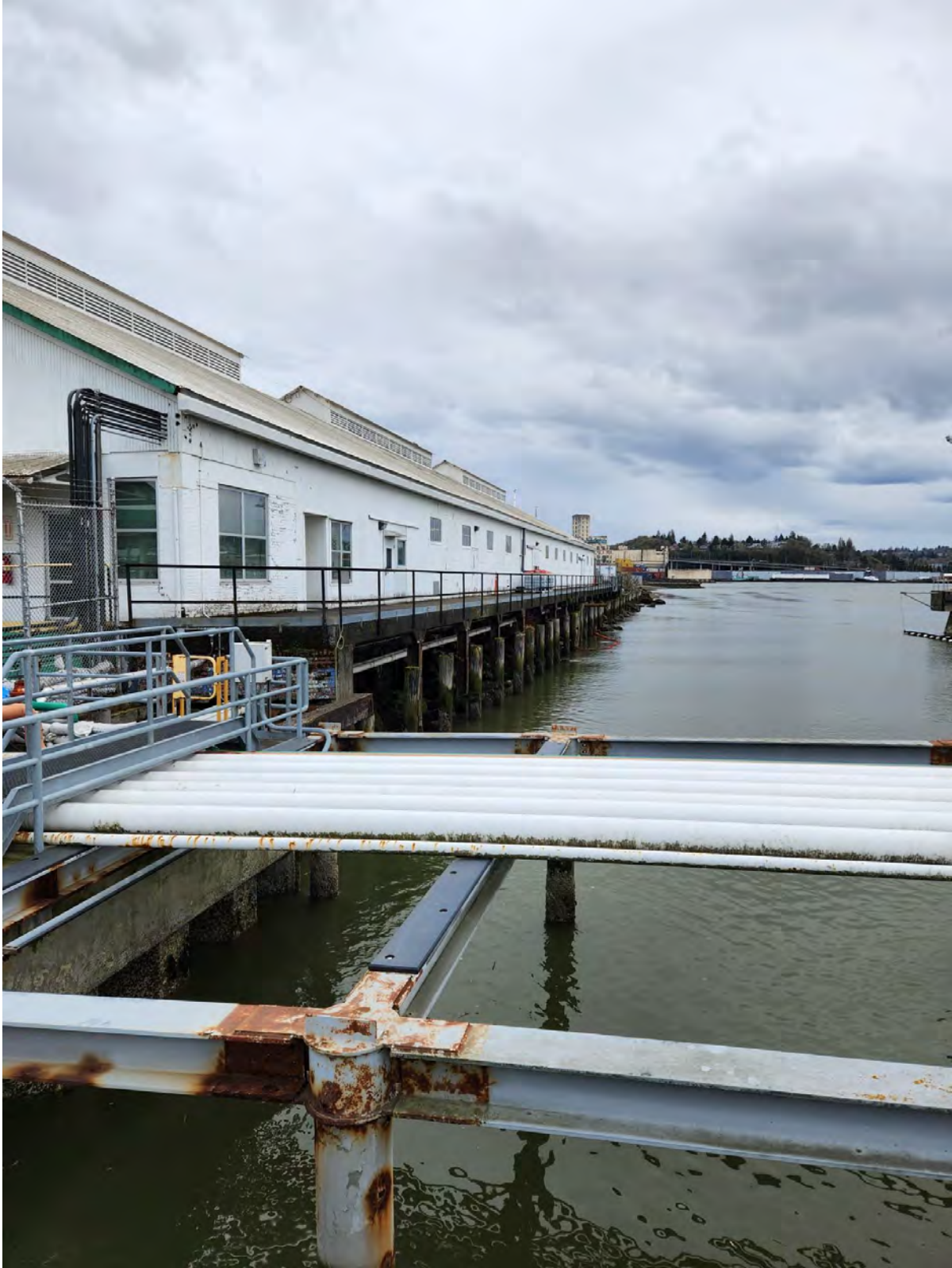
Photo 11. BP-Arco Facility Historic Seawall, Transfer Lines and Warehouse
