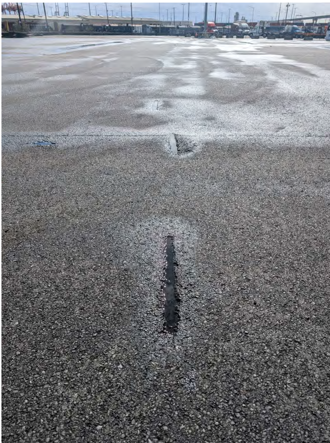
Photo 4. Lockheed Upland Gouges on Cap
