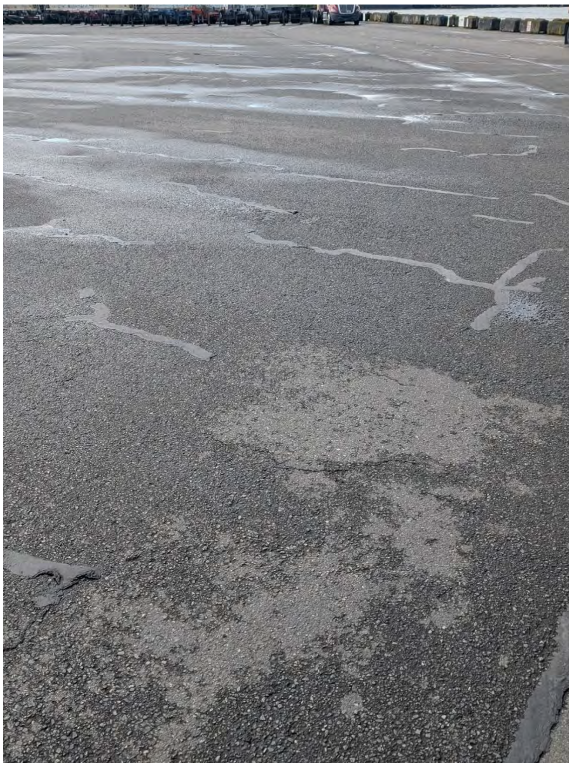
Photo 1. Lockheed Upland Cap with Repaired Cracks
