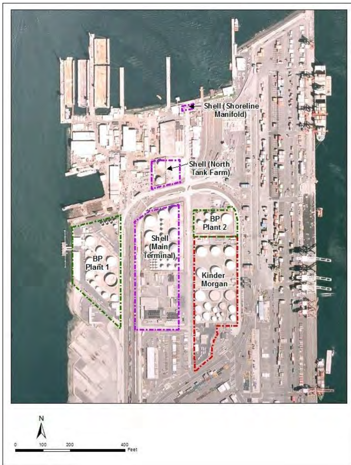
Figure 4. TF-OU2 Tank Farms Facilities
