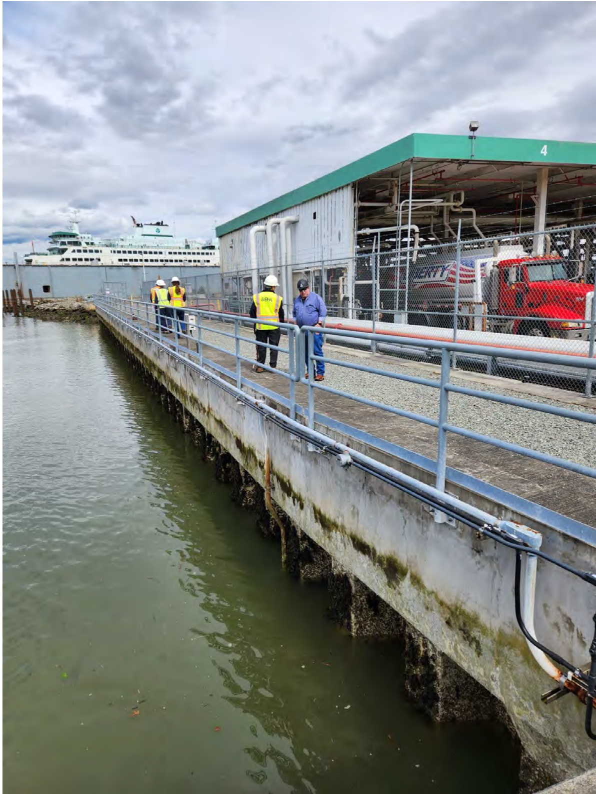
Photo 10. BP-Arco Facility New Seawall
