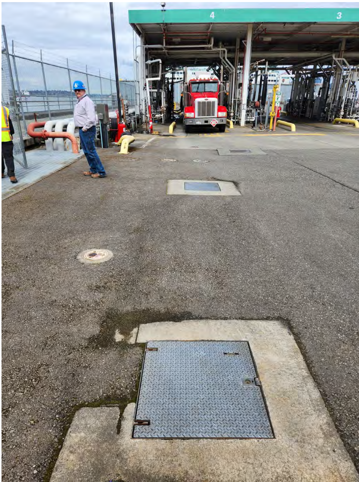
Photo 12. BP-Arco Facility Extraction System Wells
