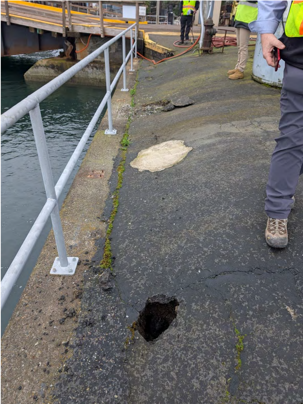
Photo 16. UPRR Parcel A Holes on Western End
