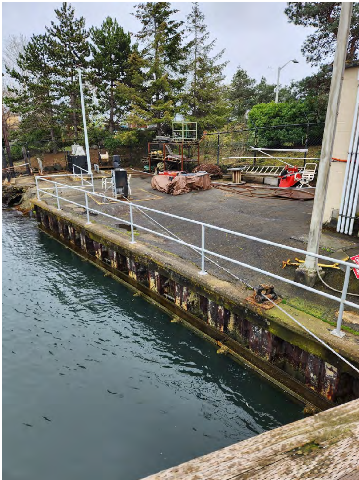
Photo 14. UPRR Parcel A East Seawall
