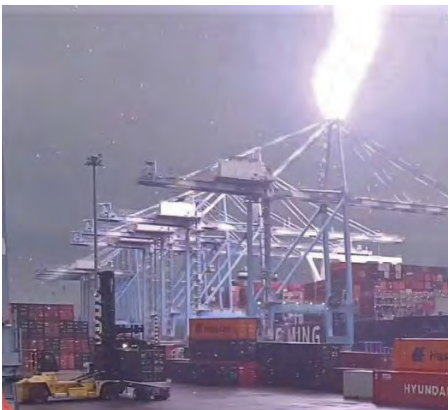
The lightning protection system on one of the port-owned cranes protected it from damage when struck by lightning.
