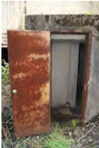
View of door taken 4/26/2010
