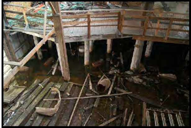
Figures 20-21. Interior view of Building B (roof and wall studs), and viewing from second floor to basement level (note pylons, oldest foundation) and posts on concrete footings (secondary foundation systems for alterations which occurred after original building was constructed).
