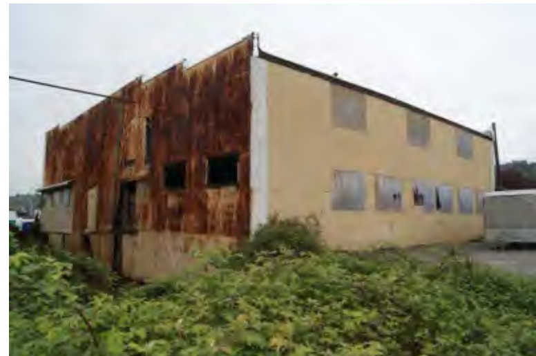
View of south oblique taken 4/26/2010
