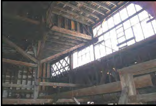
Figures 20-21. Interior view of Building B (roof and wall studs), and viewing from second floor to basement level (note pylons, oldest foundation) and posts on concrete footings (secondary foundation systems for alterations which occurred after original building was constructed).
