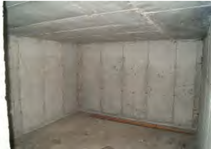
View of Interior of bunker taken 4/26/2010
