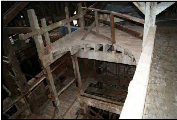
Figures 22-23. Circular framing for original tank (no longer extant) in Building B, and view to elevator shaft from top level of interior.
