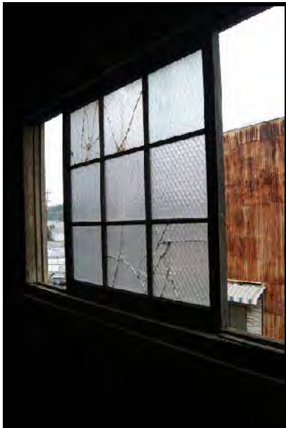
Figures 25-26. Original nine-light safety glass wood sash slider window, and interior space on top floor showing roof rafters.
