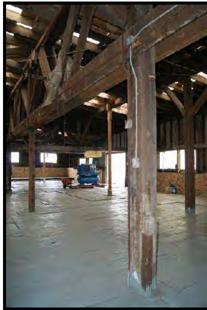
Figures 18-19. Interior view of Building B original support column in foreground, with new replacement post (background), and original door opening, as viewed from interior, showing corrugated metal siding covering opening from the exterior.
