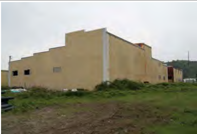
View of south oblique taken 4/26/2010
