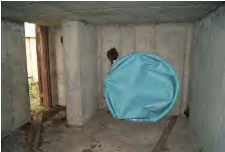
View of Interior of bunker taken 4/26/2010
