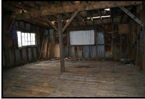
Figure 24. Interior space on top floor (note loss of original windows).
