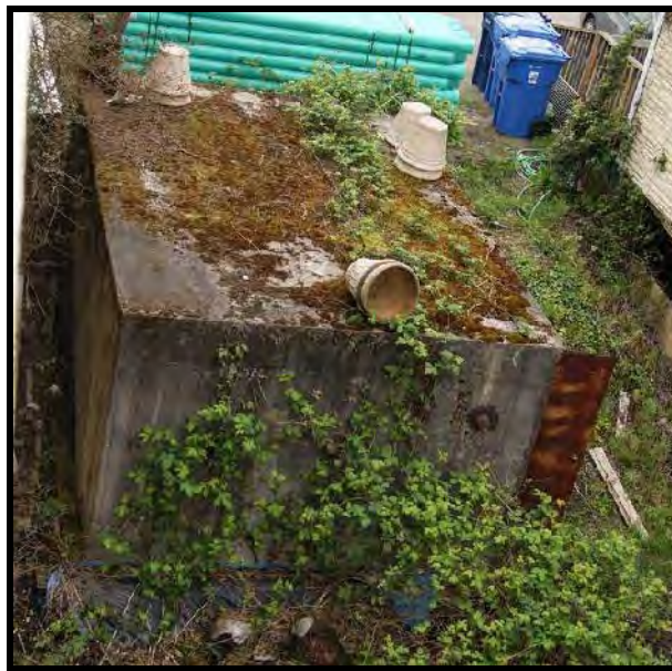
Figure 29. Viewing north, south oblique of concrete bunker from above.
