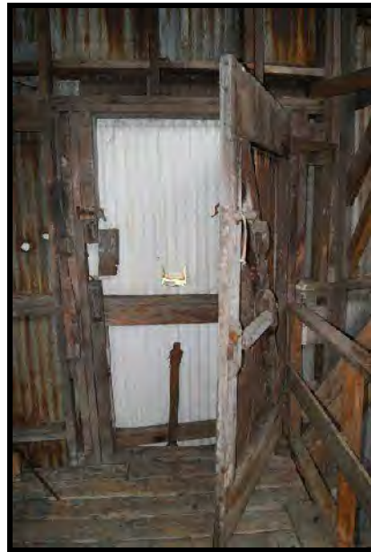
Figures 18-19. Interior view of Building B original support column in foreground, with new replacement post (background), and original door opening, as viewed from interior, showing corrugated metal siding covering opening from the exterior.
