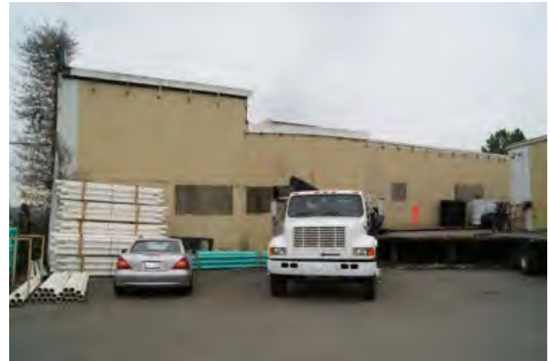
View of northwest elevation taken 4/26/2010
