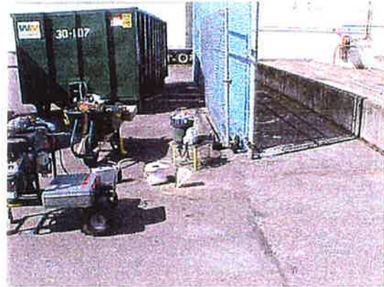
Water sampling at Boring B9.
