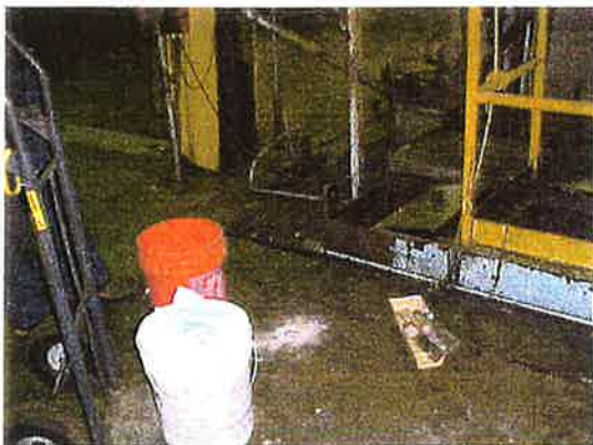
Boring B17 was located within the north end of the plant.
