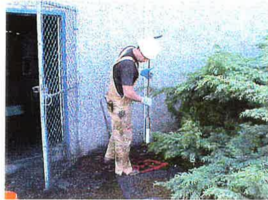
A hand auger was used to drill Boring B2 (shown here) and nearby Boring B1.
