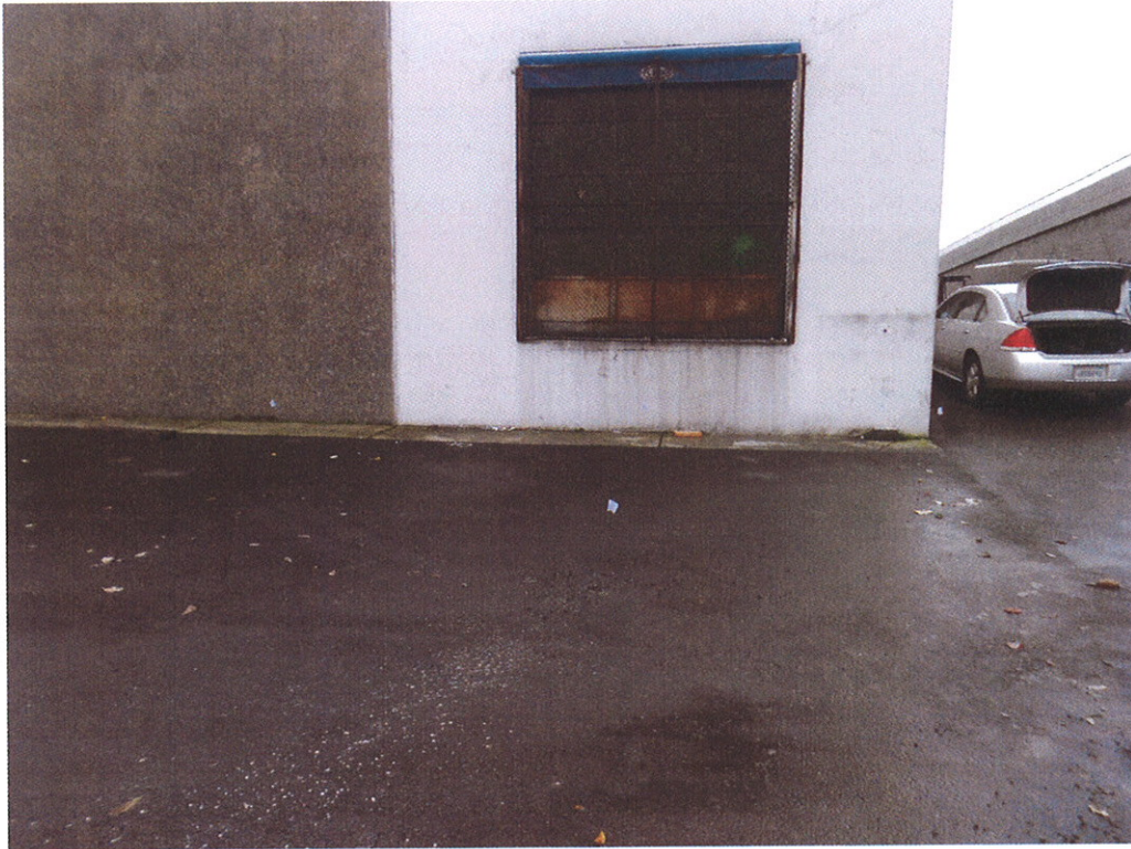
View looking west at the overhead door in the Baler area. The white flags demark soil boring SB209 (foreground) and (left to right) soil borings SB208, SB206, and SB207.
