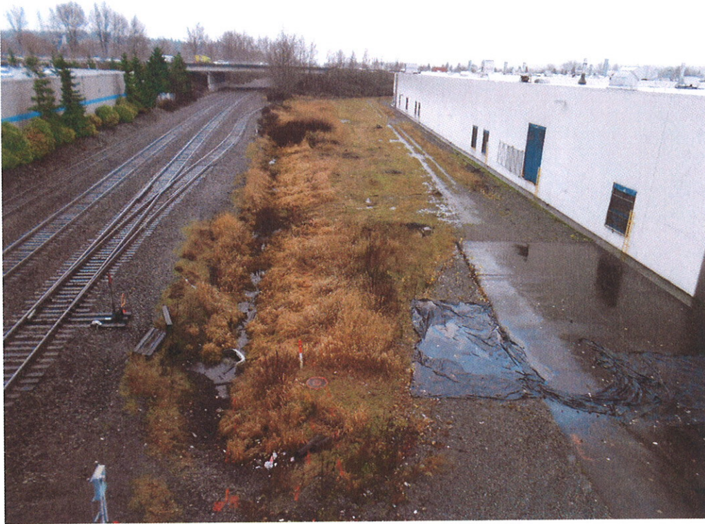
View looking south from the South 228 th Street overpass showing the Manufacturing Building, release area, covered excavation, utility markings and drainage swale adjacent to the railroad main line.
