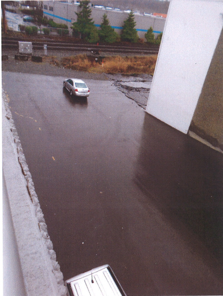
View looking east from the South 228 th Street overpass at the northeast corner of the Site. Note the stormwater flow pattern to the east-southeast with a slight sheen on the asphalt pavement from typical parking lot runoff.
