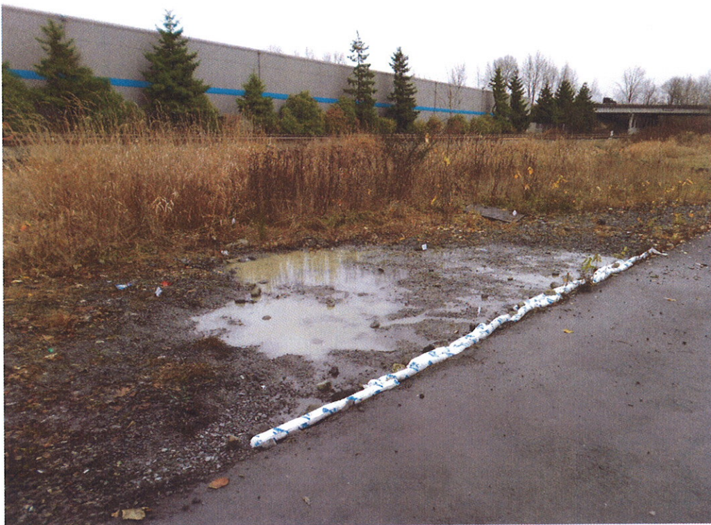
Sorbent socks placed at edge of gravel to capture any sheen on stormwater runoff from the asphalt pavement. White flags demark soil boring locations in center of and on four (4) sides of excavation.
