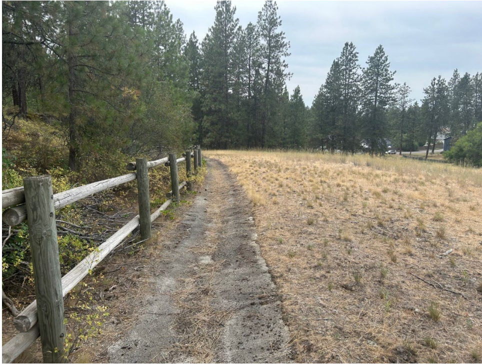
Photo 5: Southern drainage trench and fence— from the east
