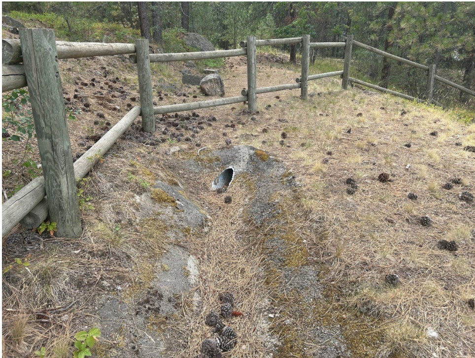
Photo 6: Southern drainage trench, culvert, and fence — from the east
