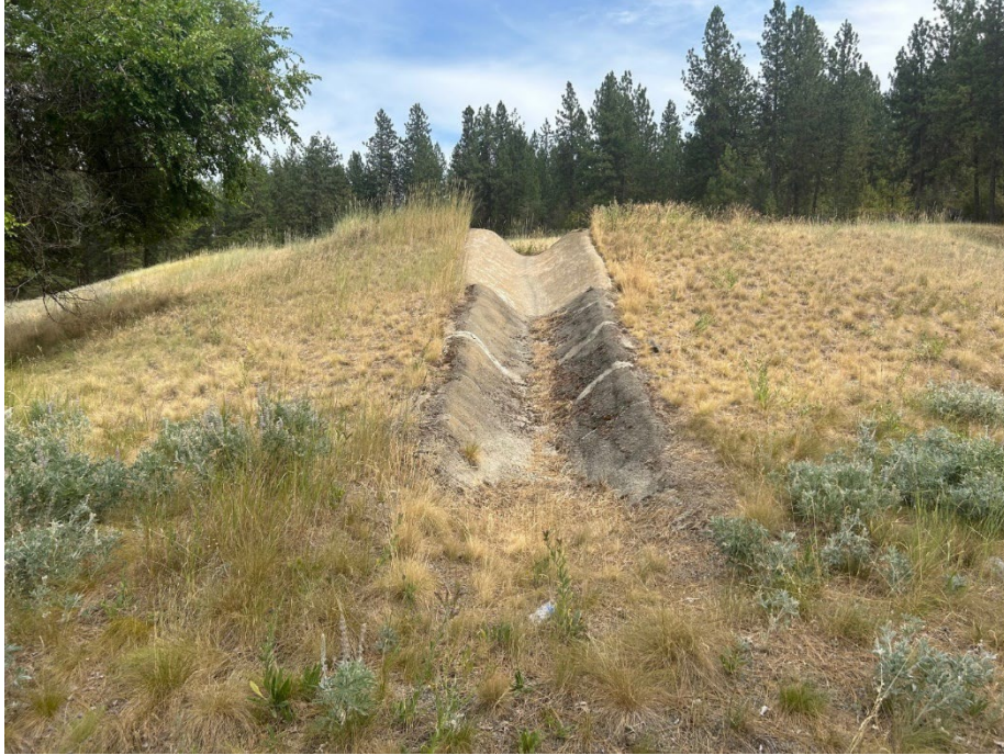
Photo 1: Northwest drainage trench — from the northwest
