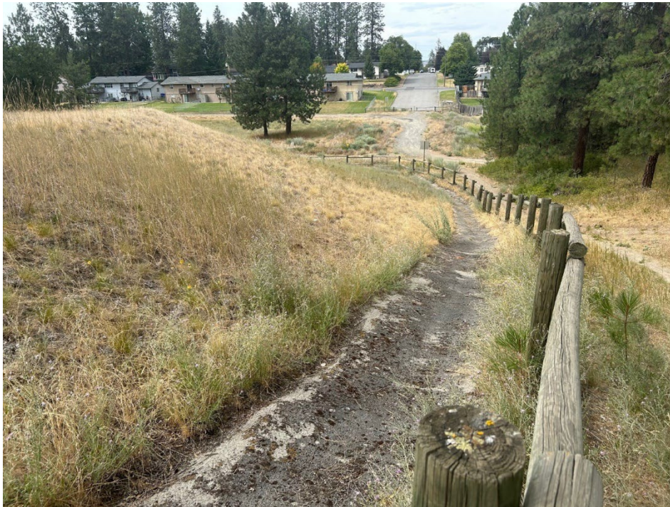
Photo 4: Eastern drainage trench and fence— from the south
