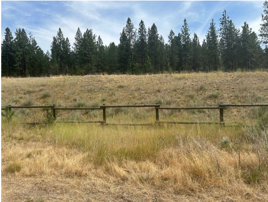
Photo 2: Northern landfill slope and fence — from the north
