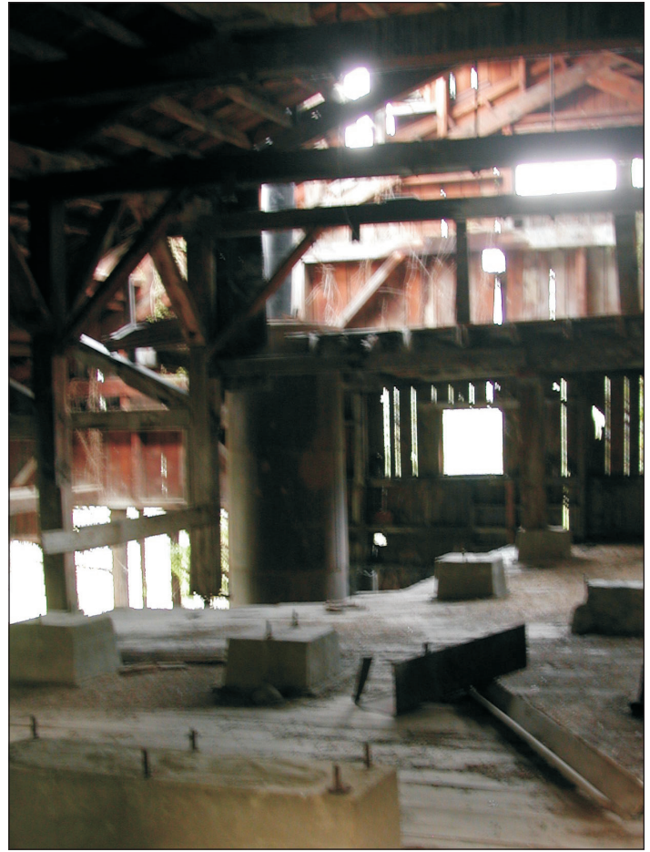
Figure 4. Mill building interior with footings.
