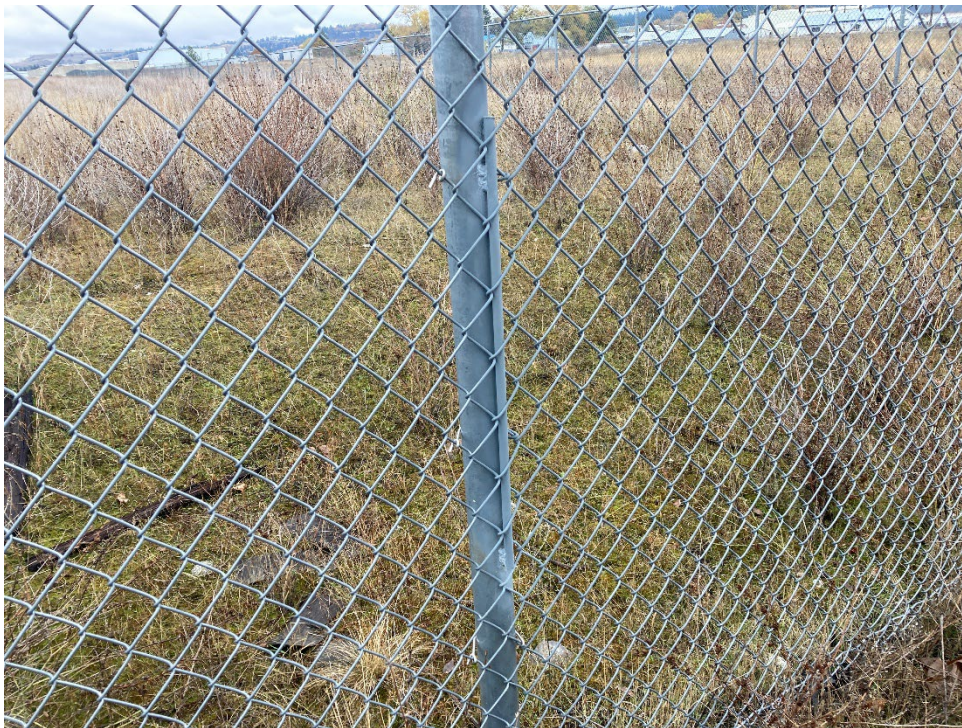
Photo 6: Welded post to reinforce perimeter fence — from the south
