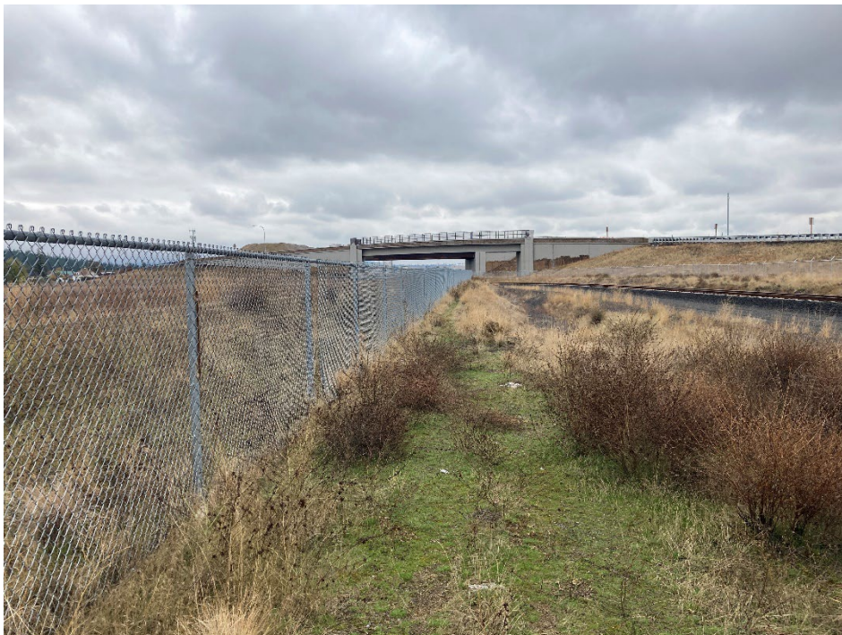
Photo 2: Western perimeter fence and BNSF railway — from the north
