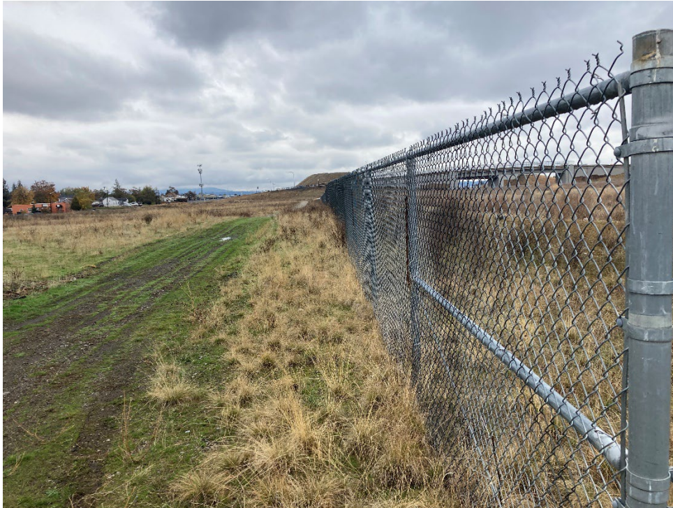
Photo 3: Eastern perimeter fence with welded reinforcement — from the north
