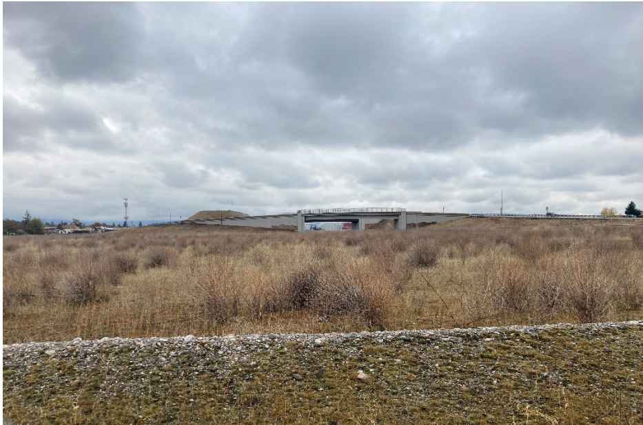
Photo 1: Capped containment area with sloped perimeter — from the north
