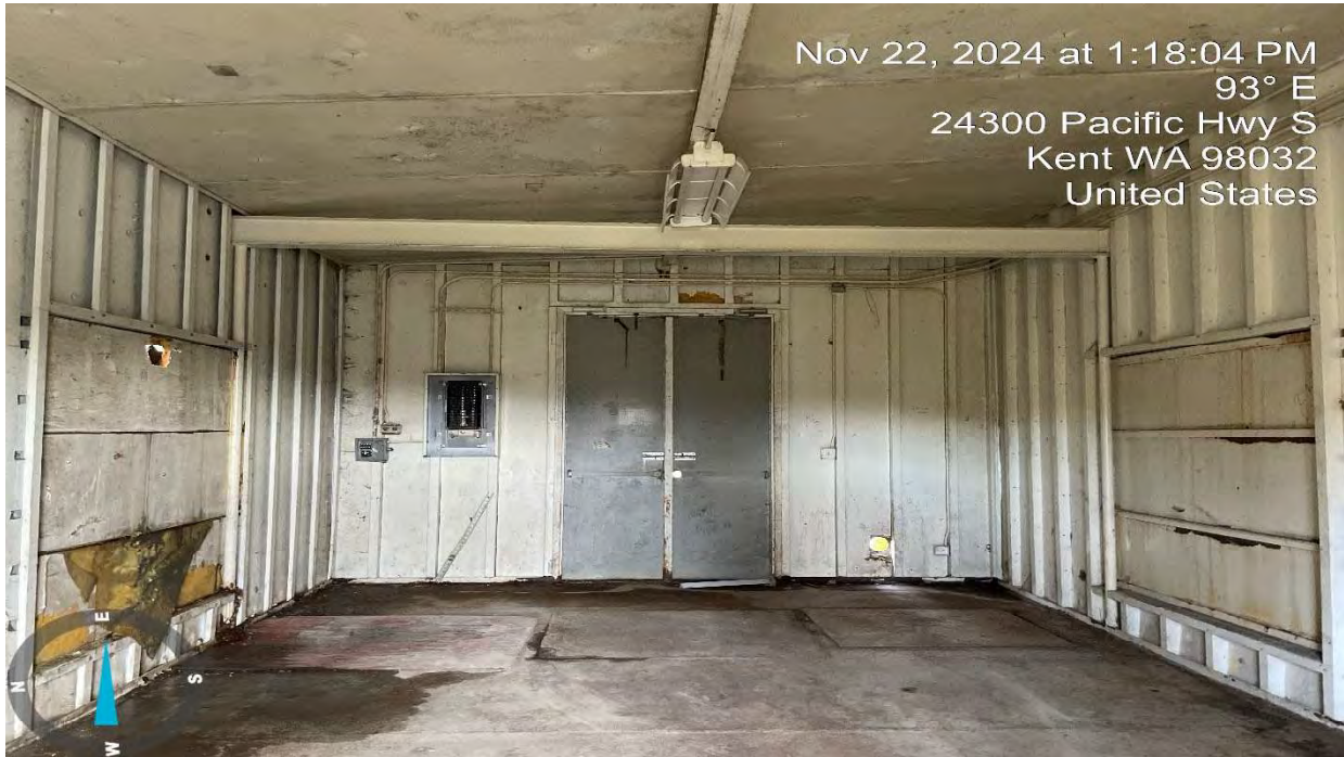
5. Interior of shed/storage building (Viewing E)
