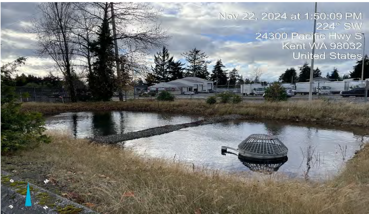
20. Settling pond (Viewing SW)
