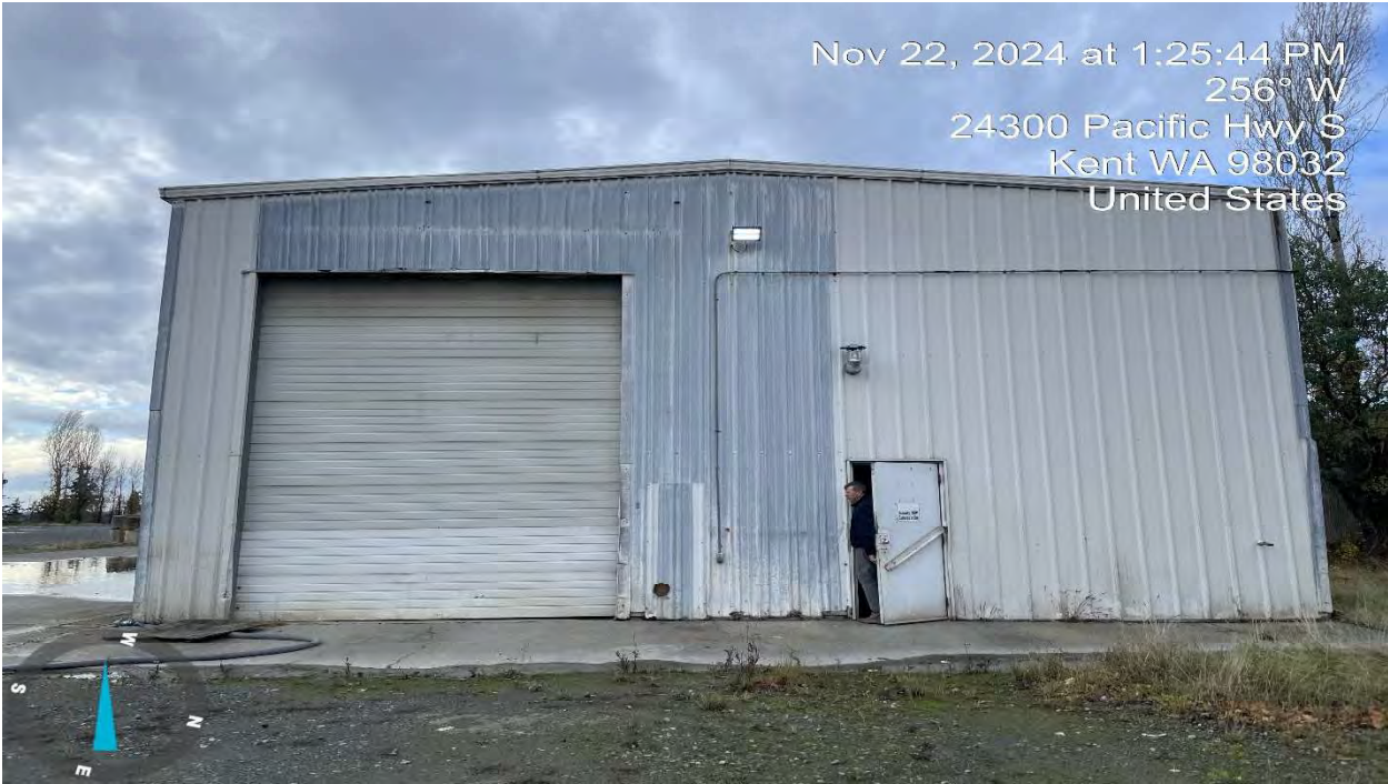
7. Maintenance garage building (Viewing W)
