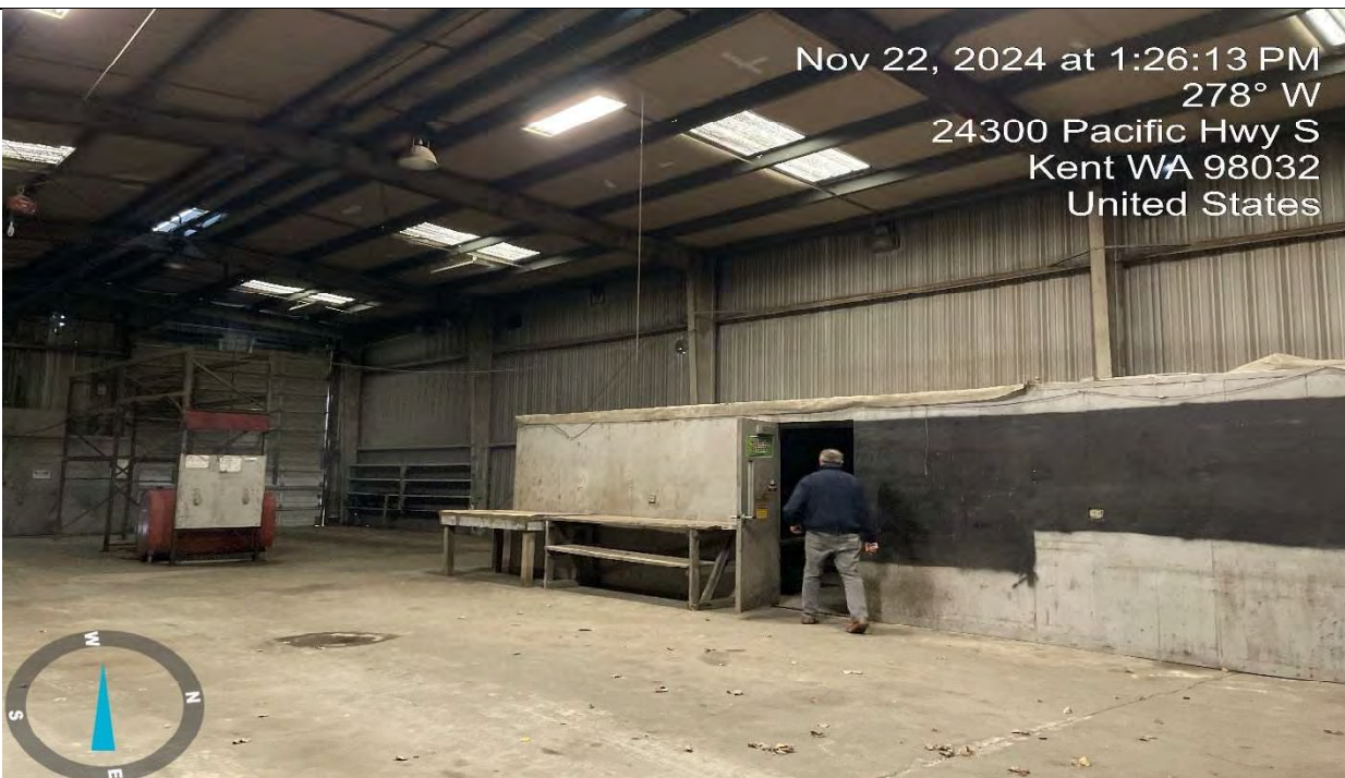
22. Interior of maintenance garage building and makeshift office/storage area (Viewing W)
