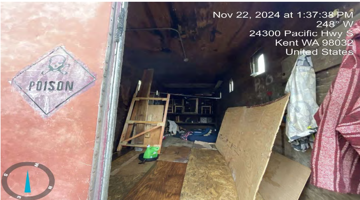
14. Interior of storage trailer (Viewing W)
