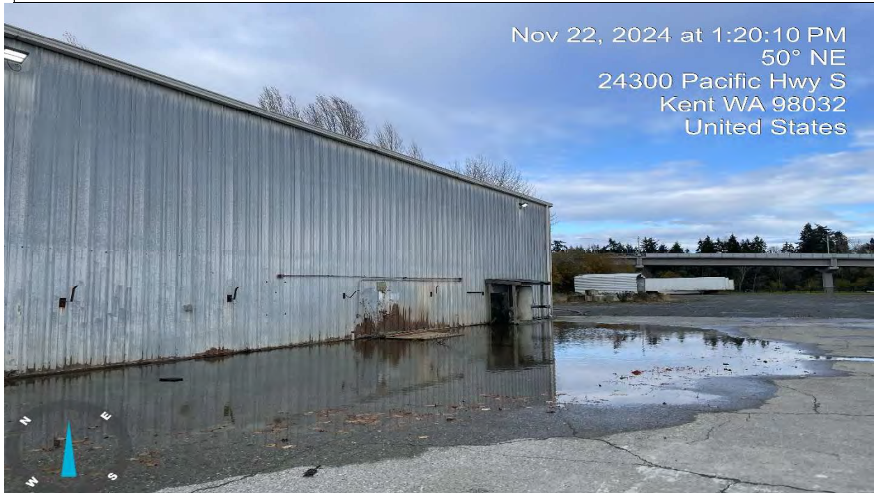
6. Southern side of maintenance garage building with sump (covered by plywood) and vacuum near center of photo (Viewing NE)
