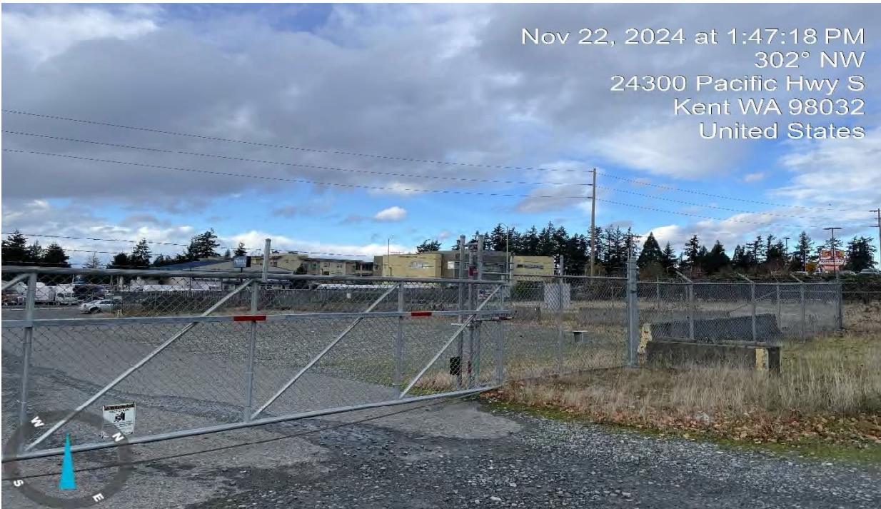
19. Entrance gate (Viewing NW)
