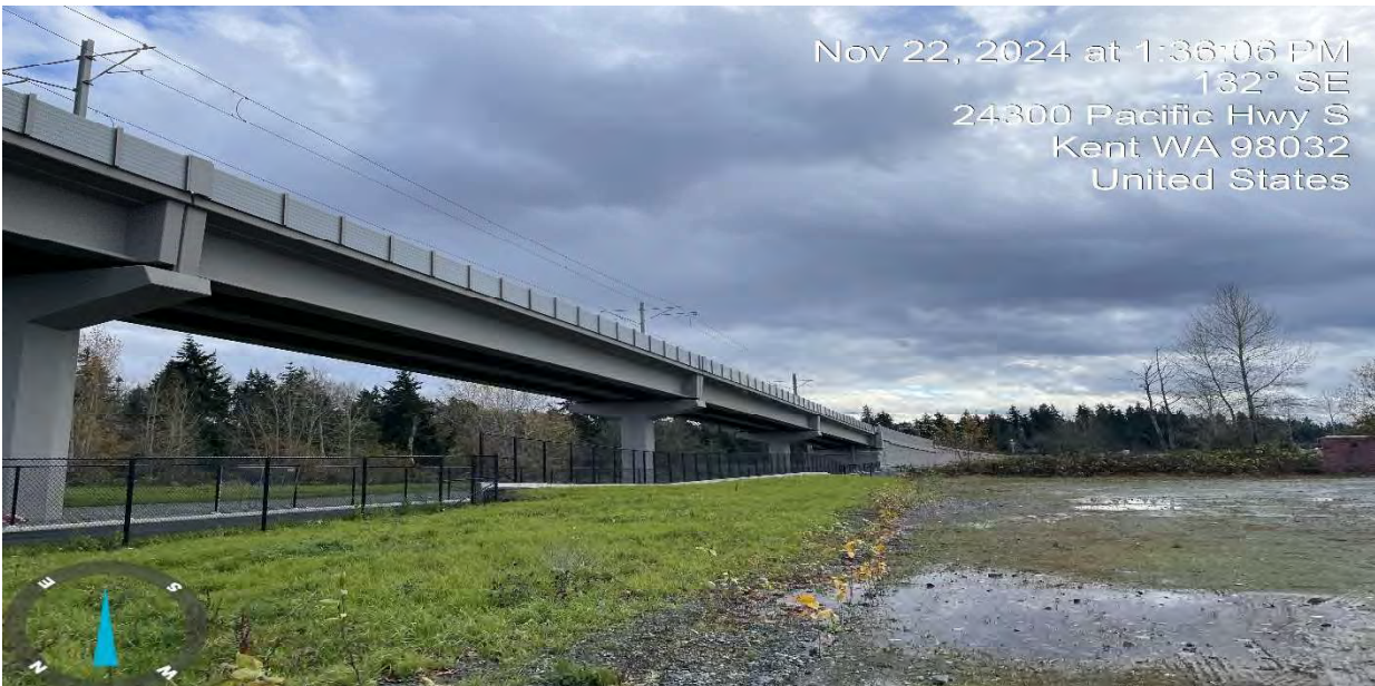
12. Sound Transit easement on far eastern portion of the Subject Property (Viewing S-SE)
