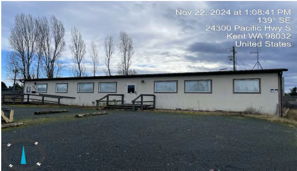
1. Front view of office building (Viewing S-SE)
