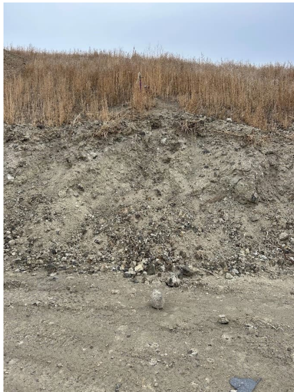
Typical Thermistor Installation Access Exposed Face
