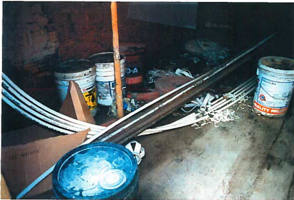
FIGURE 14 The welding contractor has several containers with the hazardous materials used in his operation stored inside small trailer containers and on wooden pallets.
