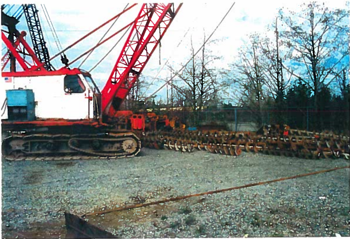
FIGURE 9 Top and bottom views of construction equipment stored on the very east end of the subject property.
