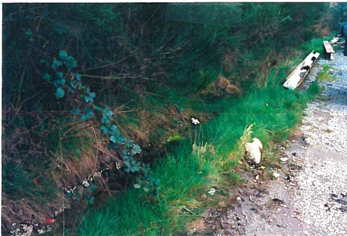
FIGURE 19 Top view of the small run-off water collection ditch located on the north side of the subject property adjacent to the maintenance building. Bottom view of the electrical utility system used by the maintenance building operation.
