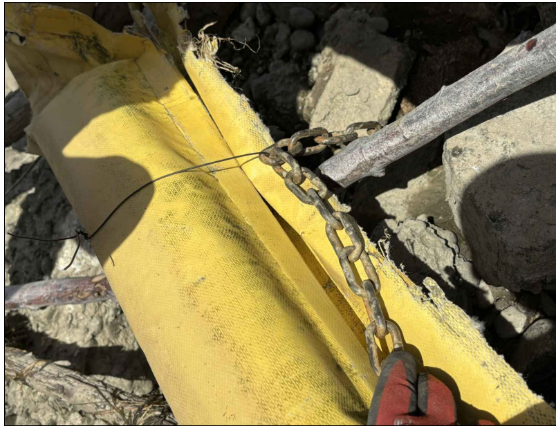
PHOTO 5 Set boom anchor.
