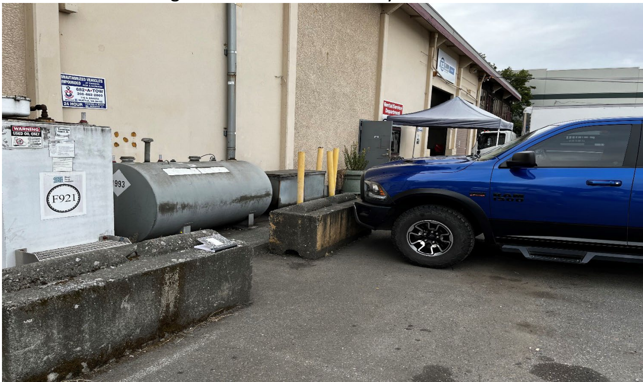
Photo 4: Former UST excavation area and area with contaminated soil beneath the building. ASTs without secondary containment observed.
