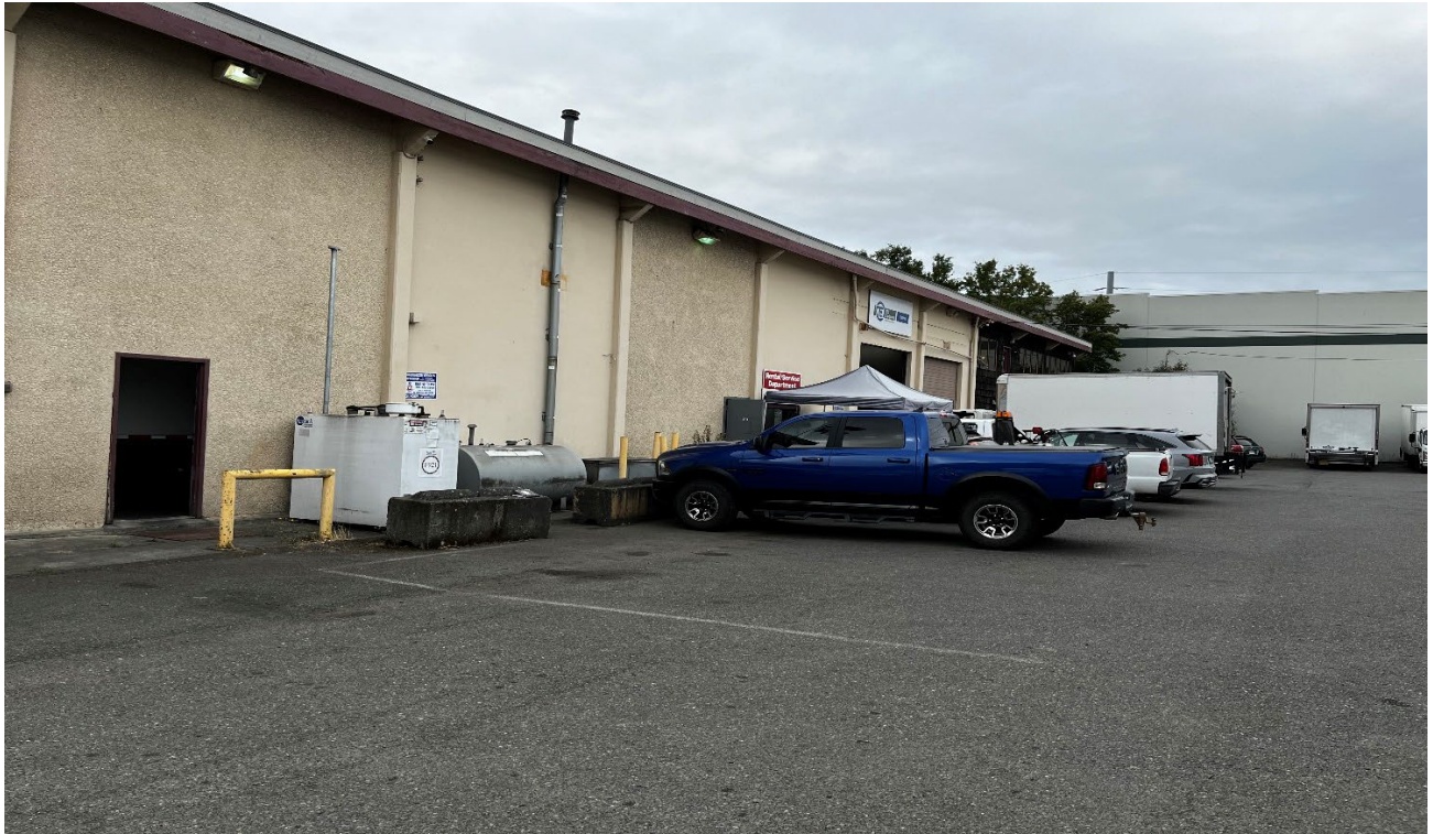
Photo 4: Former UST excavation area and area with contaminated soil beneath the building. ASTs without secondary containment observed.
