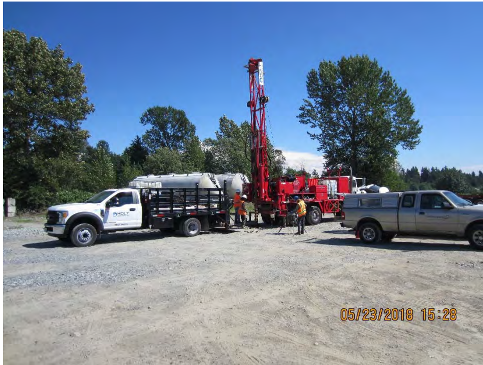
Photograph 5 – FL-252 – Exploration FL252-B3 in the central-eastern portion of the subject property, view looking southeast.
