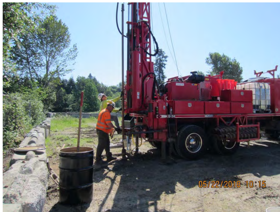
Photograph 4 – FL-252 – Exploration location FL252-B2 that was completed as a monitoring well, view to east.
