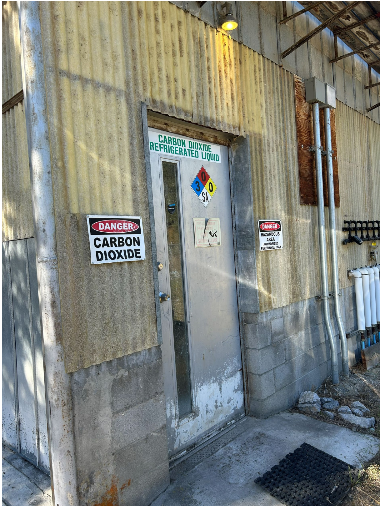
Photo 3: Support building hazardous materials signage
