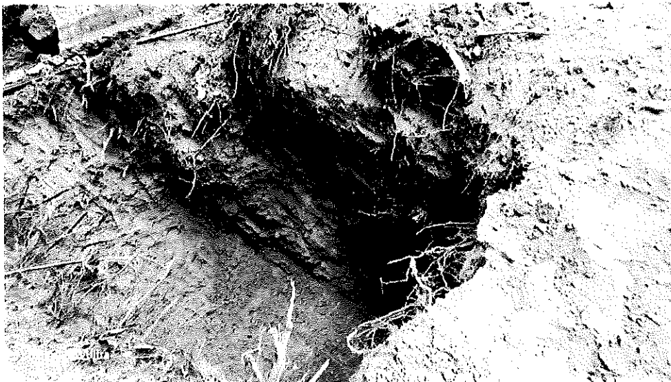
Photo of the NW side of the excavation pit after the removal of 32.43 tons of PCS.
