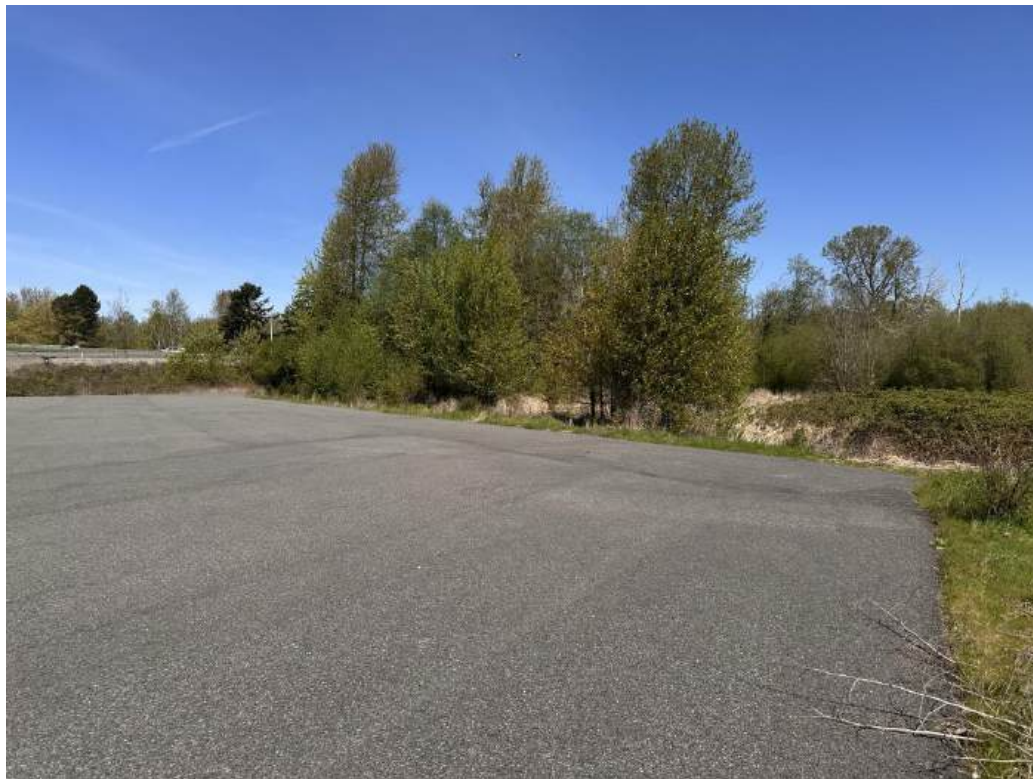
Photograph D6. Station DMCA 06 in good condition.
