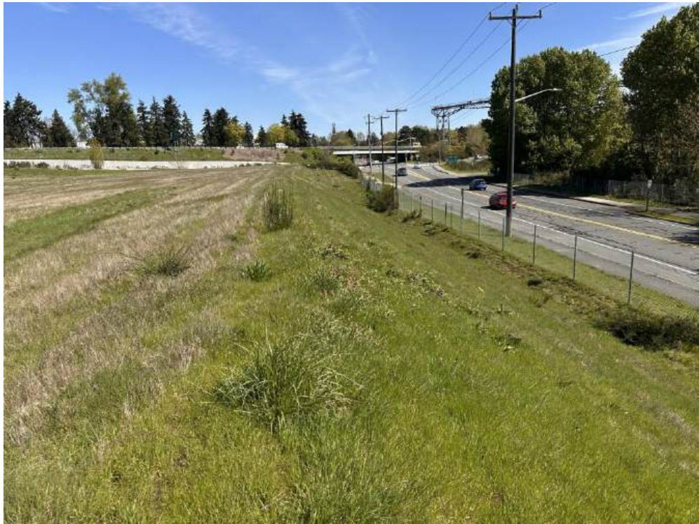
Photograph L16. Station LLA 16 in good condition.
