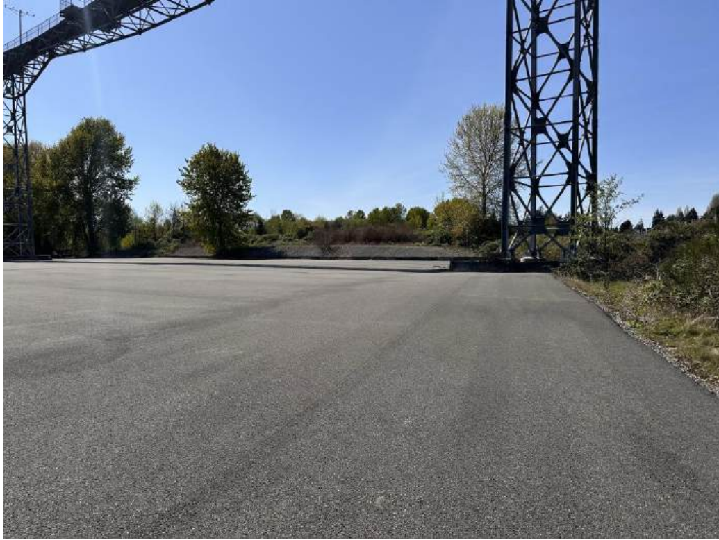
Photograph D3. Station DMCA 03 in good condition.
