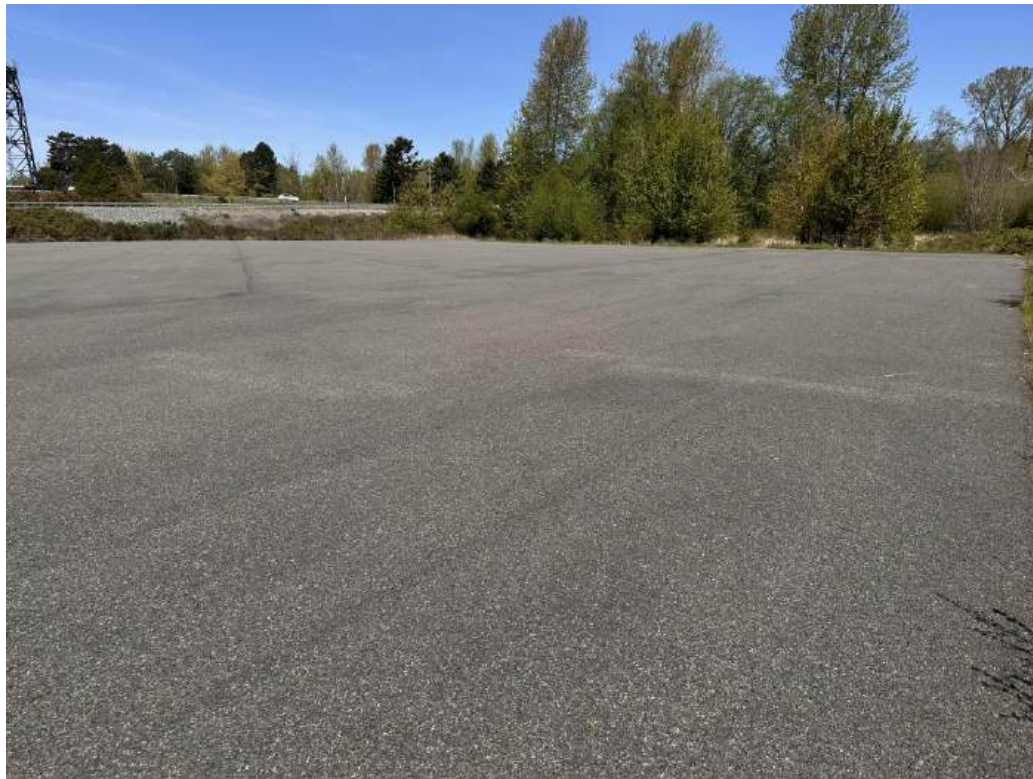
Photograph D7. Station DMCA 07 in good condition.
