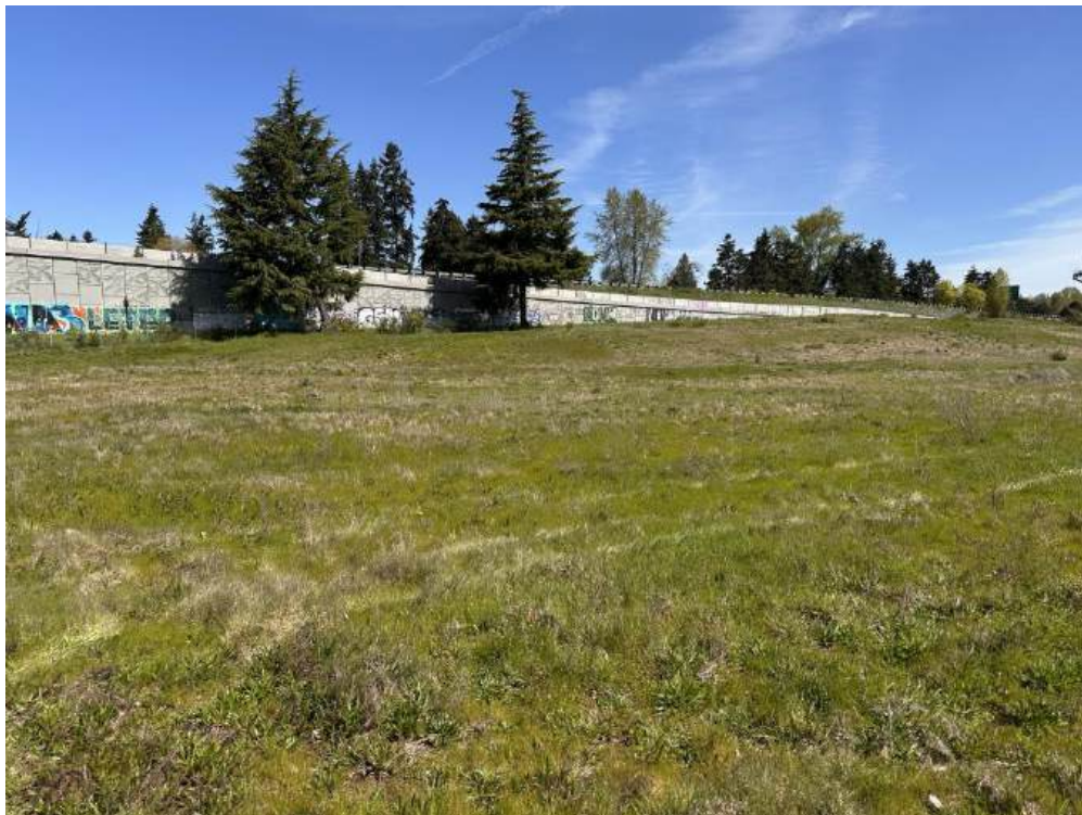
Photograph L24. Station LLA 24 in good condition.
