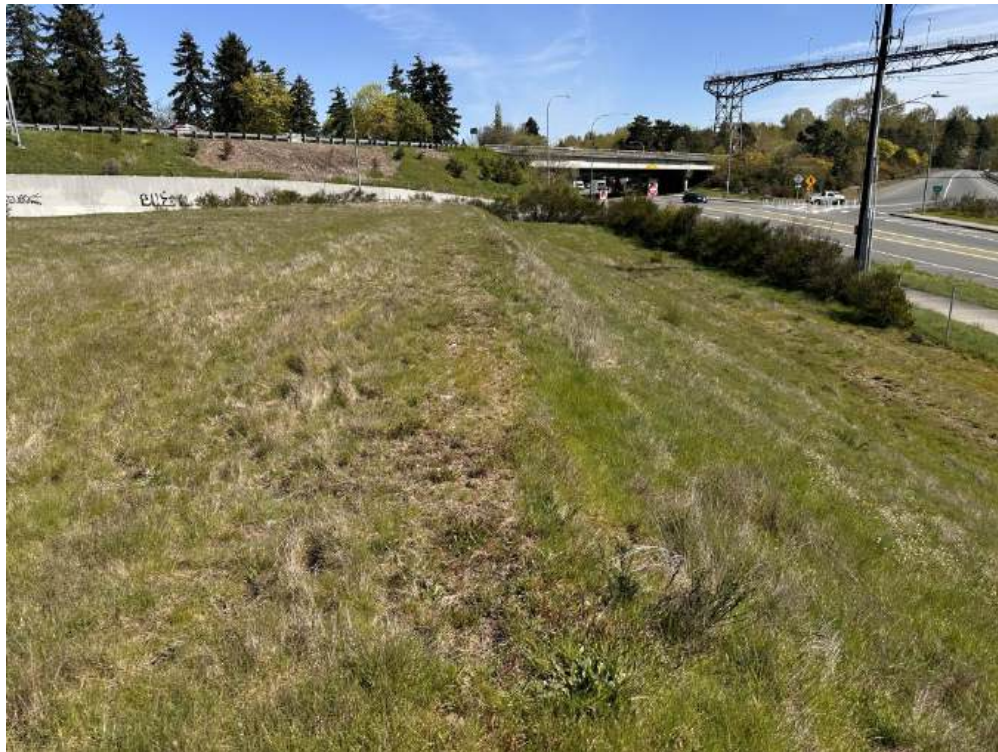
Photograph L1. Station LLA 01 in fair condition with some exposed underlying soil.
