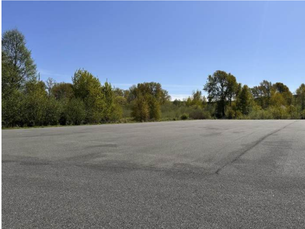
Photograph D13. Station DMCA 13 in good condition.
