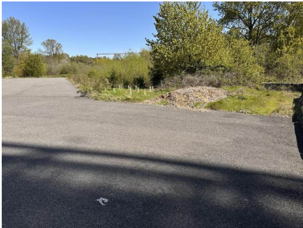
Photograph D8. Station DMCA 08 in good condition.
