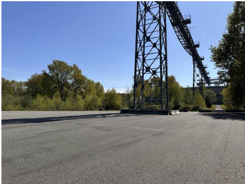
Photograph D10. Station DMCA 10 in good condition.
