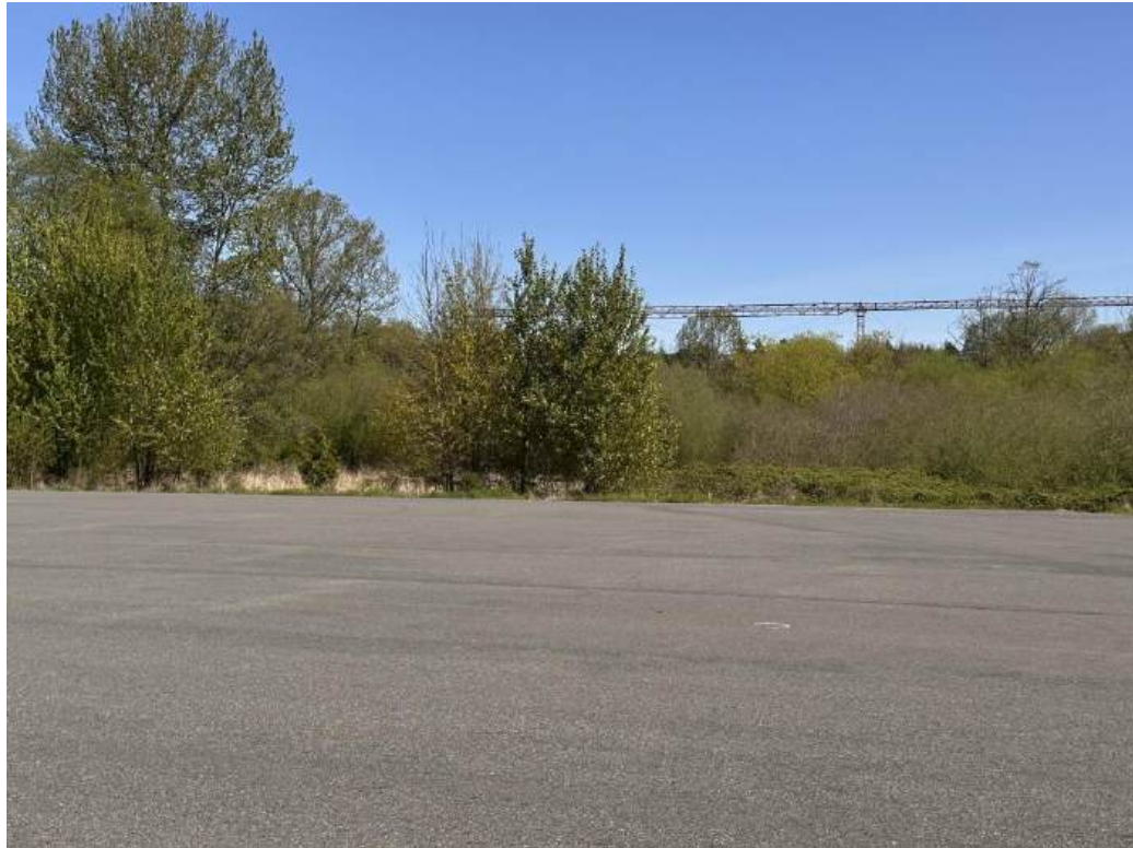
Photograph D11. Station DMCA 11 in good condition.
