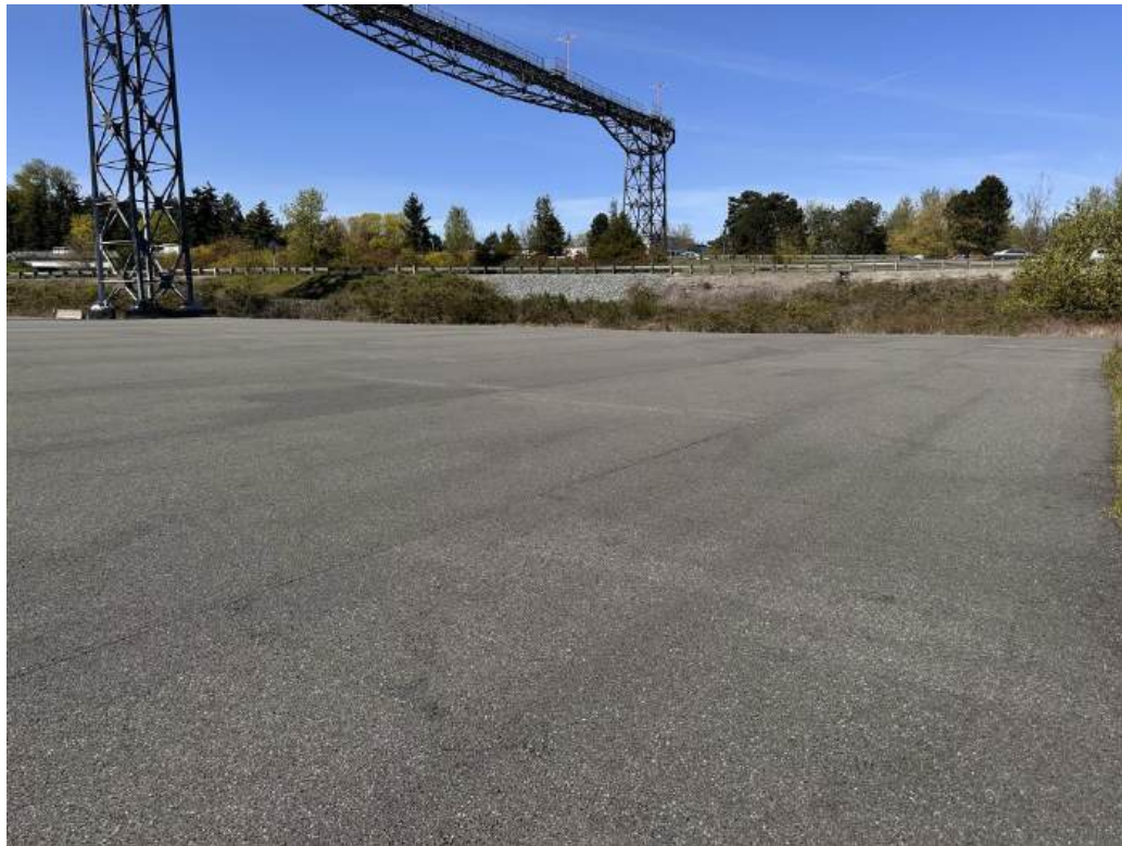
Photograph D5. Station DMCA 05 in good condition.
