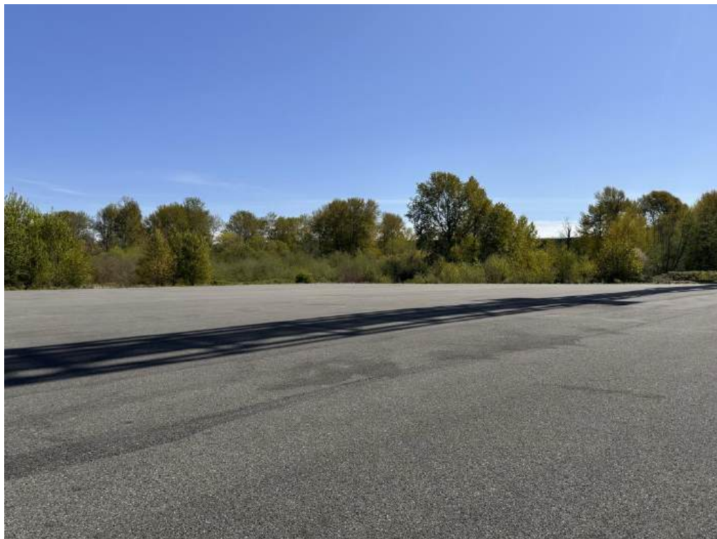
Photograph D12. Stations DMCA 12 in good condition.
