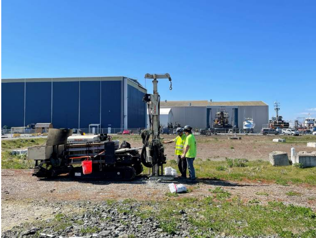
Figure 8. View of boring I13, looking northwest.
