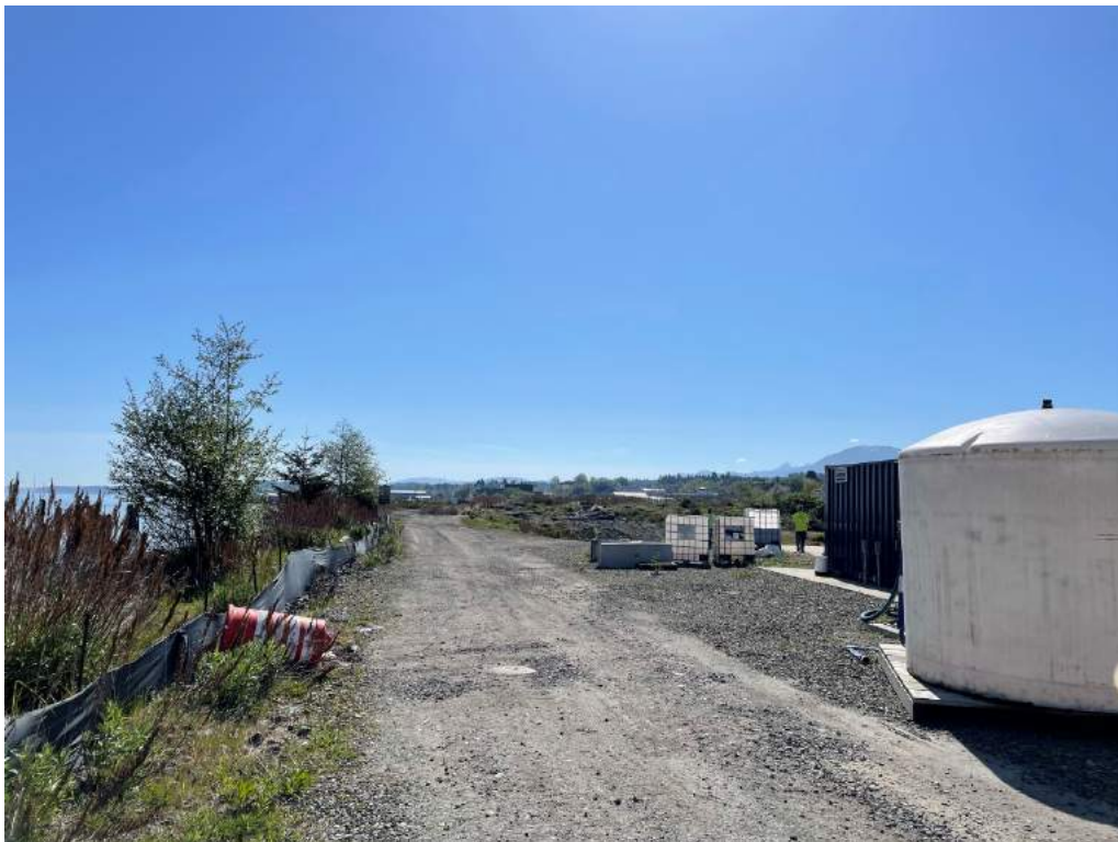
Figure 7. Overview of northern portion of KPLY Mill Cleanup project area, looking east.
