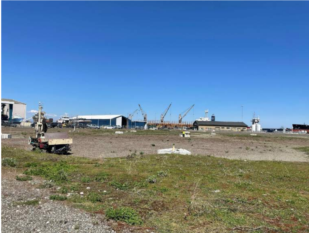
Figure 5. Overview of KPLY Mill Cleanup project area from southwest portion of project area, looking northwest.
