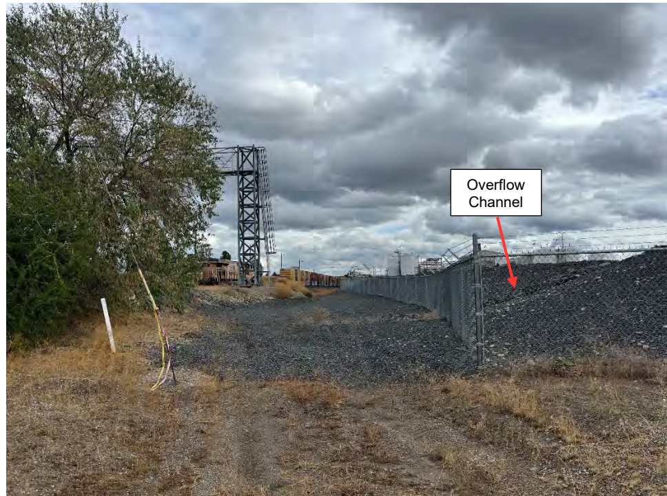
Railroad ditch and overflow channel. View looking east-northeast.
