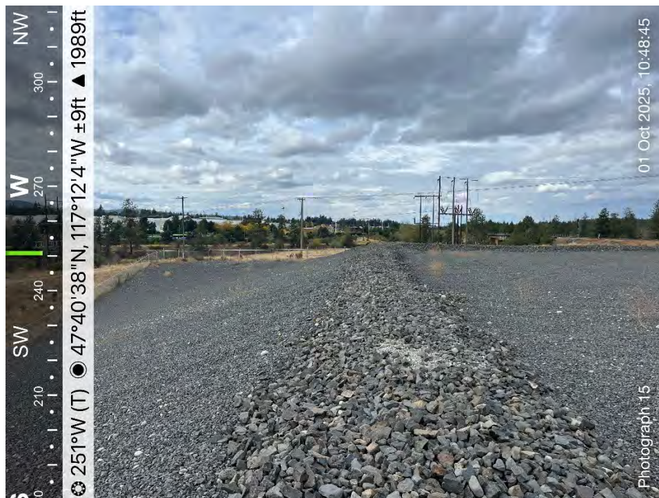
South berm overview. View looking southwest.
