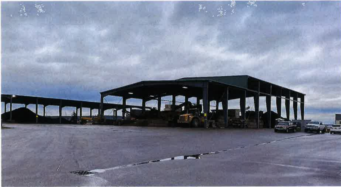
Photo 1: Soil Thermal Desorption Facility operated by Cadman.
