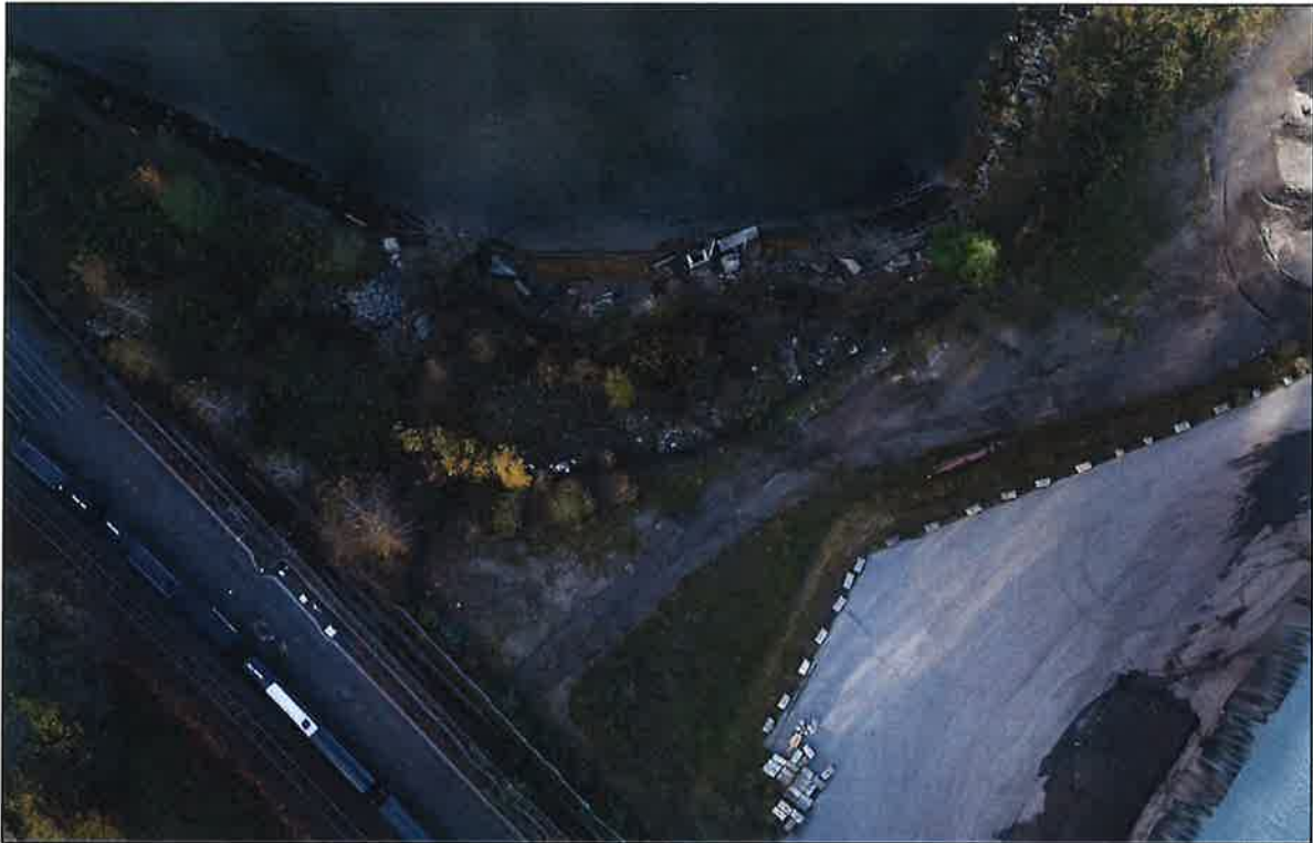
Figure B3. Area 15 Aerial Photograph Taken July 07, 2024
