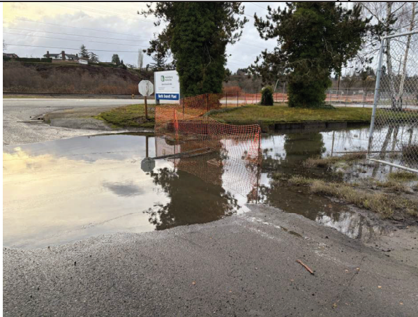
Photo 1: North Truck Bay flooding
