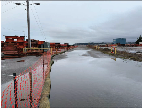
Photo 11: Current drive aisle on south end
