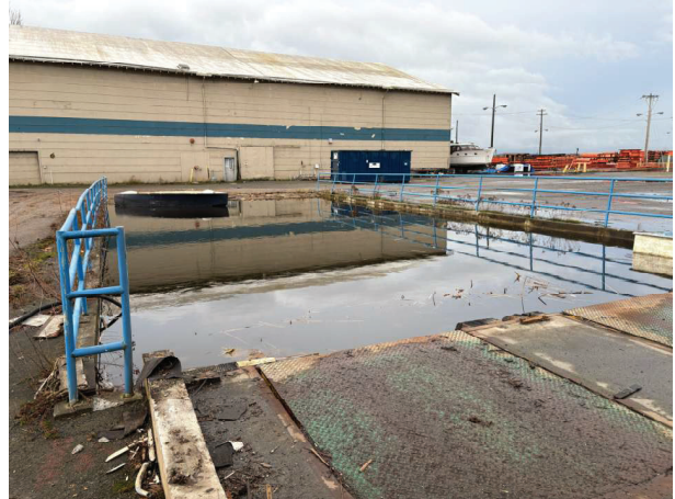
Photo 8: South Truck Bay
