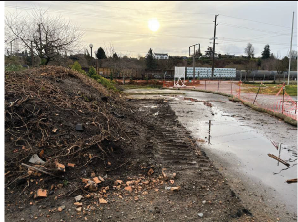
Photo 10: Stockpile at office building
