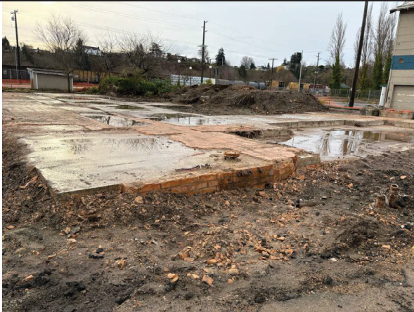
Photo 9: Office building pad
