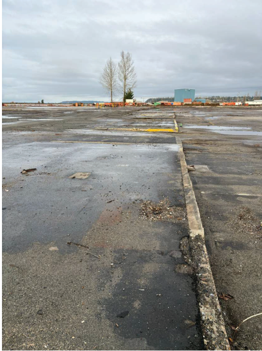
Photo 7: Curb/ramps across whole pad
