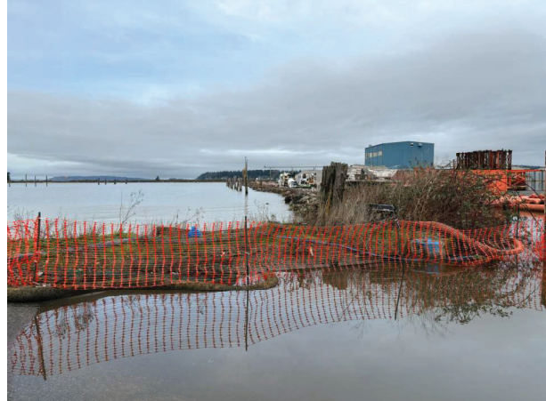
Photo 14: Flooding at OF-5, water level even with tide
