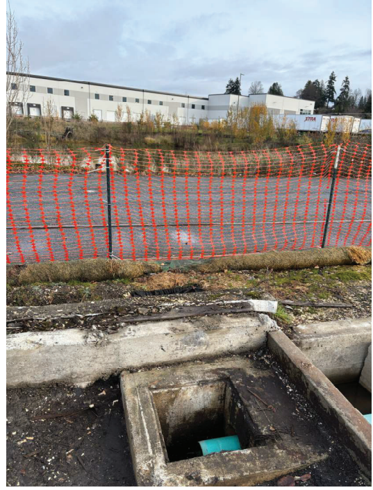
Photo 20: Catch basin (DS-7) to OF-2
