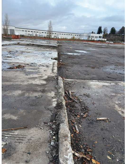
Photo 16: Curb running north-south
