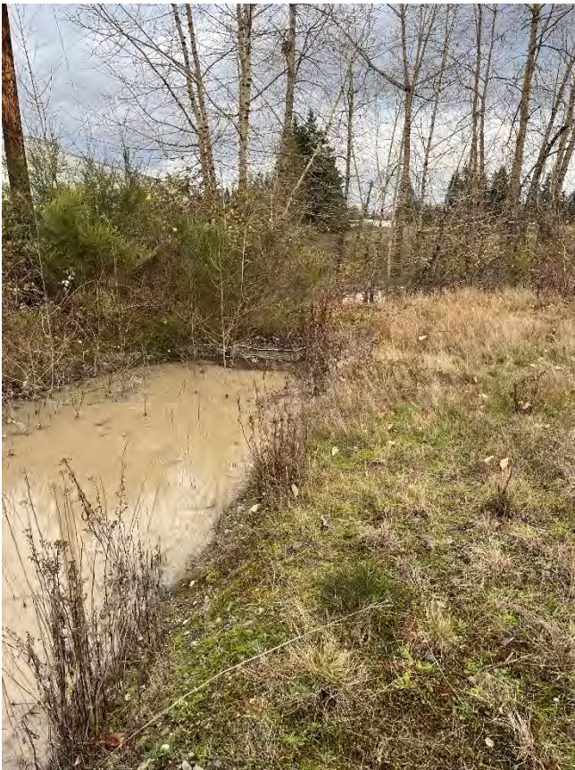
Photo point 1 Looking north at smaller cell of infiltration basin.
