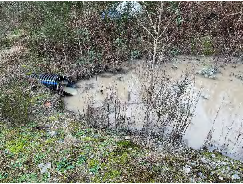
Photo point 1 Looking west at stormwater outfall into smaller cell of infiltration basin.
