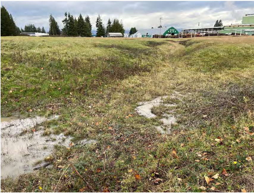
Photo point 4 Looking northeast and up "v"-shaped drainage ditch.
