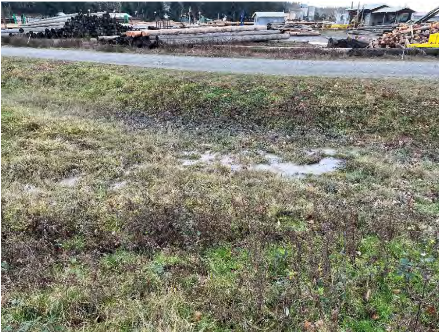
Photo point 3 Looking southeast showing NE extent of stormwater infiltration.
