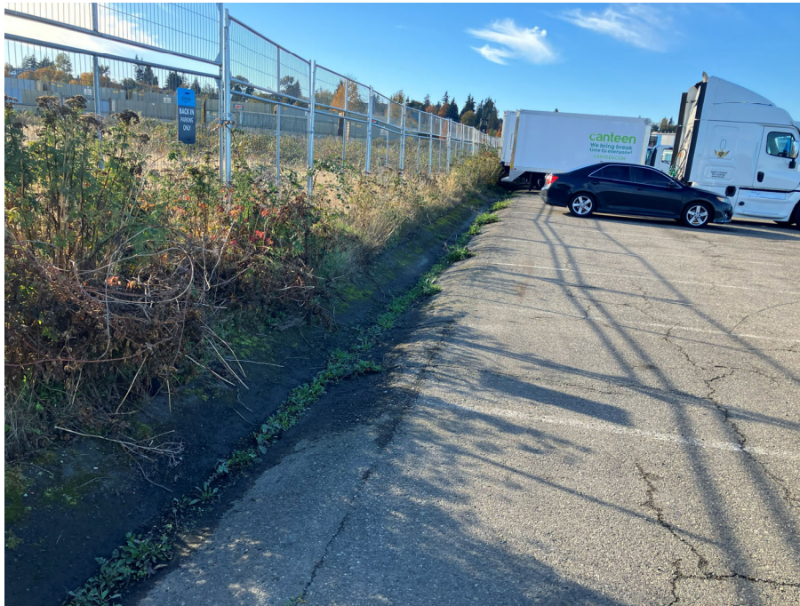
Photograph 5 – Looking west at the southern portion of the asphalt cap. Photograph shows vegetation in the south drainage ditch. Vegetation was observed to be growing through minor cracks and over the asphalt cap from the adjoining soil cap area.
