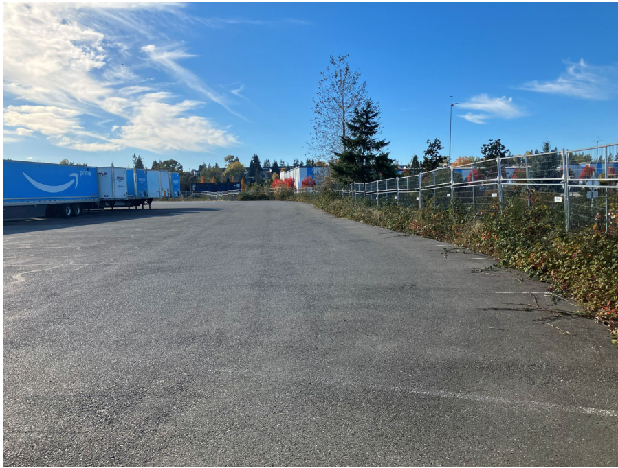
Photograph 7 - Looking west at the northern portion of the asphalt cap. Photograph shows vegetation growing over the asphalt cap surface from the northern landscaped area.
