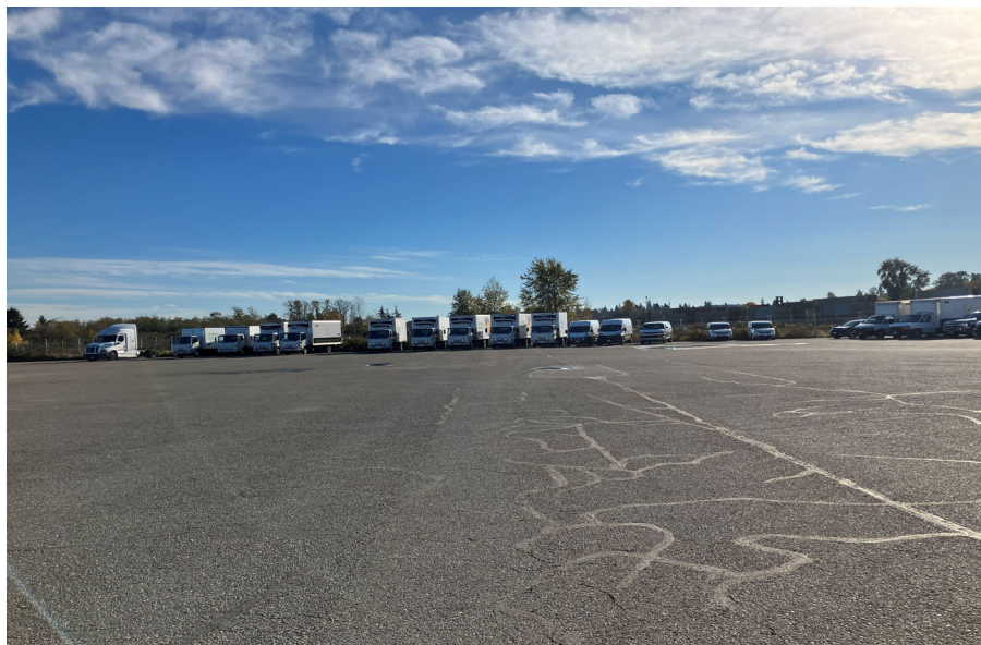
Photograph 4 – Looking south at the southern portion of the asphalt cap. Photograph shows repaired cracks and minoring ponding on asphalt cap surface.
