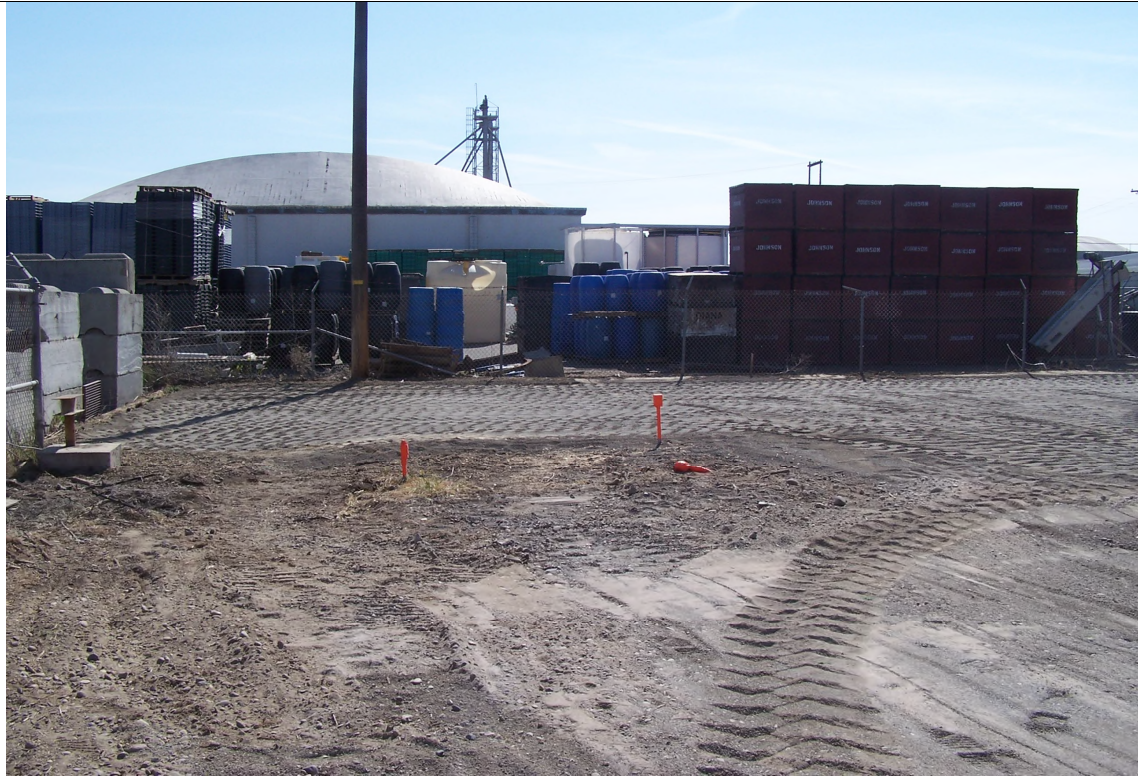
Grading of final surface.
