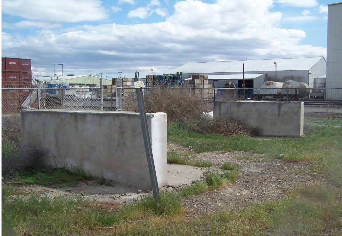
Concrete tank saddles and debris removed during closure activities.
