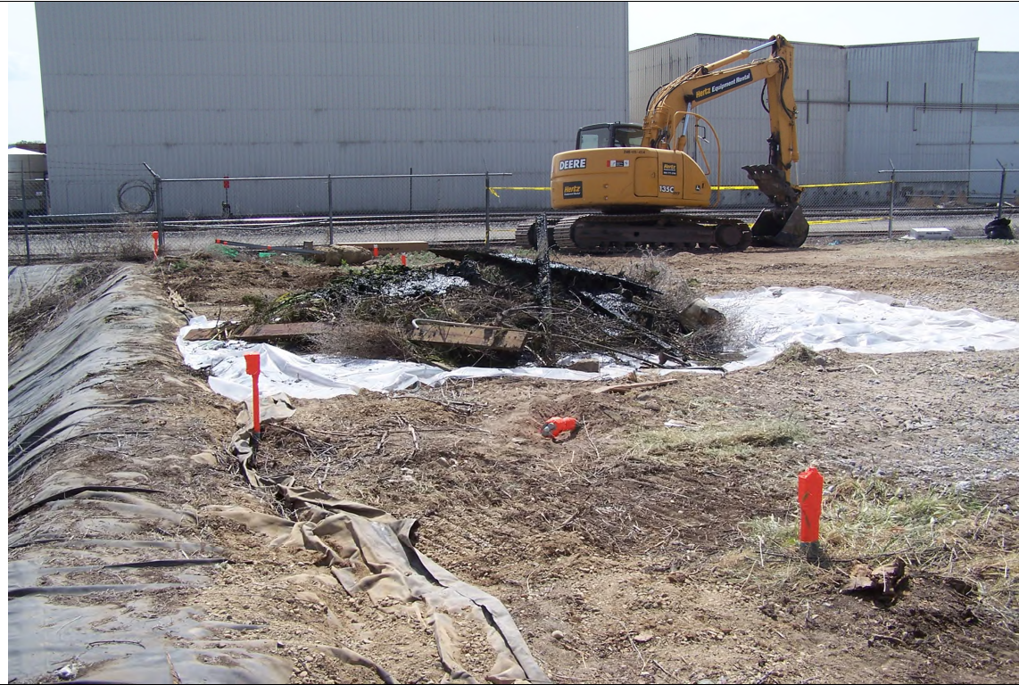
Debris removal from lagoon.
