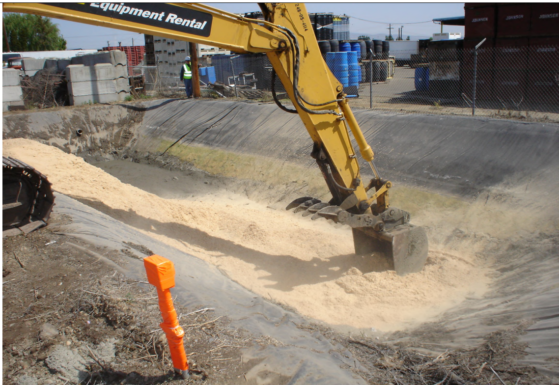
Addition of sawdust to stabilize remaining lagoon material.
