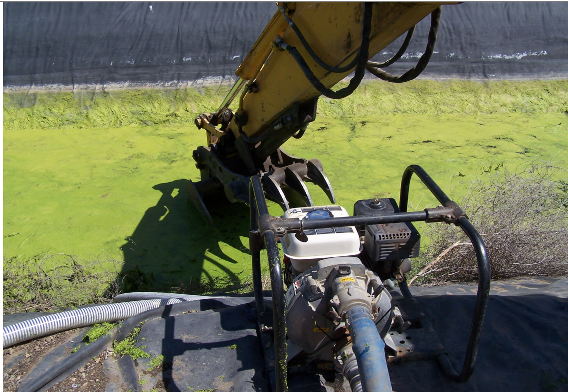
Removal of lagoon material and water.
