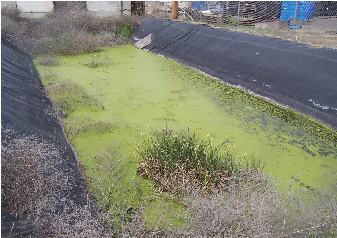
Lagoon prior to closure activities.
