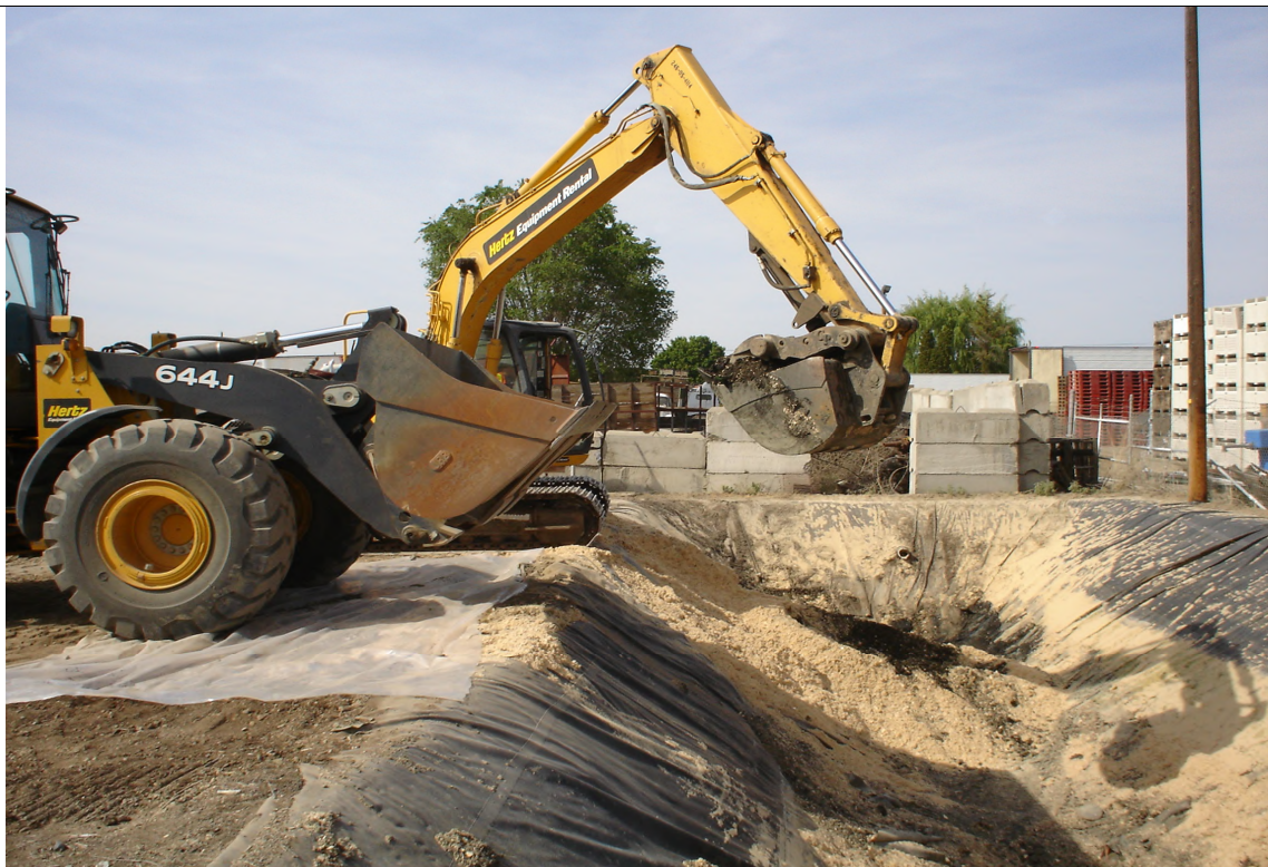
Stabilization and removal of lagoon material.
