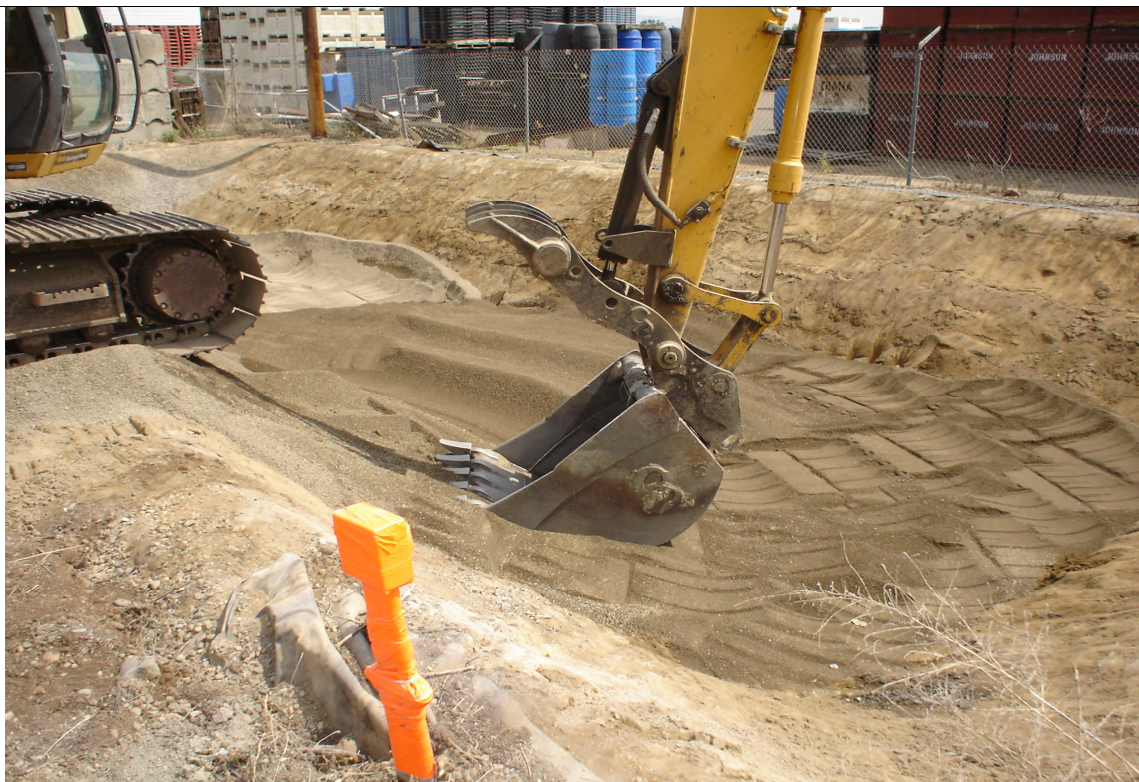
Backfill and compaction.
