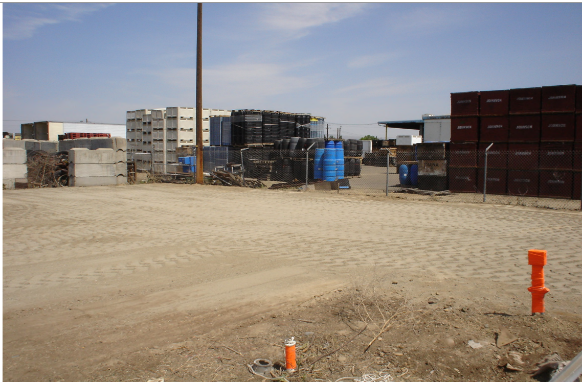
Completed lagoon closure.
