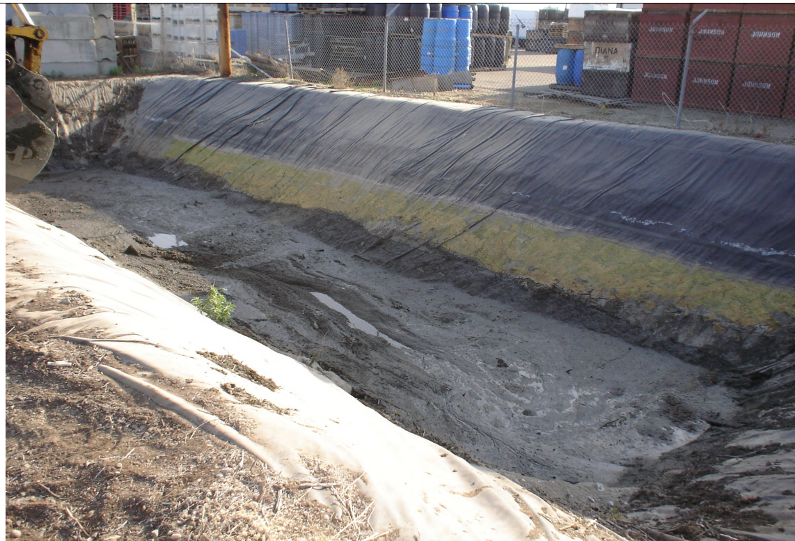
Lagoon after water and debris removal.
