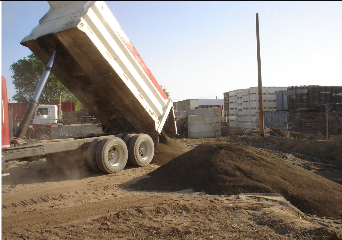
Dumping of fill material.
