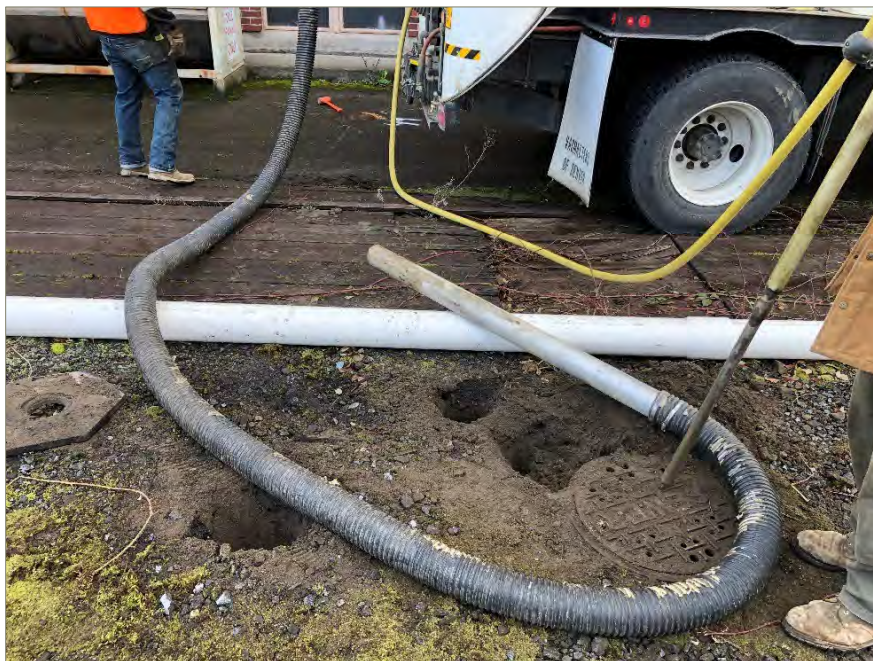
Exhibit C-10: Photo of Pressurized Air Wand and Vacuum Hose Used for Boring SB-2021-042 (View Direction is South)
