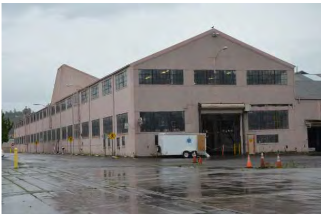
West end of Erection Shop (Hollowbore)
