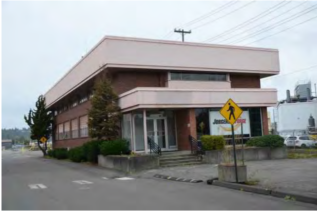
Office headquarters, view to the northwest.
