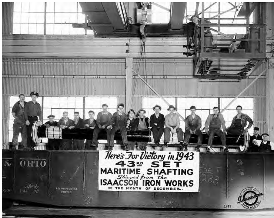
Figure 2-12. Workers at Issacson Iron Works in 1943 (University of Washington Libraries Digital Collections, IND0085).
