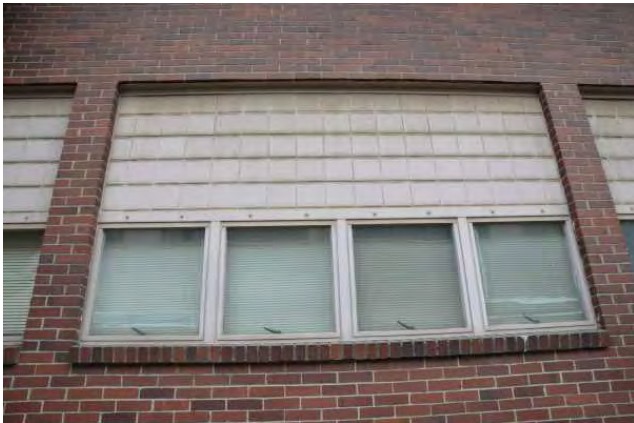
Window opening on south side of building, showing extent of infill, view to the north.
