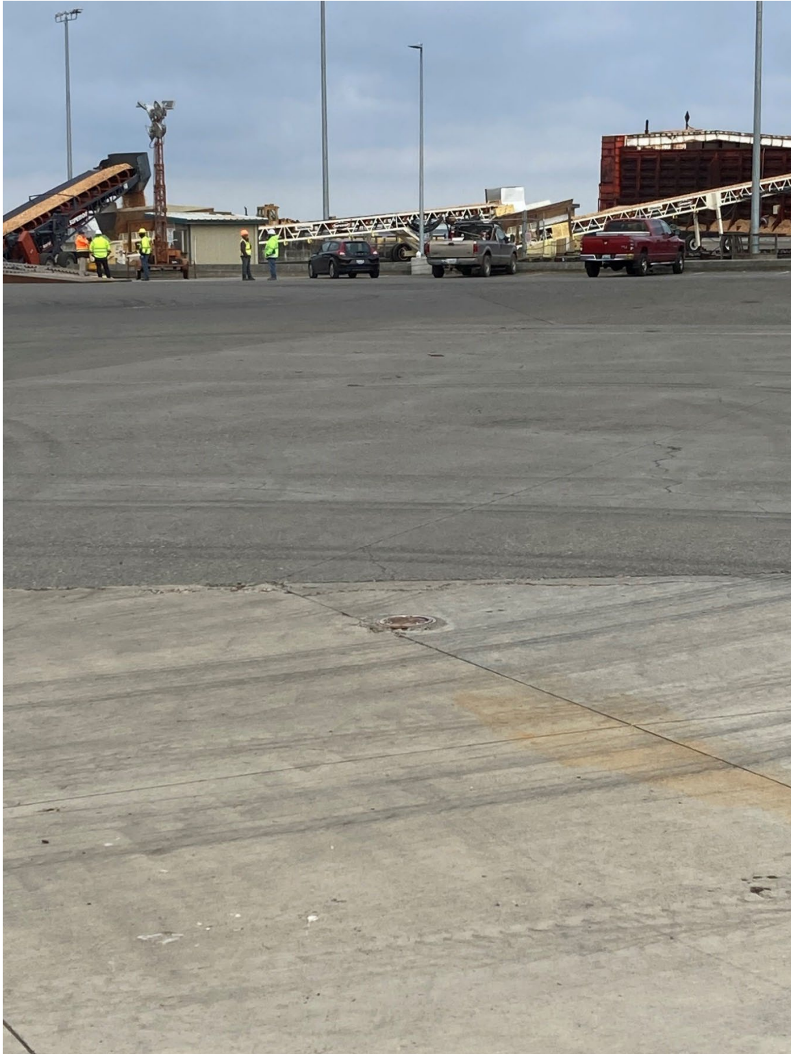
Photo 5: Flush-mounted well PP-37R in pavement located at the entrance to Wash Pad.
