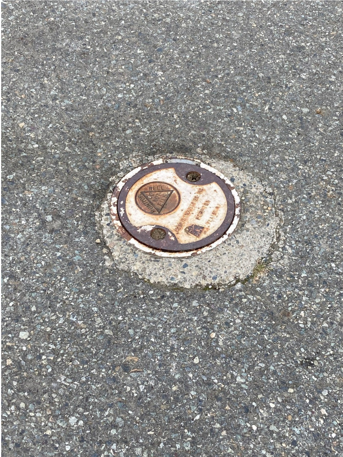
Photo 4: Flush mounted well PP-33.
