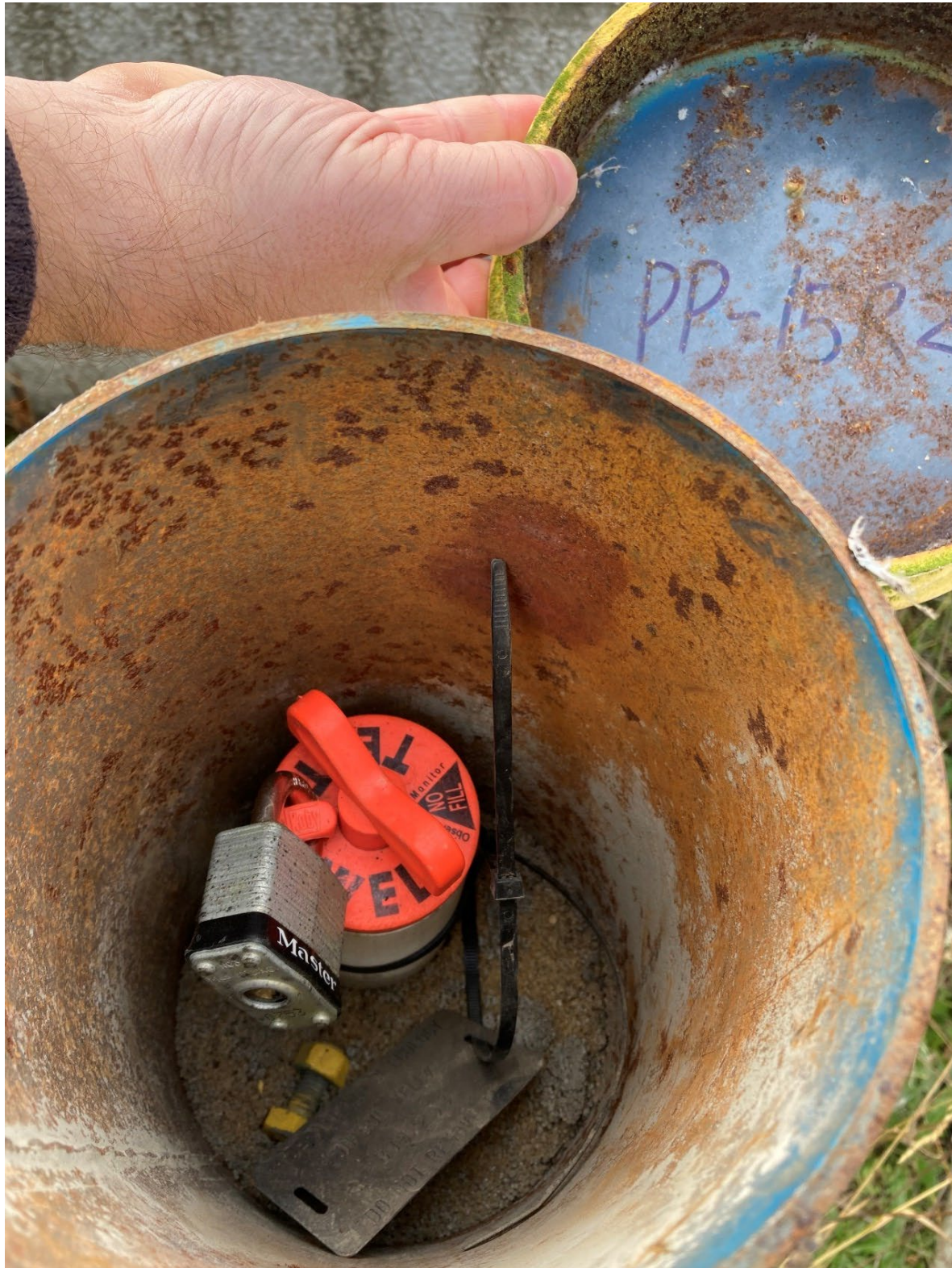
Photo 3: Photo of locked cap on monitoring well PP-15R2.
