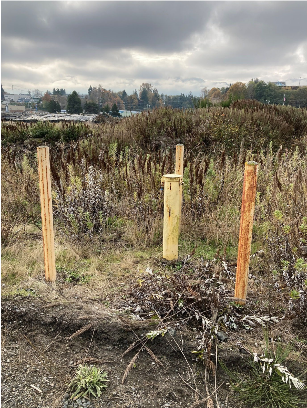
Photo 8: Metal bollards protecting well PP-21.
