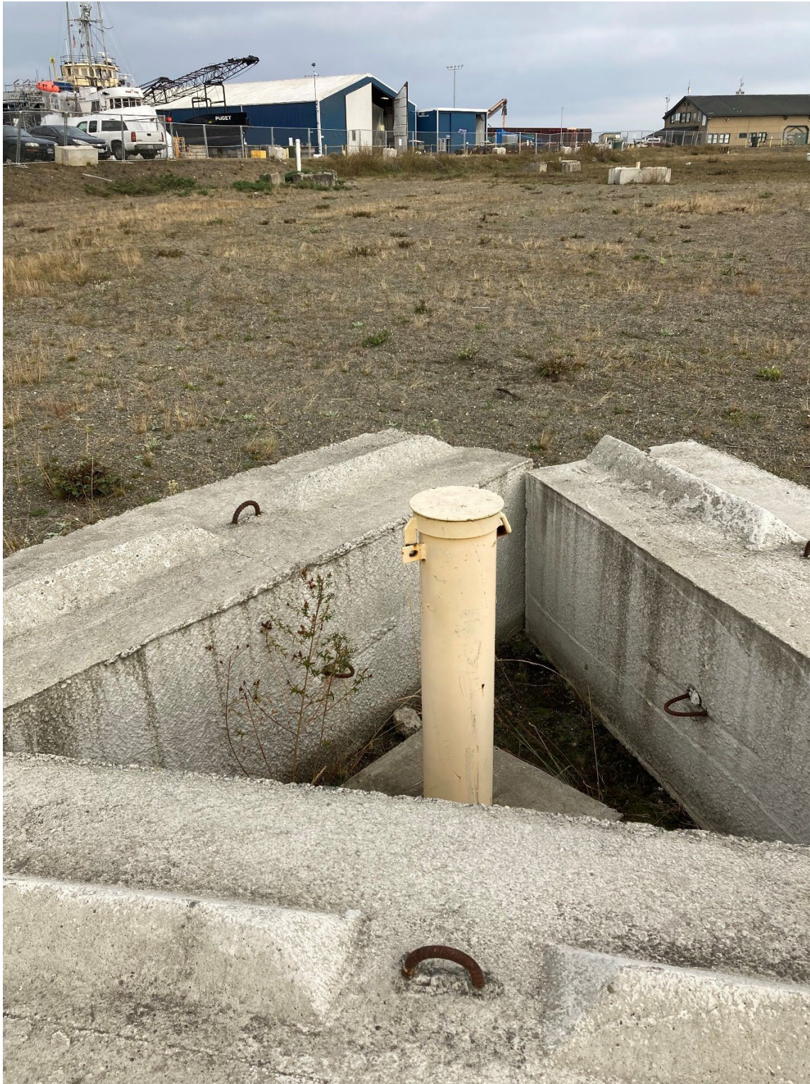
Photo 2: Typical well PP-27 completed aboveground surrounded by concrete blocks.
