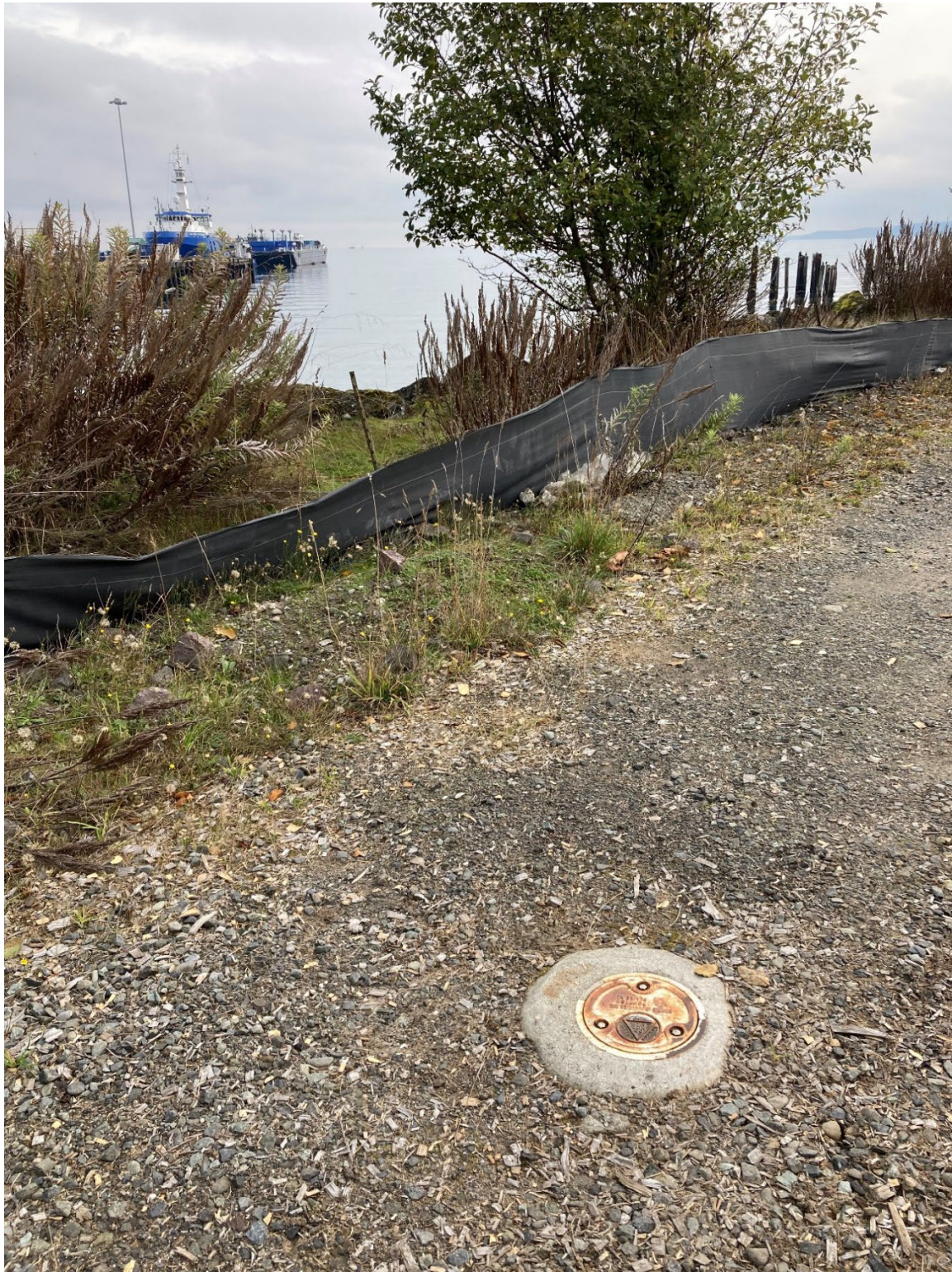
Photo 7: Flush-mounted well PP-18R2 in gravel north of Wash-Down Facility.
