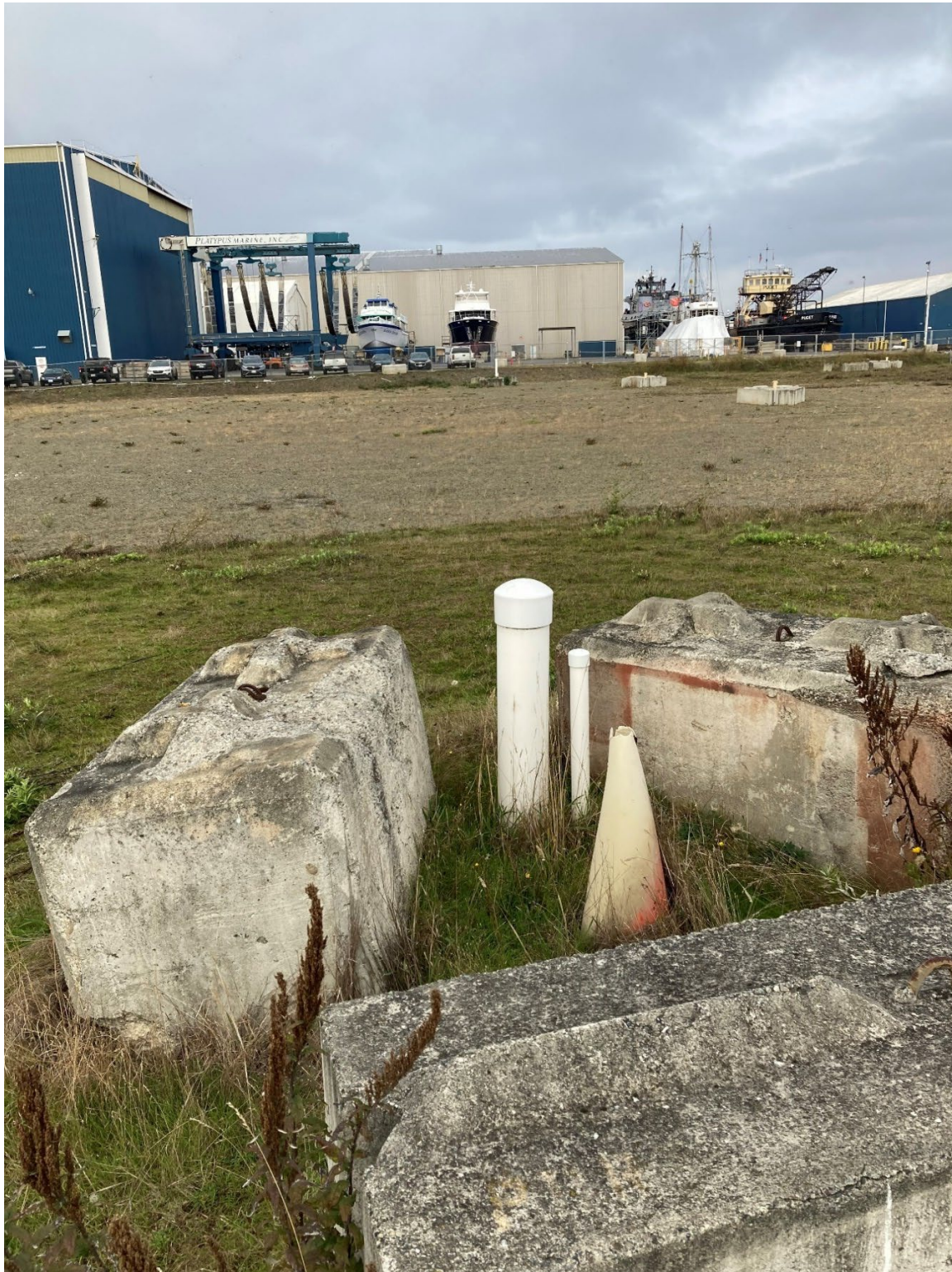
Photo 6: Infiltration Gallery #2 risers on either side of remediation area.
