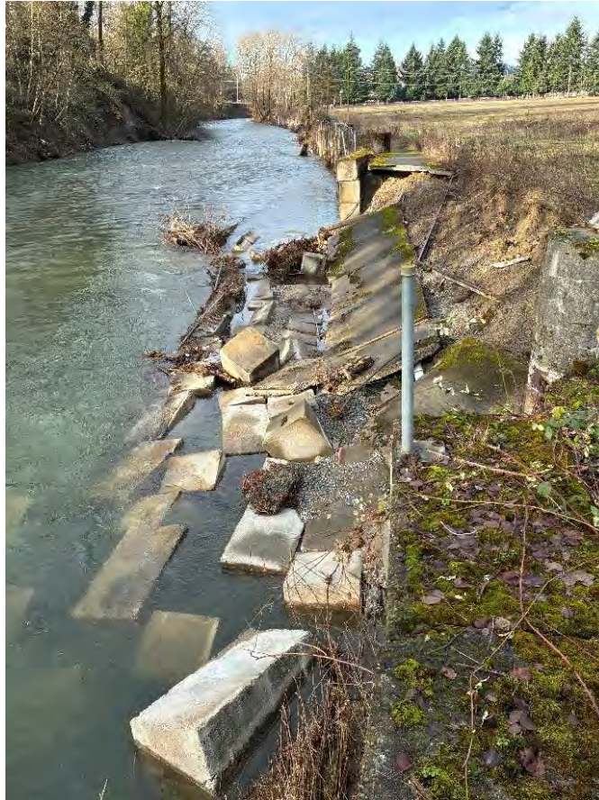
Pic 1. Preconstruction site conditions, looking west.
