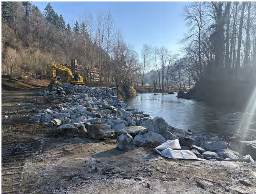
Pic 4. Final conditions of wall repair area.
