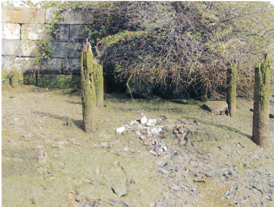
East End of Block Wall (view to north)
