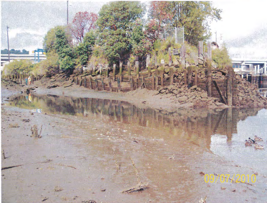
East End of North Bank (view to northwest)
