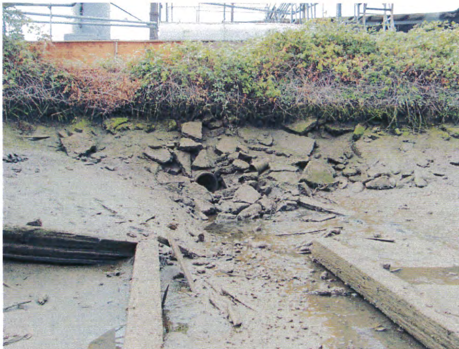
South Bank - 2nd Ave. Outfall (view to south)
