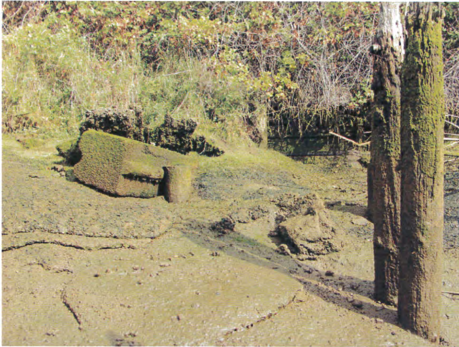
Conditions Near East End of Block Wall North Bank (view to northwest)
