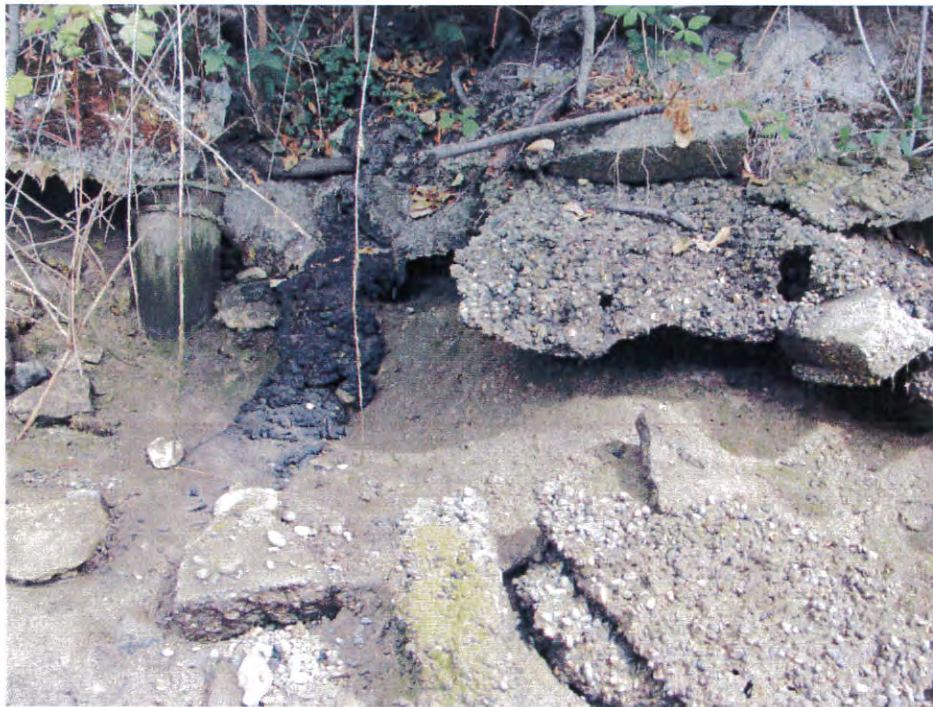
Asphalt-Like Material North Bank (view to north)
