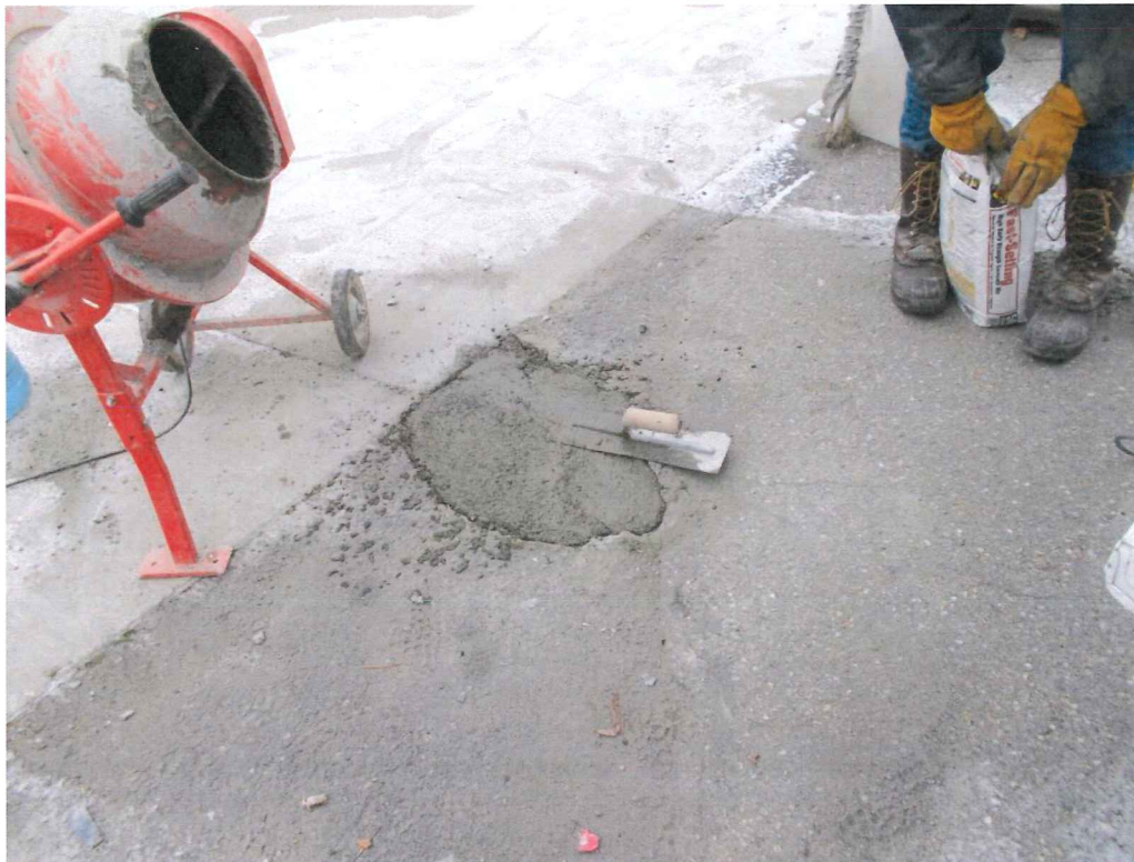
PHOTO NO. 2: Monitoring well MW-7, capped with concrete at surface.
