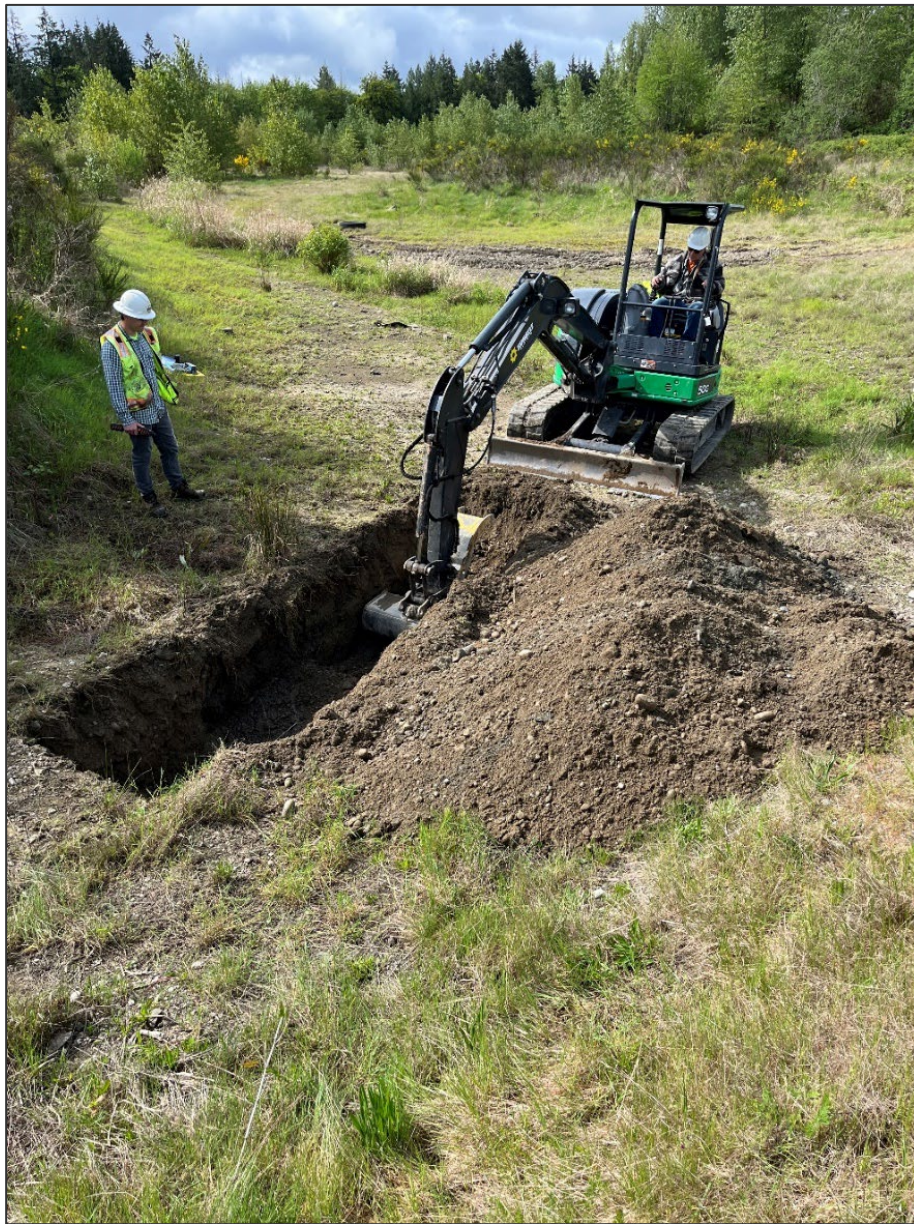
Figure 2: Test pit at the site during Phase 1 of the investigation.
