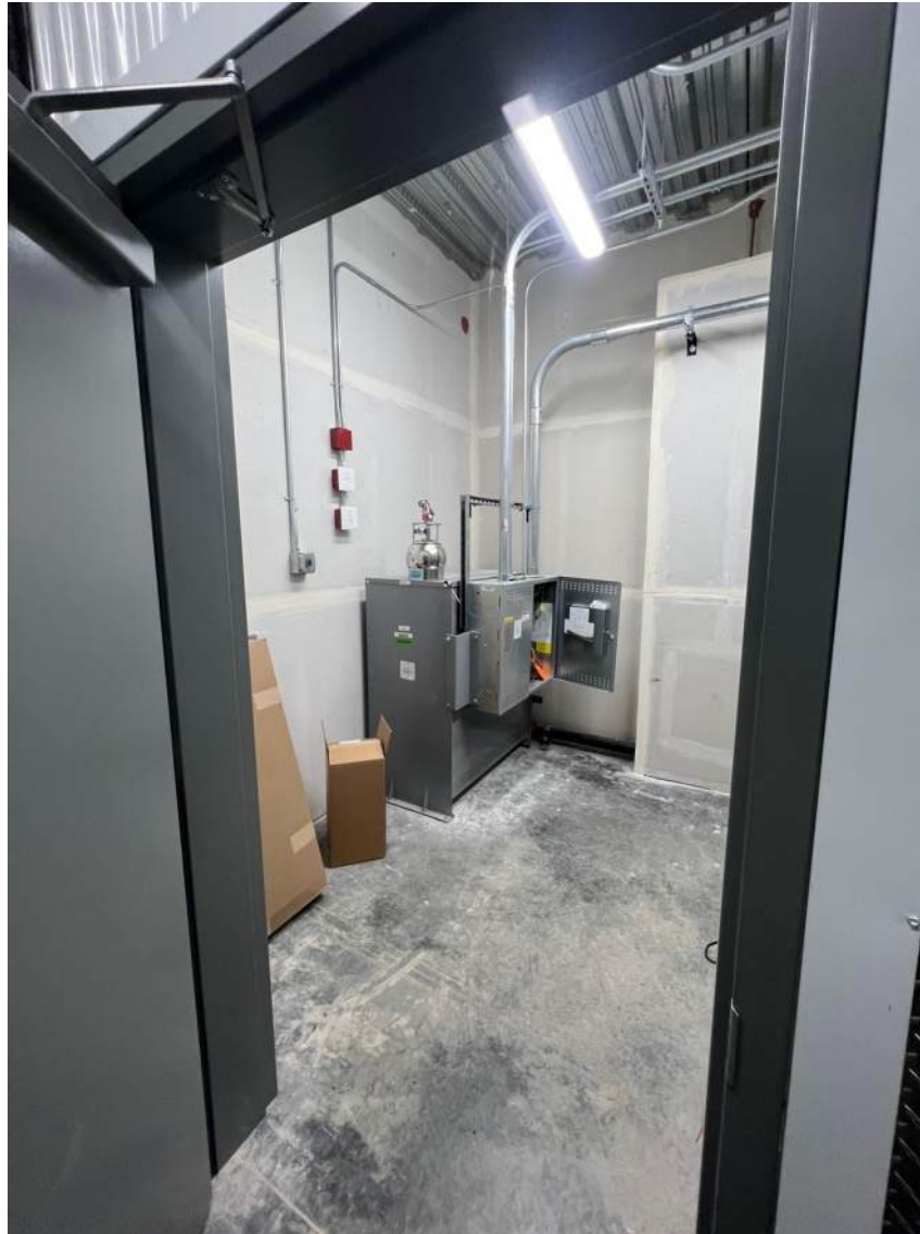
Indoor Air Sample Location 2 - Indoor2-060425 Mechanical Room
