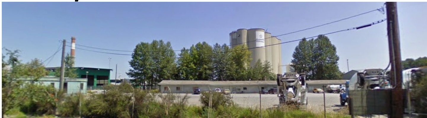
View of the site from W Marginal Way SW.
