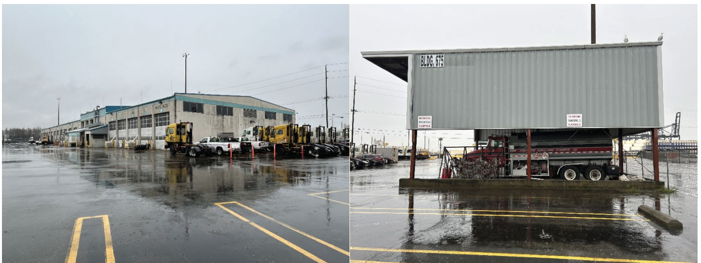
Figure 3. March 2026 photos of the Building 600 service garage (left) and fuel shed (right).
