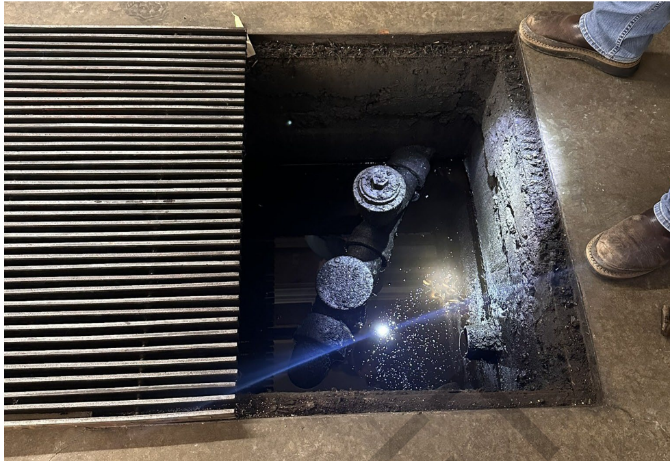
Photo 1. Interior of the oil/water separator containing approximately 8 inches of fluid and solids with petroleum-like odor and sheen.
